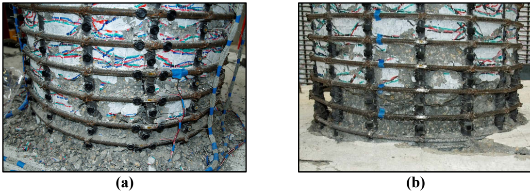
Figure 5.1: Existing plastic hinge (a) before and; (b) after crushed core removal
