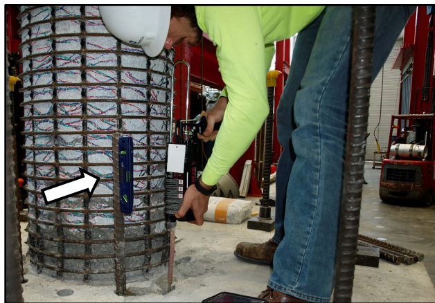
Figure 5.6: Installation of two-part epoxy into footing
