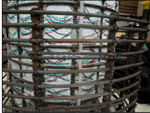
Figure 5.13: Completed rebar splice groove weld
