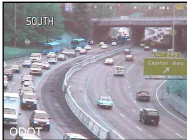
Figure 1-1. CCTV View of I-5 at Barbur Boulevard.
