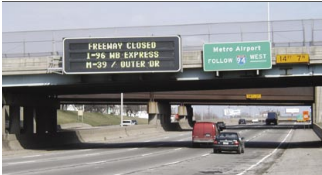
Figure 6-3. CMS informing drivers of a freeway closure
