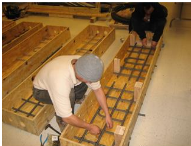
Figure 9. Photo. Fabrication of two bottom mats.
