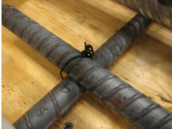
Figure 10. Photo. Close-up view of two crossing bars in the bottom mat.
