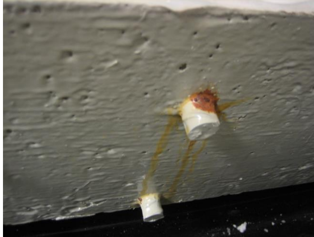
Figure 48. Photo. Rust oozing out of a top mat transverse bar.
