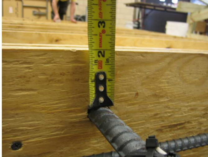
Figure 17. Photo. Top mat with 2-inch clear cover.
