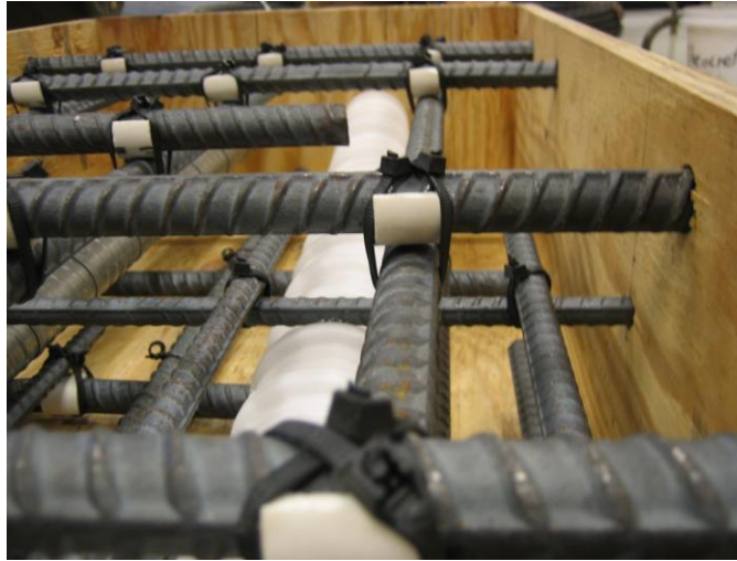
Figure 12. Photo. Close-up view of transverse and longitudinal bars in the top mat.
