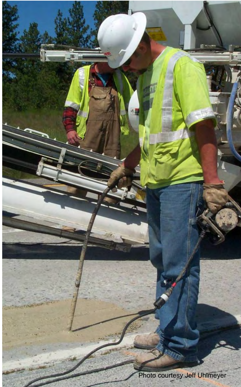
Figure A-68. Consolidating patching material.
