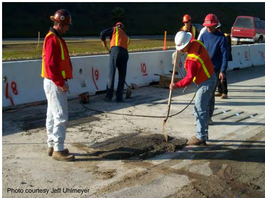
Figure A-65. Moving patching material into dowel bar slots.
