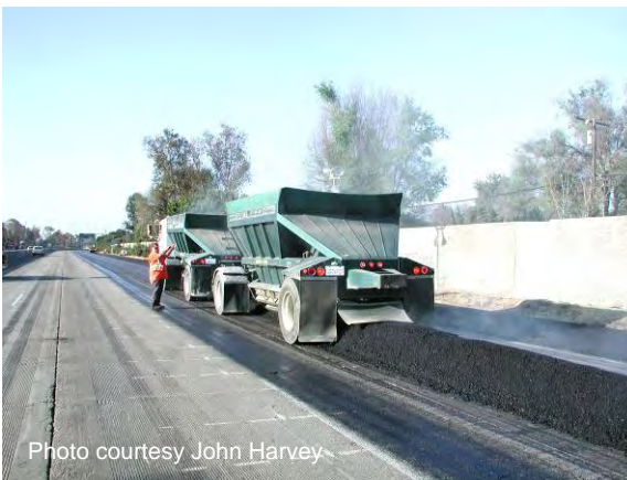
Figure 87 Delivery of HMA.
