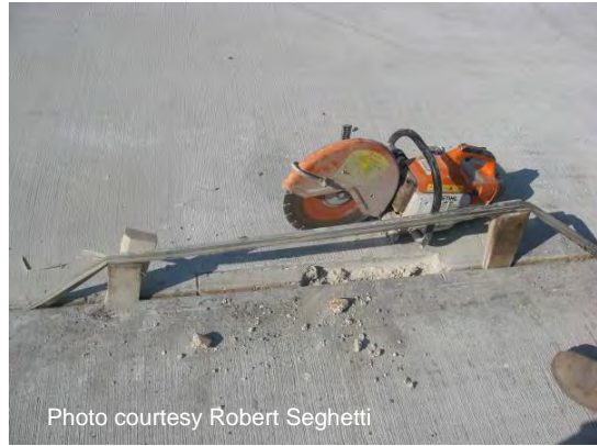
Figure 40 Sawcutting around spall.
