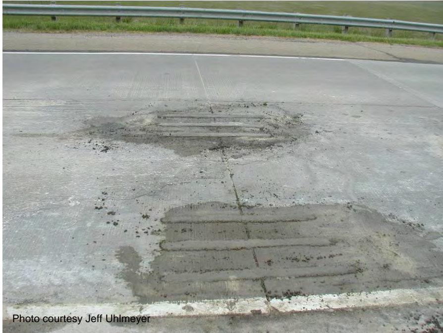
Figure A-73. Patching material should be left high to prevent overworking.
