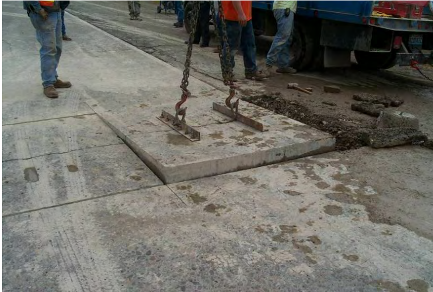
Figure 125 Removal of dowel bar retrofitted joint on I-90 test section.
