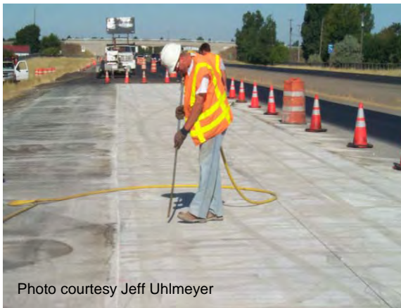
Figure 31 Cleaning joints.
