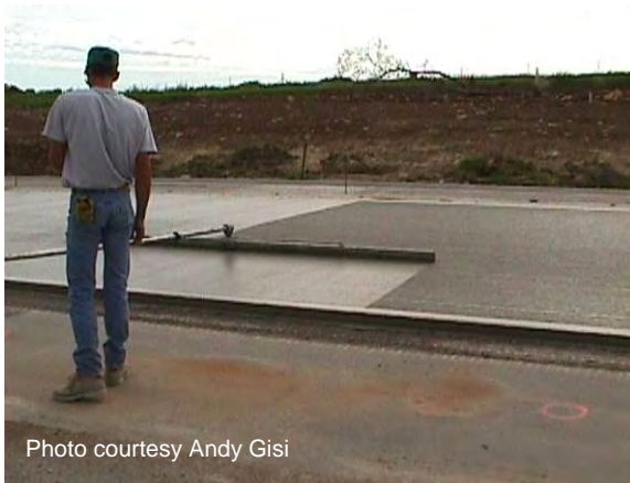
Figure 93 Tining bonded concrete overlay.
