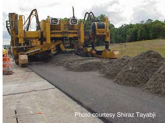
Figure 97 Placing concrete.
