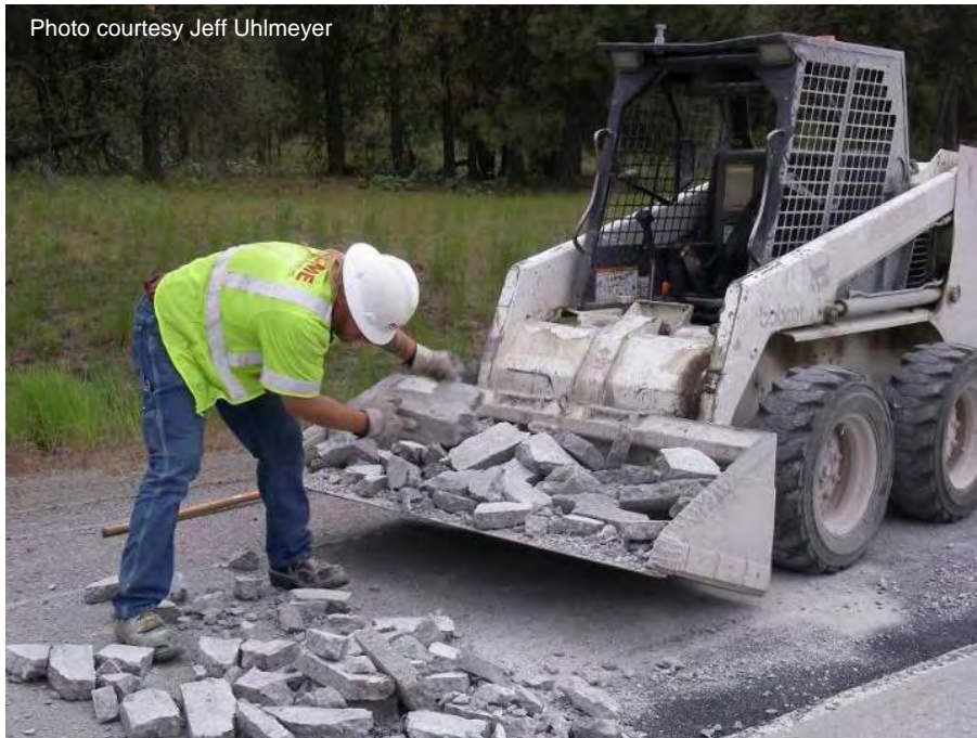
Figure A-34. Debris removal.
