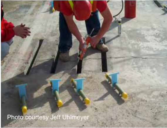
Figure 75 Applying silicone sealant.
