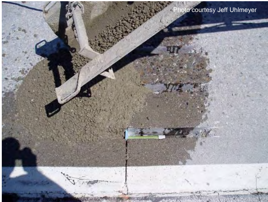
Figure A-64. Placing patching material.
