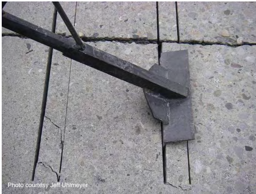
Figure A-28. Breaker bar.
