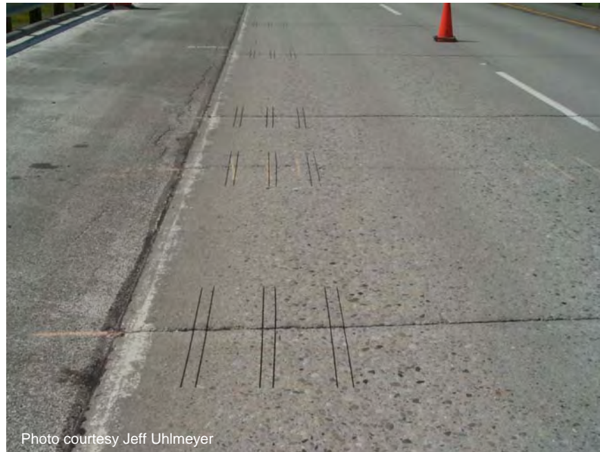
Figure A-13. Cut dowel bar slots on non-skewed transverse joint.
