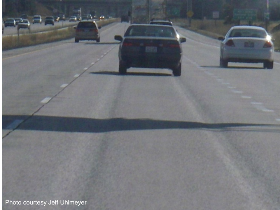
Figure 164 Studded tire wear on I-90, Spokane, Washington (2008).
