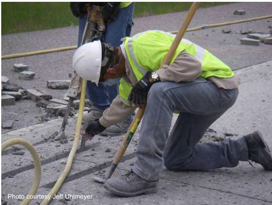
Figure A-17. Check depth of dowel bar slot.
