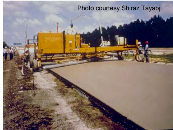
Figure 92 Placing bonded concrete overlay.
