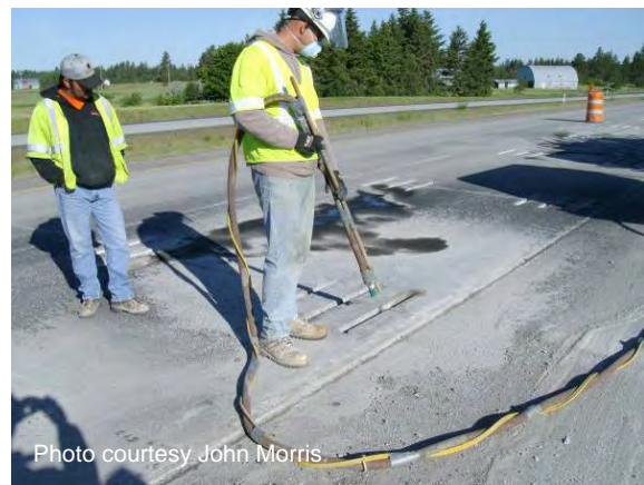
Figure 74 Cleaning dowel bar slots.
