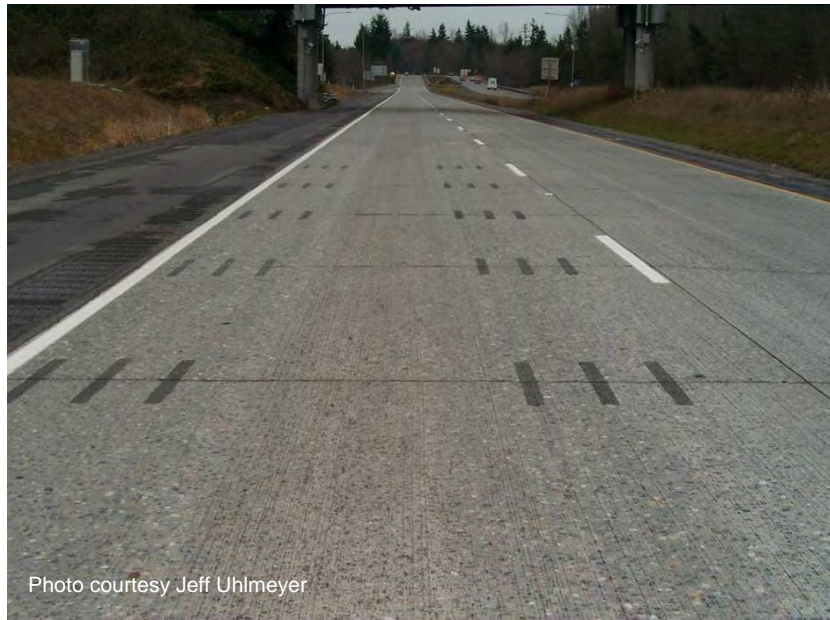
Figure A-84. Completed roadway.
