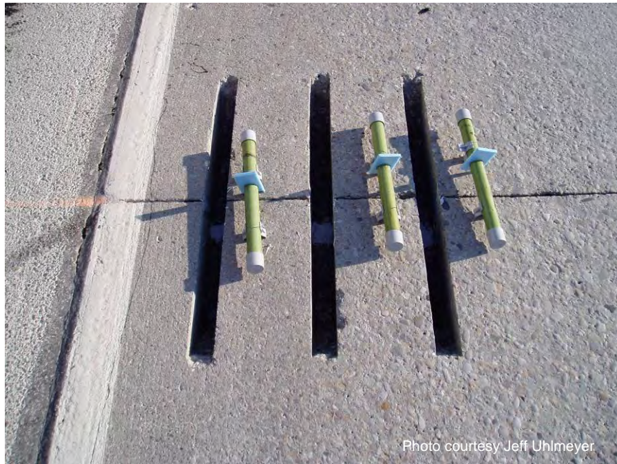
Figure A-54. Dowel bar retrofit assemblies.
