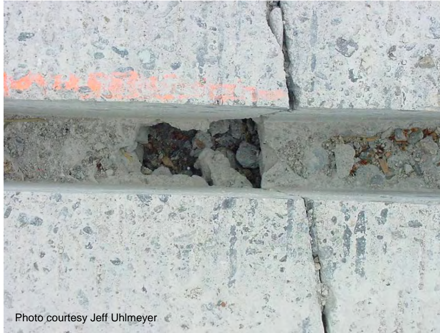
Figure A-31. Jackhammer punching through the bottom of the dowel bar slot.
