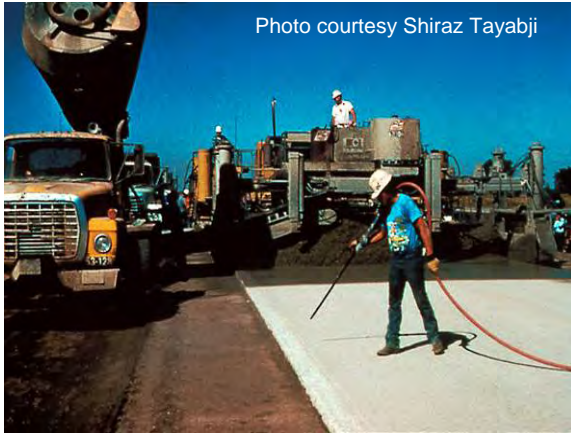
Figure 91 Final cleaning prior to paver.
