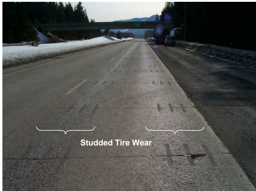
Figure A-79. Wear due to studded tires.
