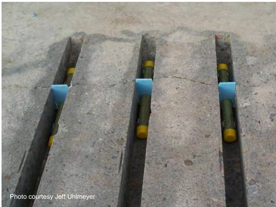
Figure A-57. Dowel bar retrofit assembly at a transverse crack.
