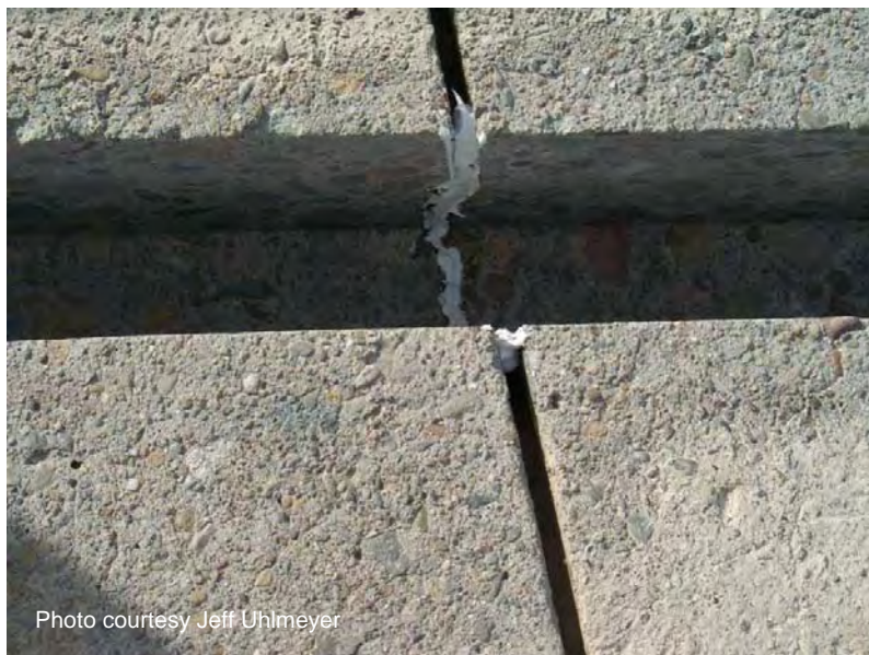
Figure A-51. Caulked dowel bar slot.
