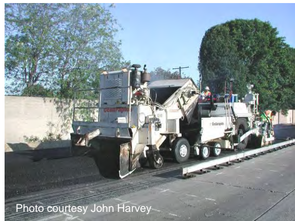
Figure 88 HMA pick up and paving.
