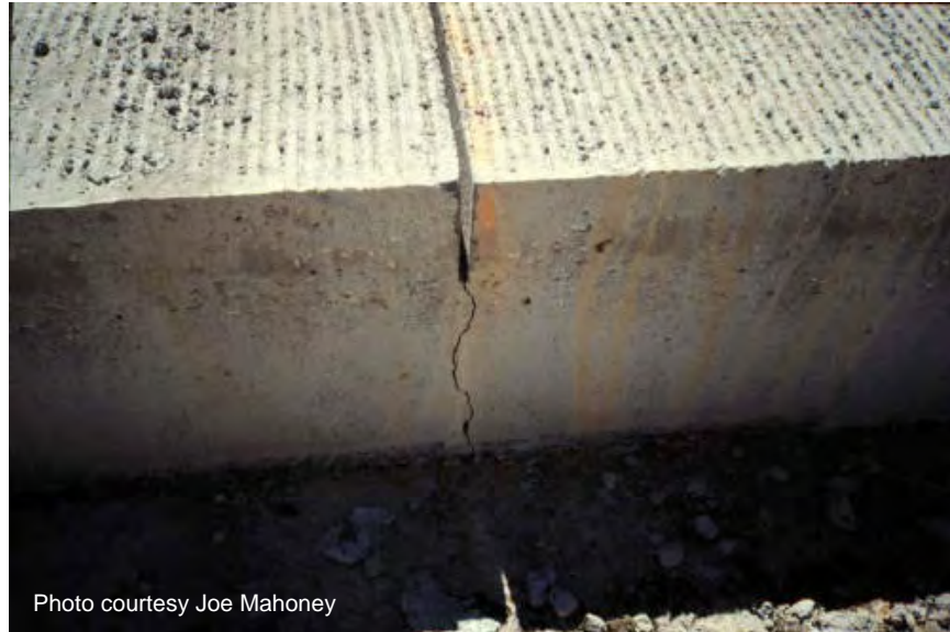
Figure 10 Aggregate interlock.
