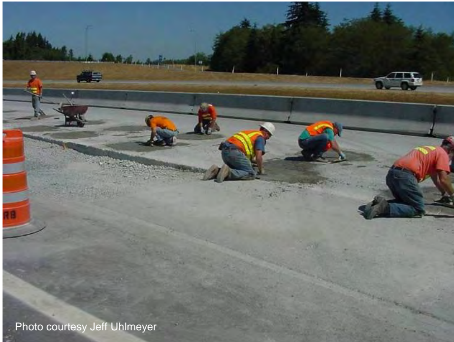
Figure A-72. Finishing patching material.
