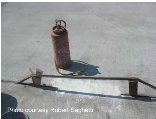
Figure 47 Applied curing compound.
