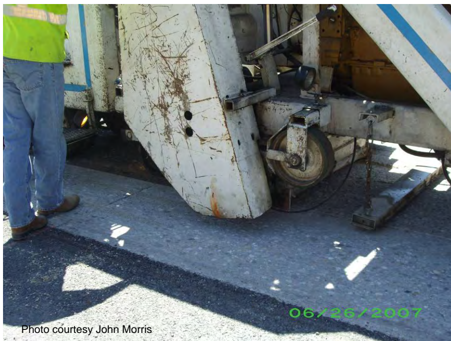
Figure A-83. Diamond grinding equipment.
