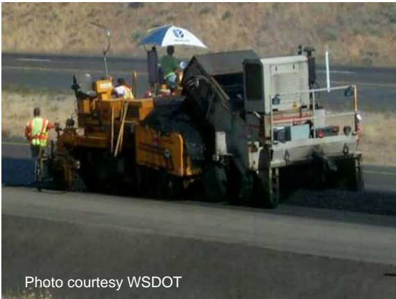
Figure 83 Placing HMA.
