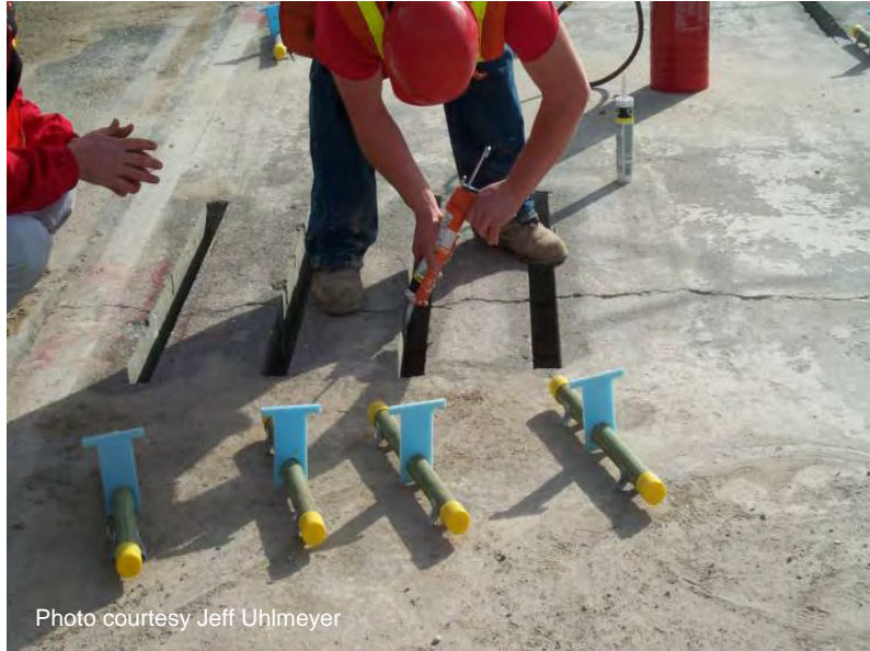
Figure A-50. Caulking dowel bar slot sides and bottom.
