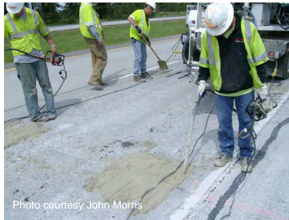
Figure 80 Consolidating patching material.
