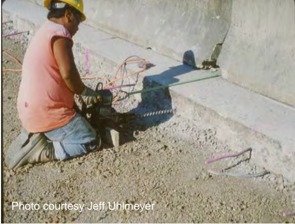
Figure 55 Drilling holes for tie bars.
