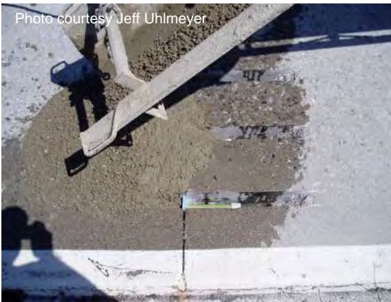
Figure 79 Placing patching material.
