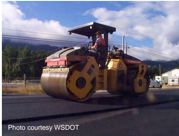
Figure 84 Compacting HMA.
