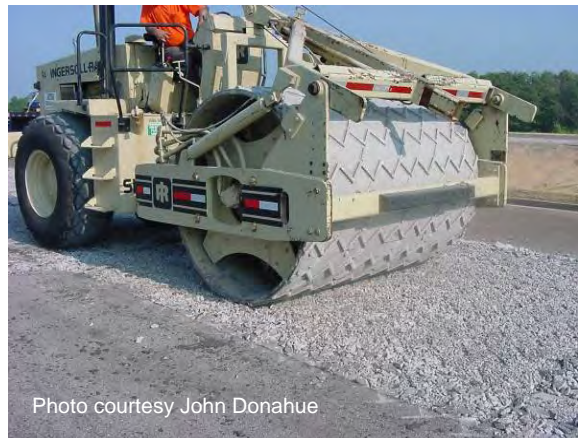
Figure 104 Rolling rubblized layer.
