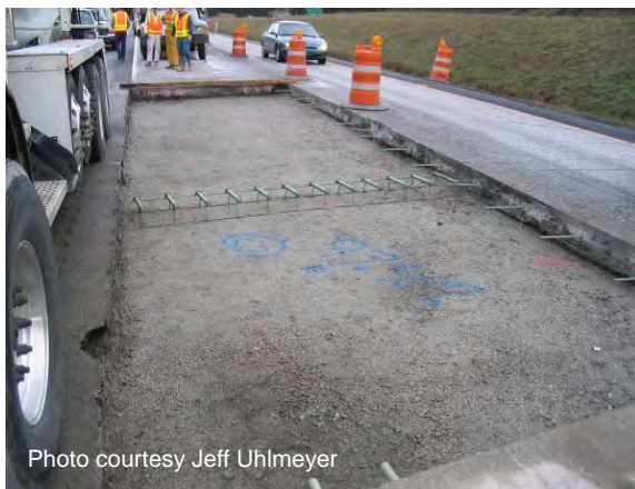
(a) Dowel bars in cages.
