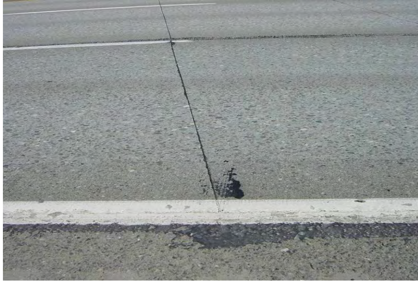
Figure 7 Contraction joint.
