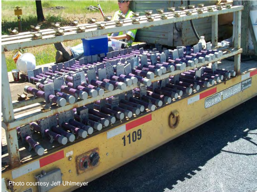
Figure A-52. Dowel bar retrofit assemblies.
