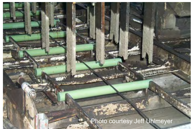
(b) Dowel bar inserter.
