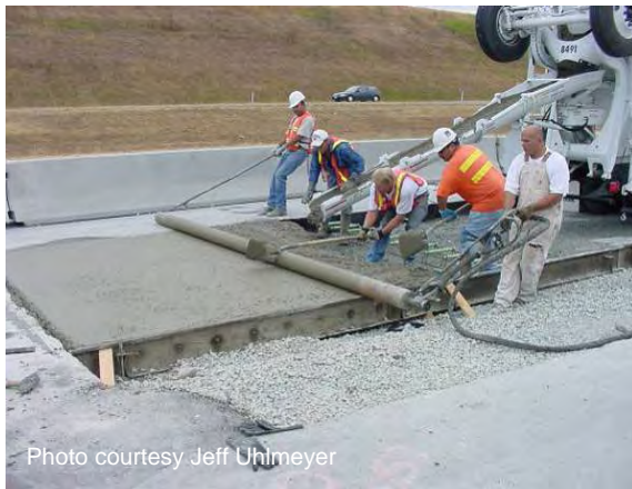
Figure 61 Final screed rolling.
