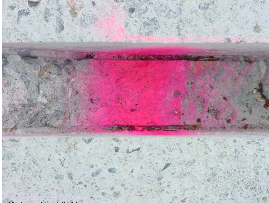
Figure A-29. Concrete not fully removed from the bottom of the dowel bar slot.
