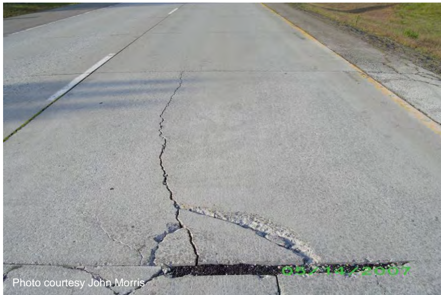
Figure 24 Multi-cracked panel.
