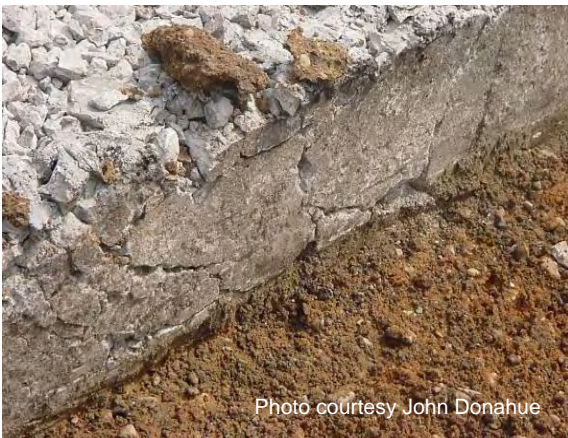
Figure 103 Rubblized concrete slab.
