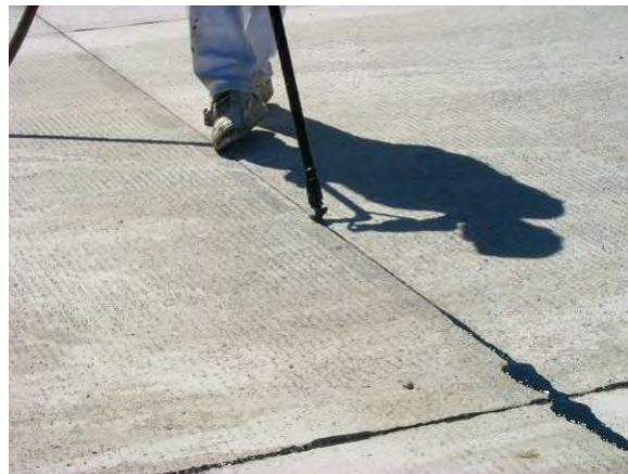
Figure 32 Sealing joints or cracks.
