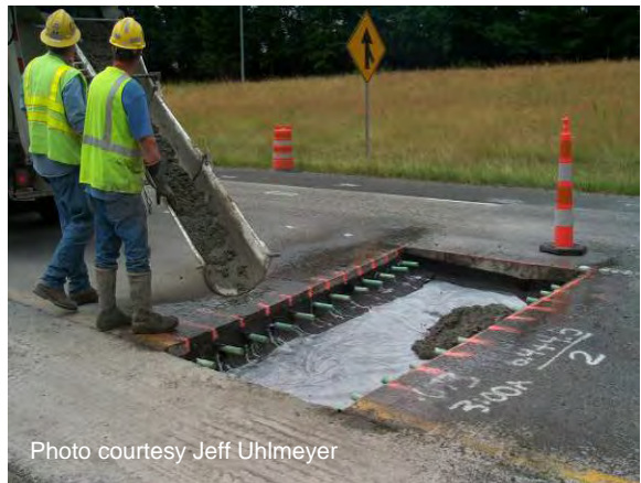
Figure 60 Placing concrete.
