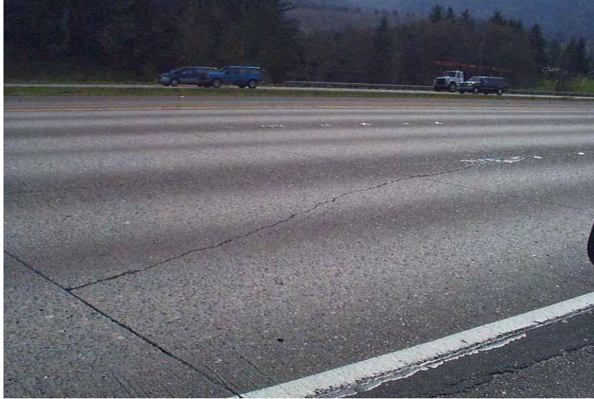
Figure 23 Longitudinal cracking.
