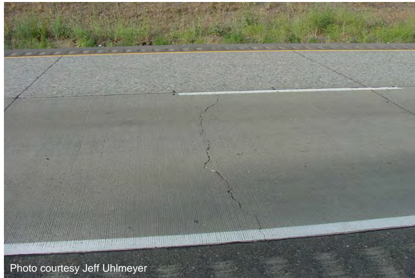
Figure 22 Transverse cracking.
