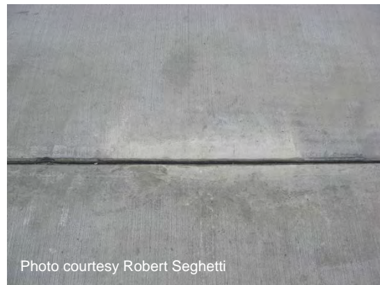
Figure 48 Final spall repair.
