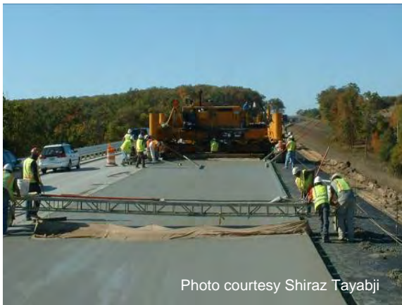
Figure 98 Finishing concrete.
