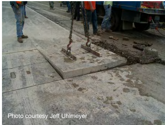
Figure 52 Concrete removal (lifting method).
