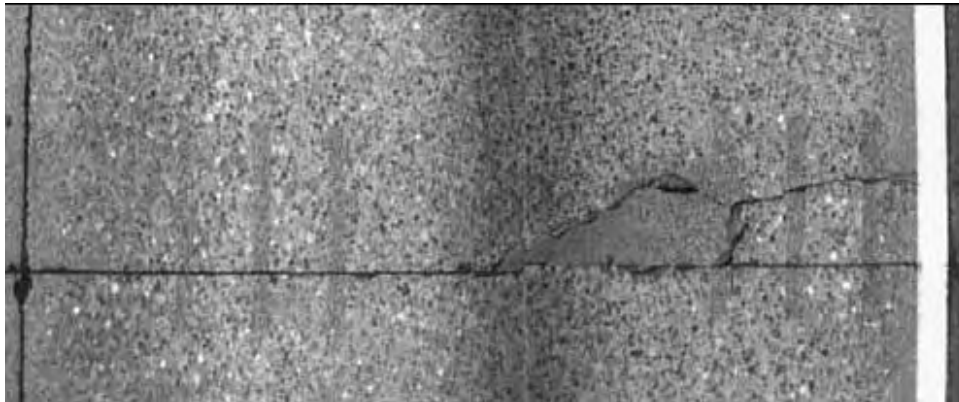
Figure E-19 Spall repair with dowel bar retrofit.
