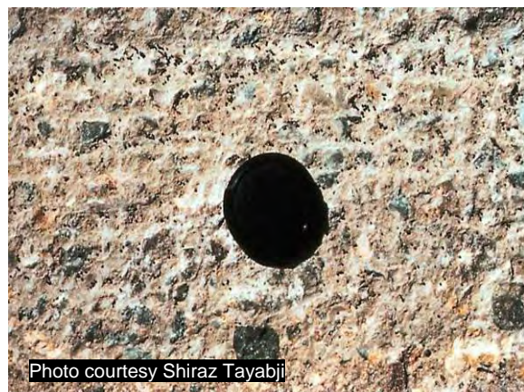
Figure 90 Shotblasted surface (close-up).
