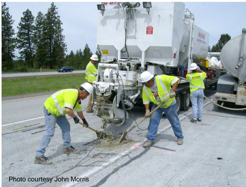
Figure A-63. Placing patching material.
