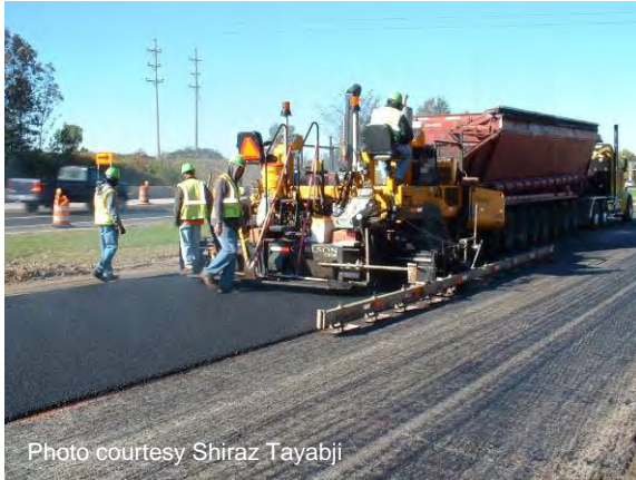
Figure 96 Placing HMA separator layer.
