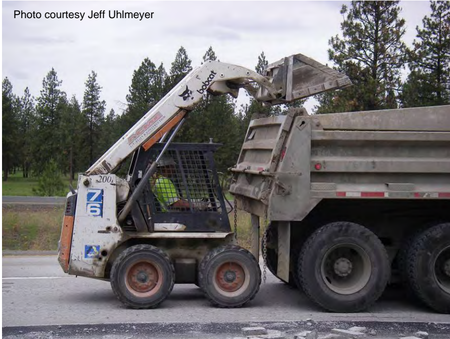
Figure A-35. Debris removal.
