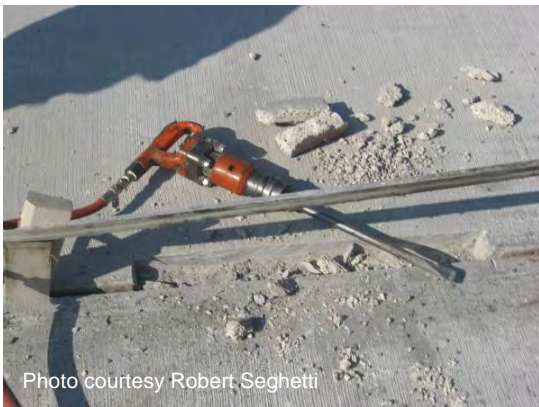
Figure 41 Removing concrete.
