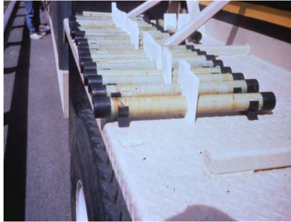
Figure 76. Dowel bar retrofit assembly.
