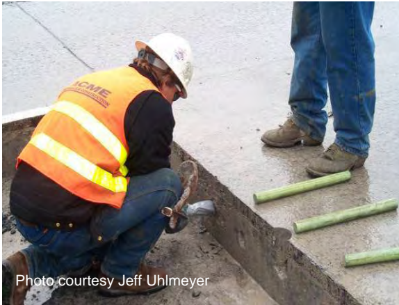
Figure 57 Inserting epoxy into dowel hole.
