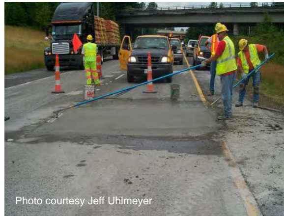
Figure 62 Finishing concrete.
