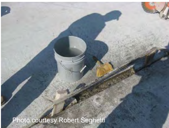
Figure 43 Applying bonding agent.
