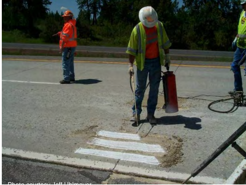
Figure A-75. Applying curing compound.
