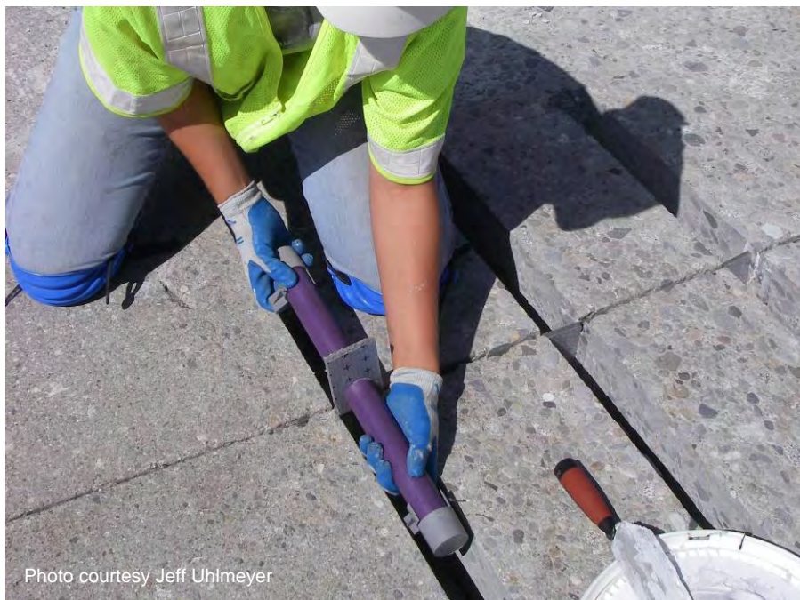
Figure A-55. Inserting dowel bar retrofit assemblies into dowel bar slots.
