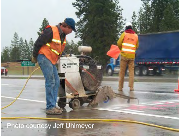
Figure 49 Sawcutting.
