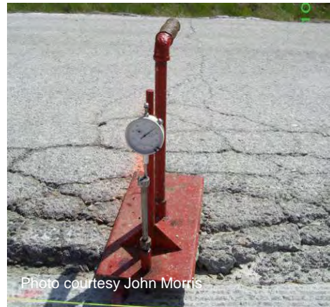
Figure 38 Measuring slab lift.
