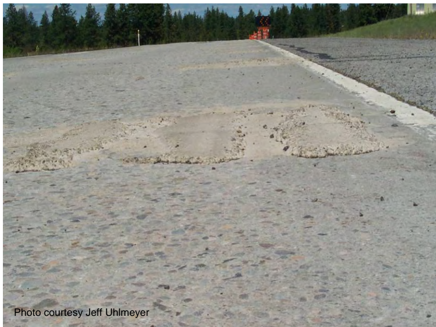
Figure A-74. Patching material left high to minimize segregation.
