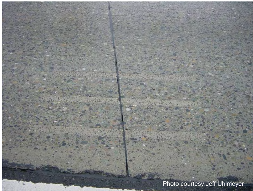
Figure A-85. Close-up of completed dowel bar retrofit.
