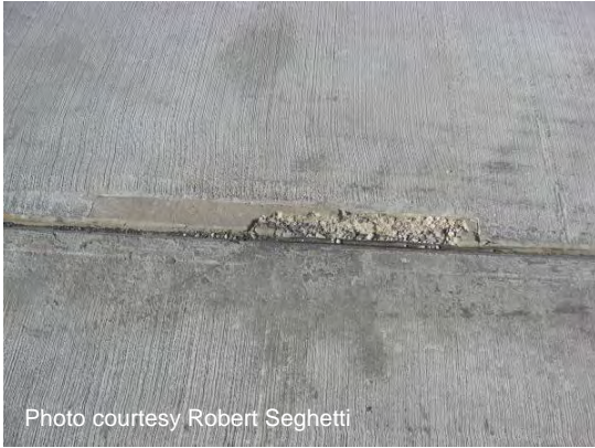
Figure 39 Spall to be repaired.
