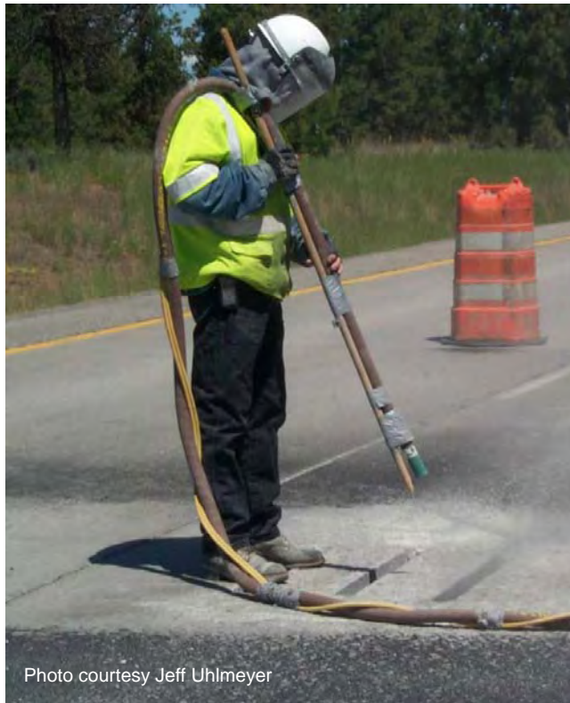
Figure A-37. Cleaning dowel bar slot by shot blasting.
