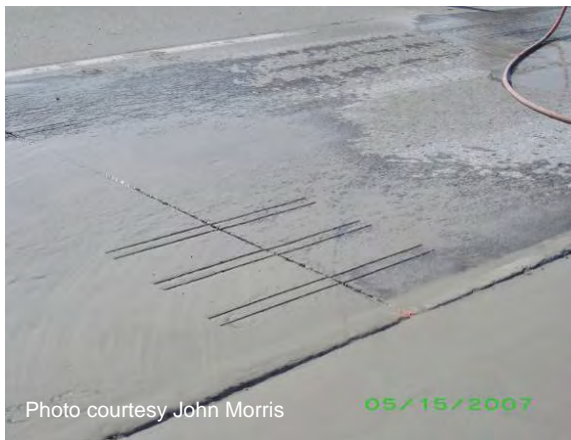
Figure 71 Cut dowel bar slots.
