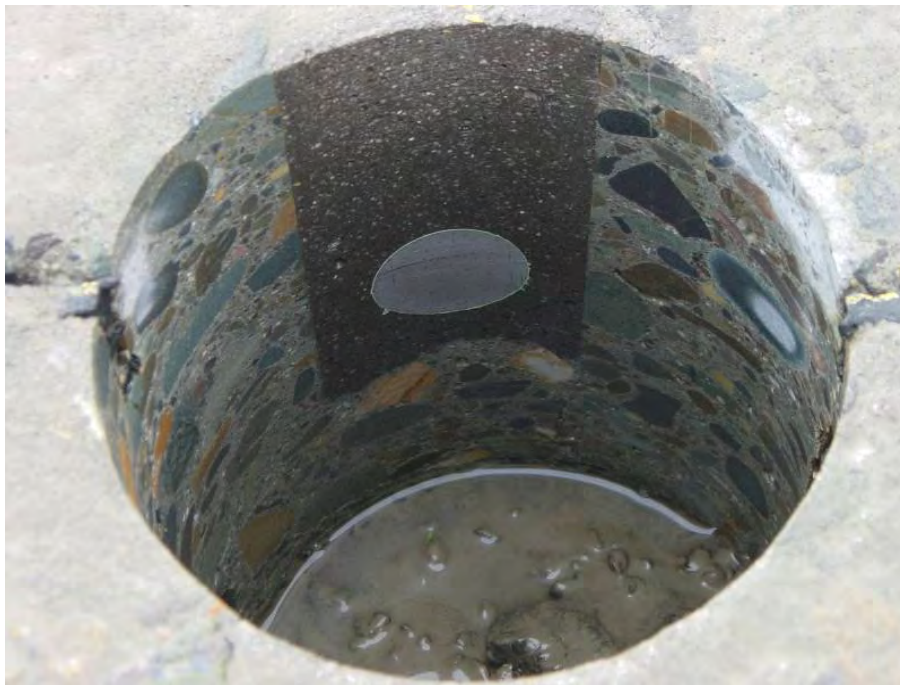
Figure 212 Good consolidation of patching material in dowel bar retrofit slot.
