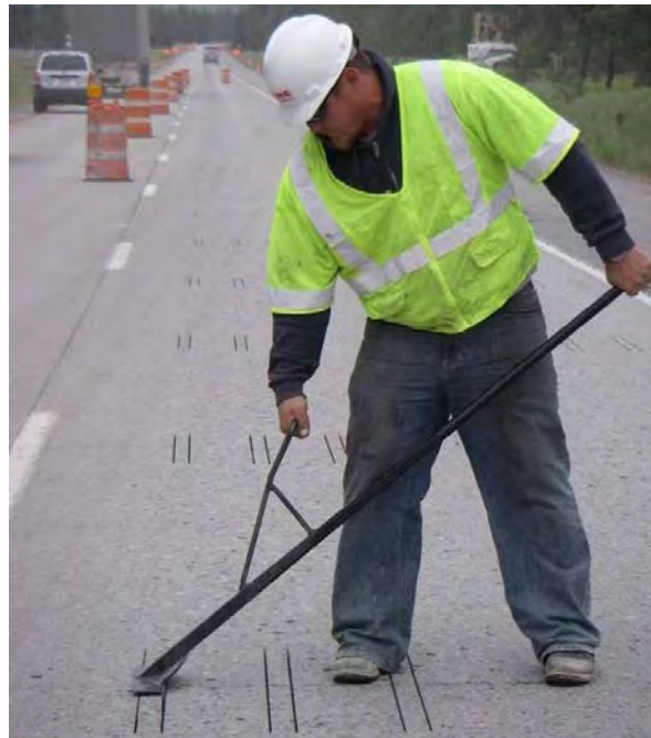
Figure A-27. Breaker bar.
