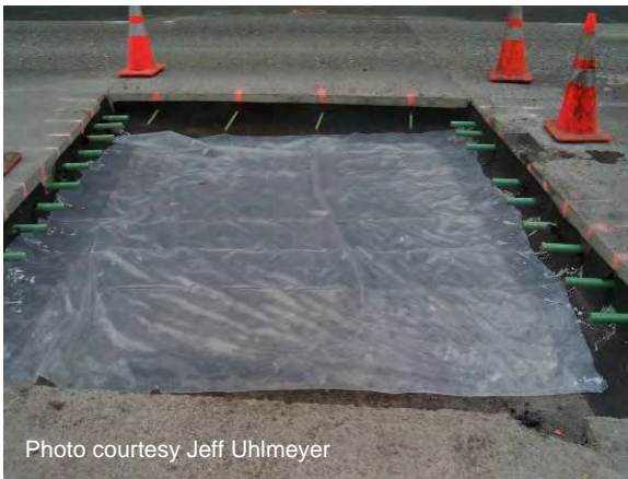
Figure 59 Plastic sheeting to debond concrete from base.
