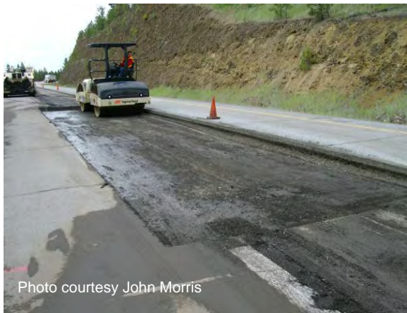
Figure 53 Compacting base.
