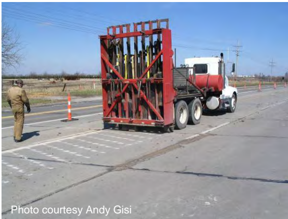
Figure 85 Drop hammer for cracking panels.
