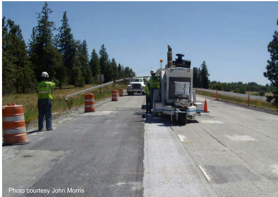
Figure A-82. Diamond grinding equipment.
