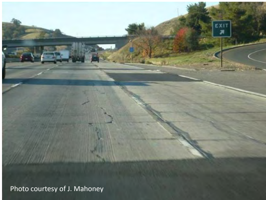
Figure 240 Severely deteriorated concrete pavement (I-80, California).
