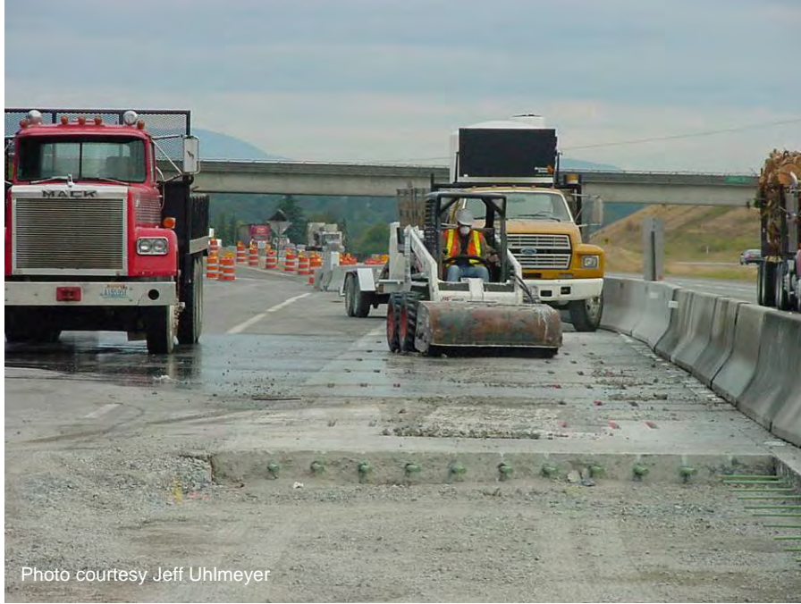
Figure A-33. Debris removal.
