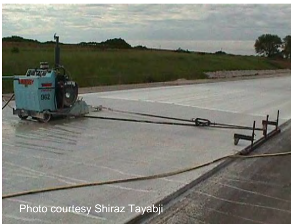
Figure 95 Joint sawing.
