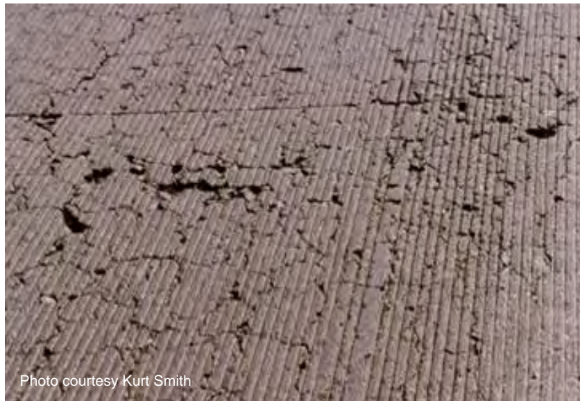
Figure 16 Alkali-Silica Reactivity.
