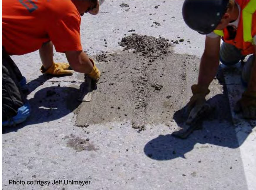
Figure A-71. Finishing patching material.
