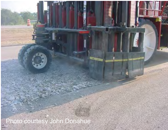
Figure 99 Multi head breaker.
