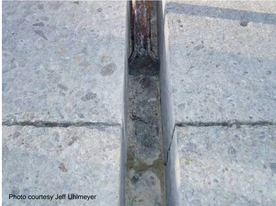
Figure A-26. Leveling dowel bar slot bottom.
