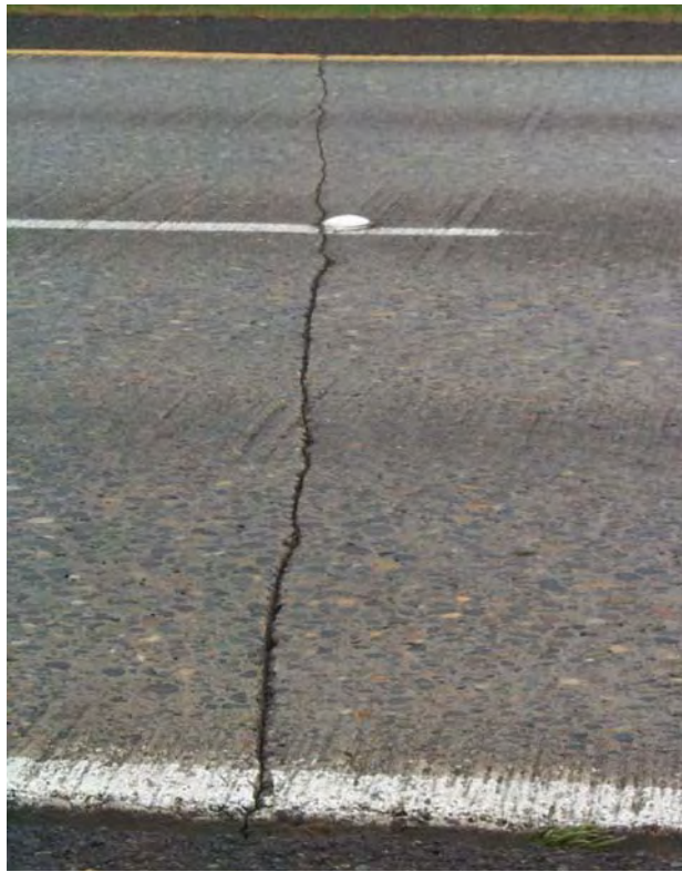
Figure A-77. Transverse tape joint (original construction).
