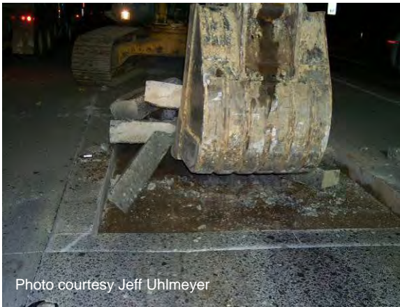
Figure 51 Concrete removal.
