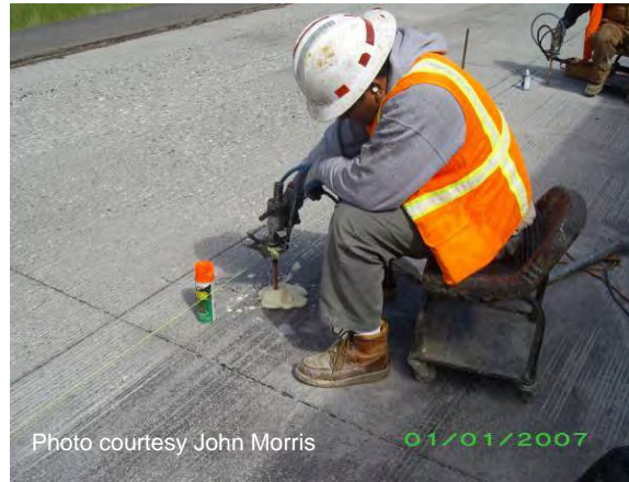
Figure 36 Pressure grouting.
