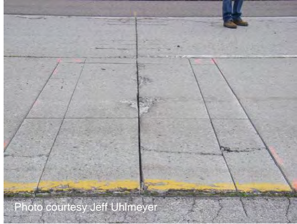
Figure 50 Relief saw cuts.
