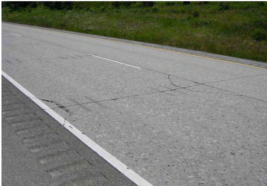
Figure 216 45-degree cracking.
