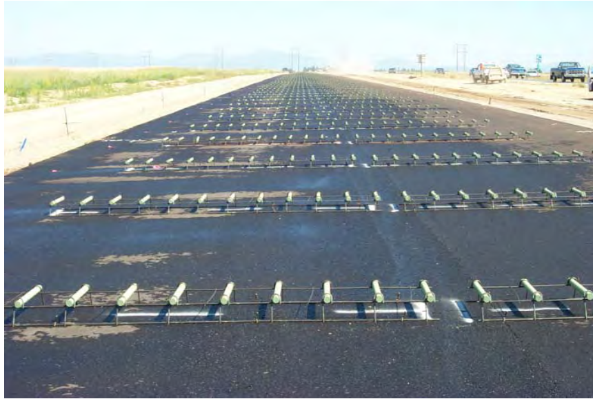
Figure 11 Epoxy coated dowel bars in cages and HMA stabilized base.
