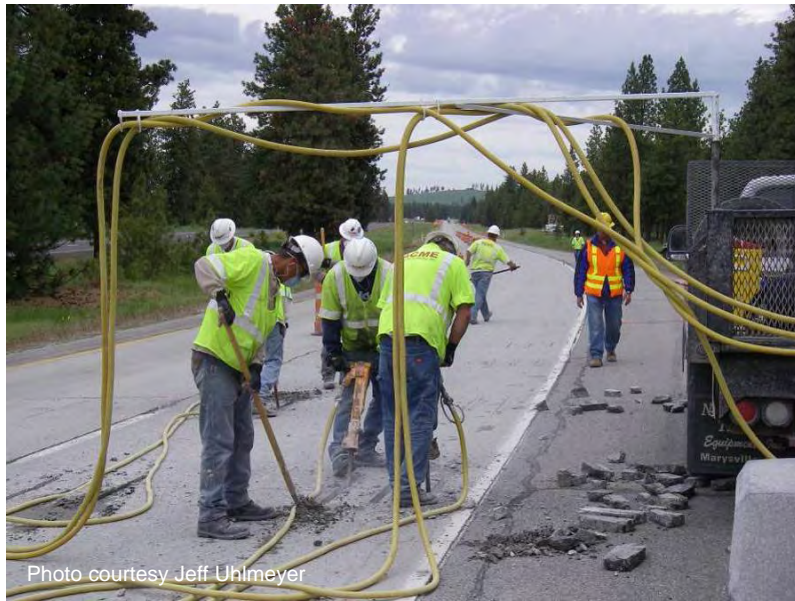
Figure A-24. Jackhammer operation.
