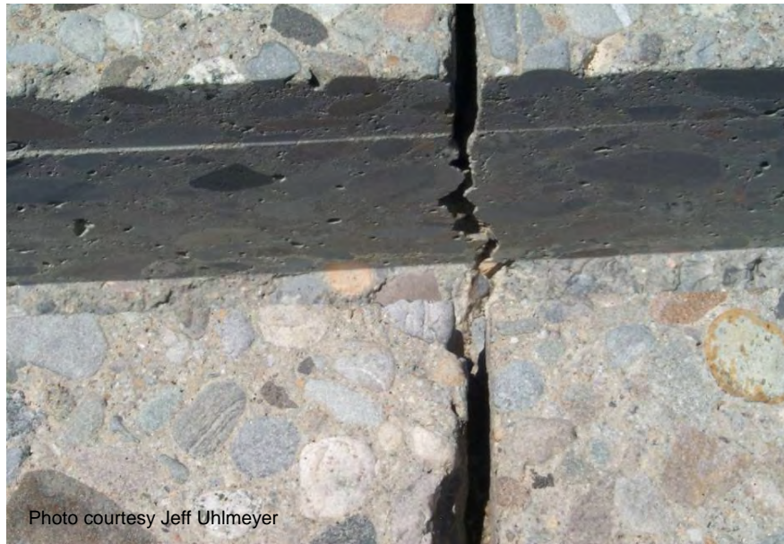
Figure A-42. Cleaned dowel bar slot.
