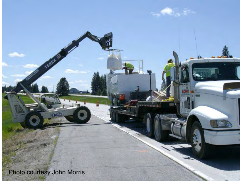
Figure A-62. Delivery of materials to mobile mixer.
