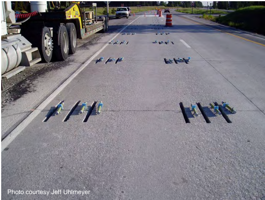
Figure A-53. Dowel bar retrofit assemblies.
