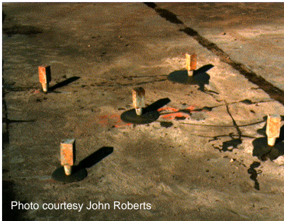
Figure 37 Plugging holes when pozzolan-cement is used.
