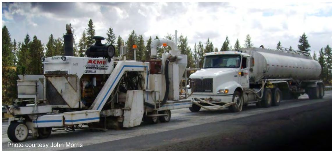
Figure A-81. Diamond grinding equipment.
