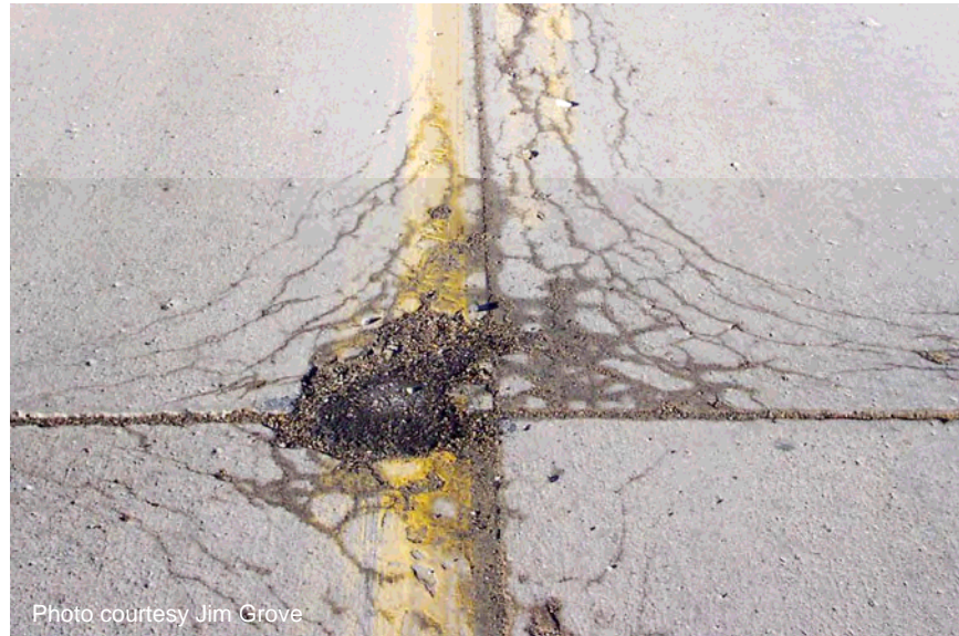
Figure 17 D-cracking.
