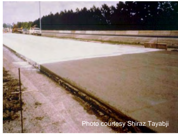
Figure 94 Curing bonded concrete overlay.
