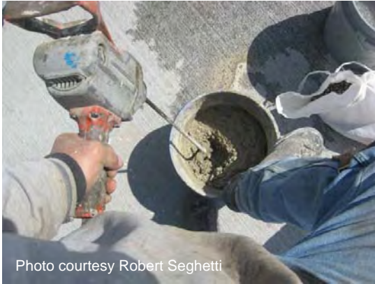
Figure 45 Mixing patching material.
