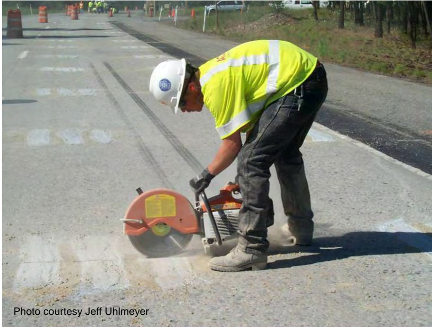
Figure A-76. Establishing joint in patching material.
