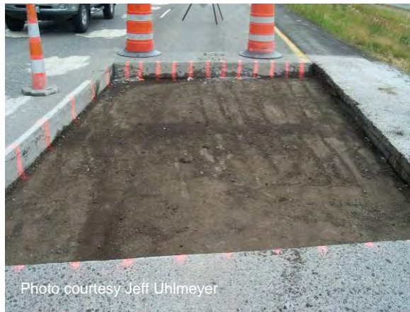
Figure 54 Prepared base.
