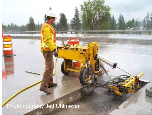
Figure 56 Drilling holes for dowel bars.
