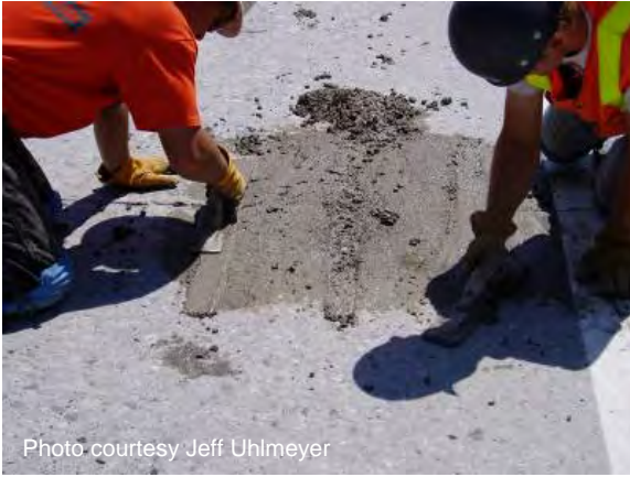
Figure 81 Finishing patching material.
