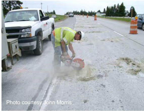
Figure 82 Resawing joint in dowel bar slots.
