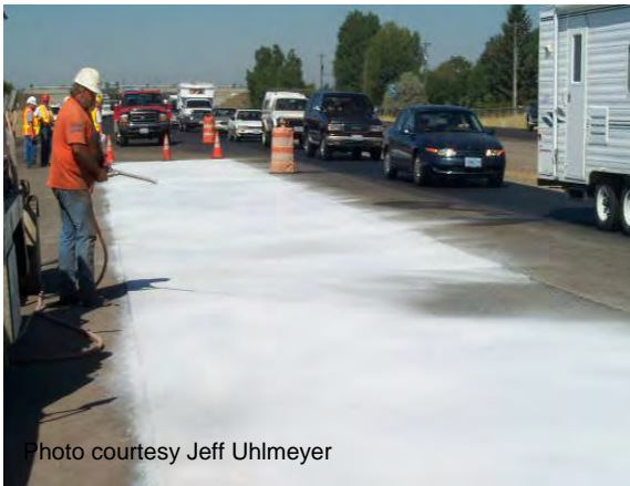
Figure 63 Applying curing compound.
