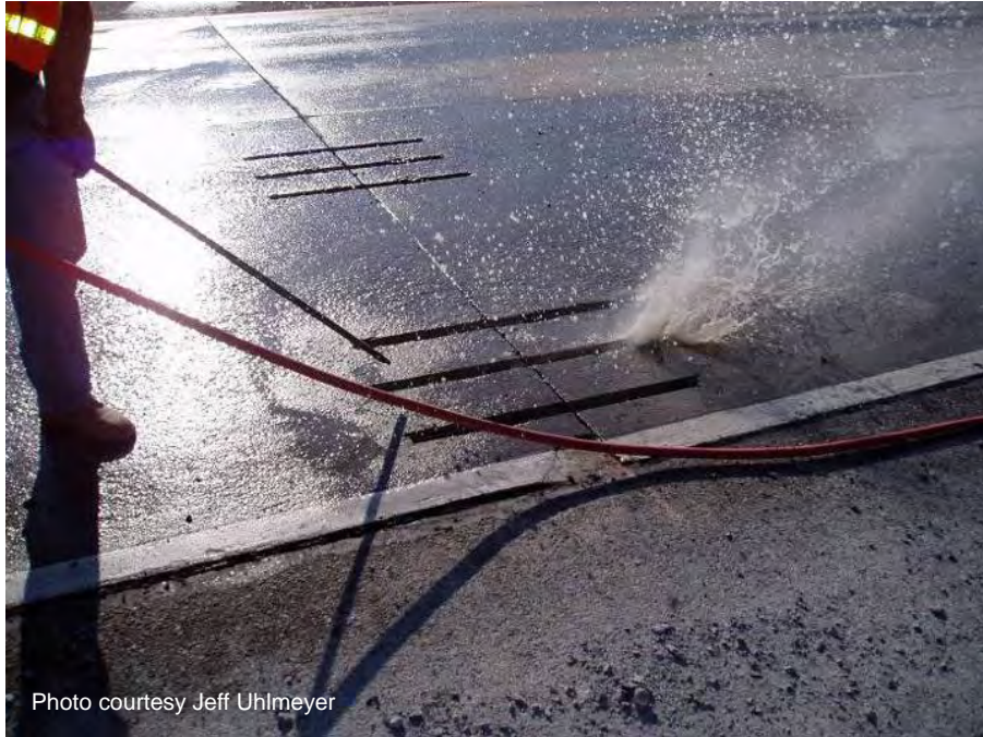
Figure A-40. Removing water and other debris with compressed air.
