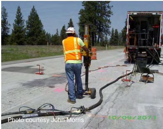
Figure 35 Drilling holes.
