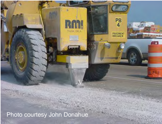
Figure 101 Resonant breaker.
