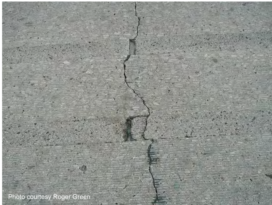
Figure A-67. Misaligned foam core board.
