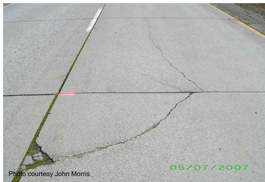
Figure 21 Corner cracking.
