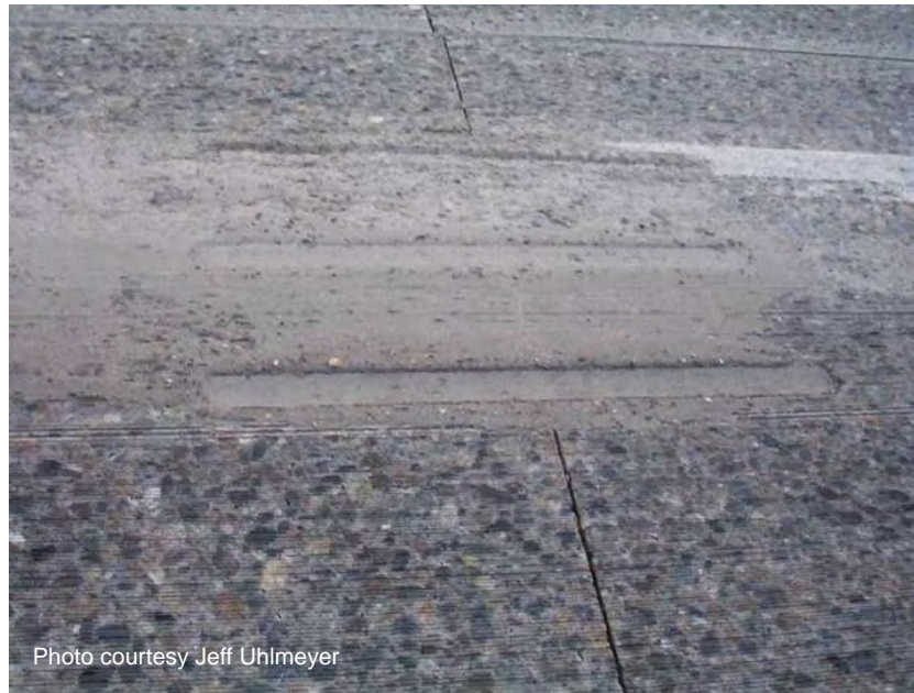
Figure A-78. Mechanical sweeping prior to patching material reaching strength.
