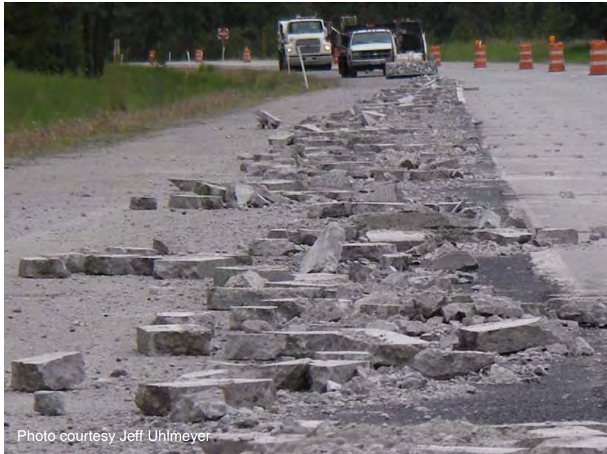
Figure A-32. Debris from the jackhammering process.
