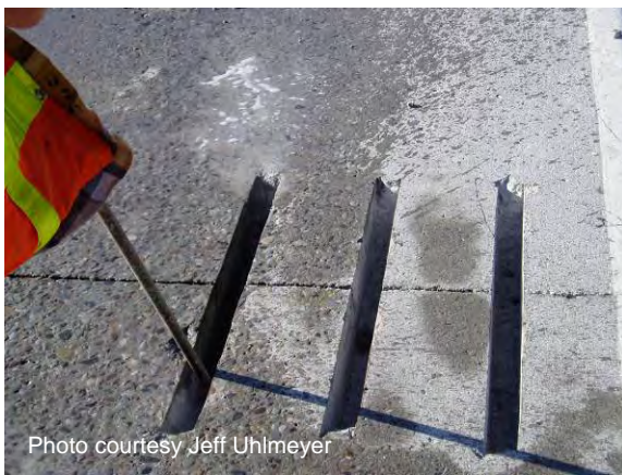
Figure 73 Cleaning dowel bar slots (close-up).
