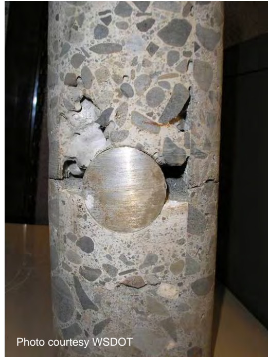
Figure A-70. Poor consolidation.
