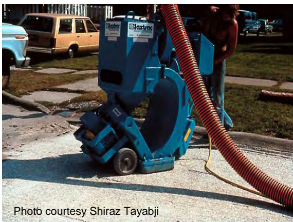
Figure 89 Shotblasting surface.
