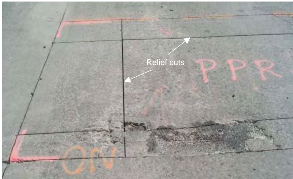
Figure 238 Relief cuts for panel replacements.
