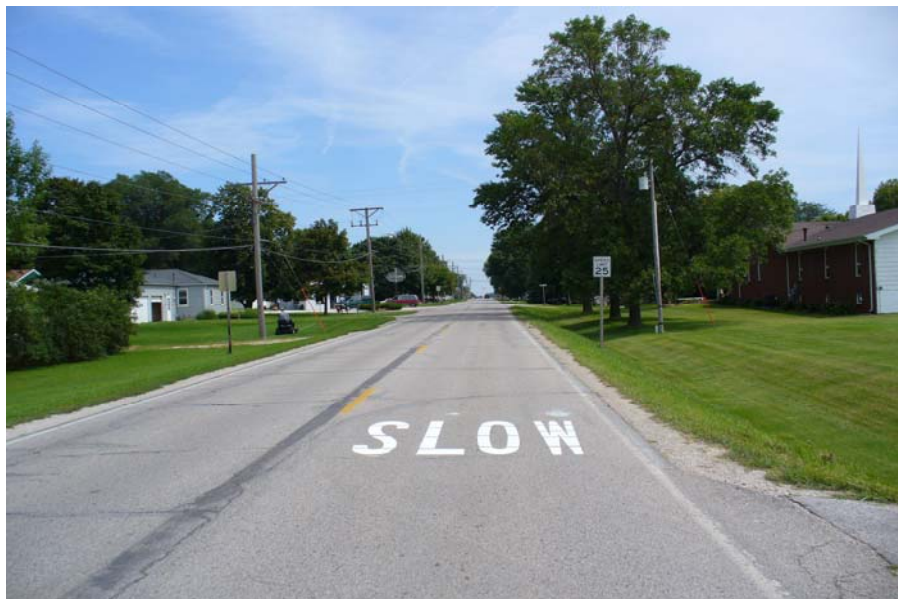
Figure 3.38. Use of on-pavement “SLOW” marking around a pedestrian crossing area in Slater, Iowa
