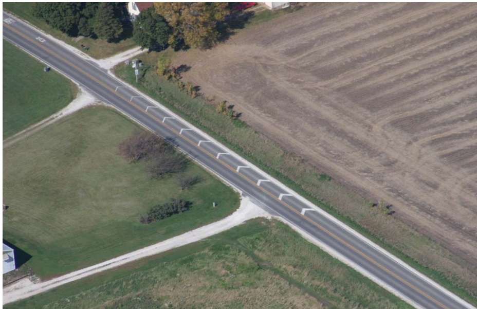
Figure 5.21. Aerial view of Roland treatment
