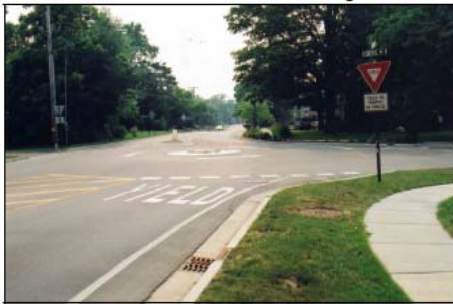
Figure 3.44. Another view of the Dimondale, Michigan installation
