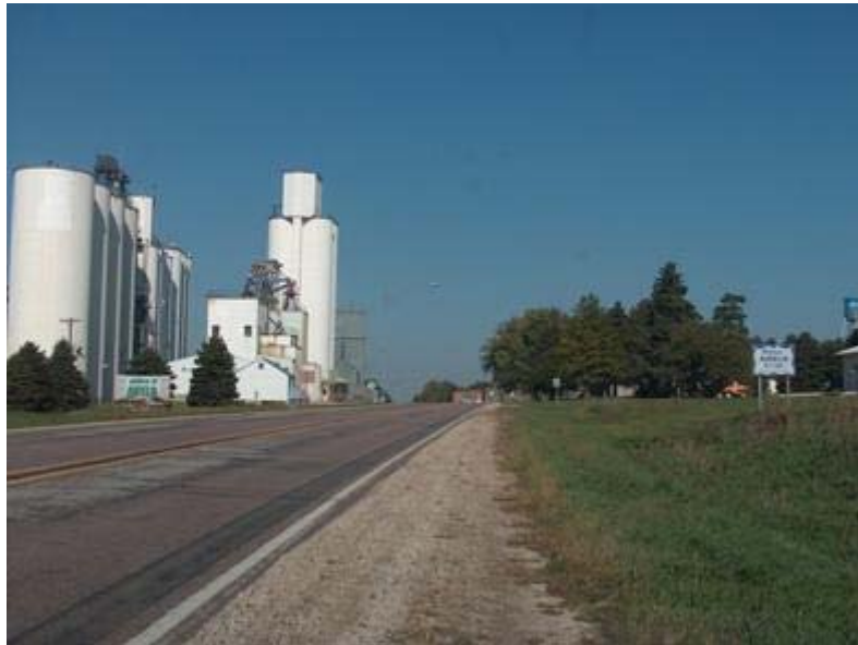
Figure 1.1. Major highway entering a small Iowa community
