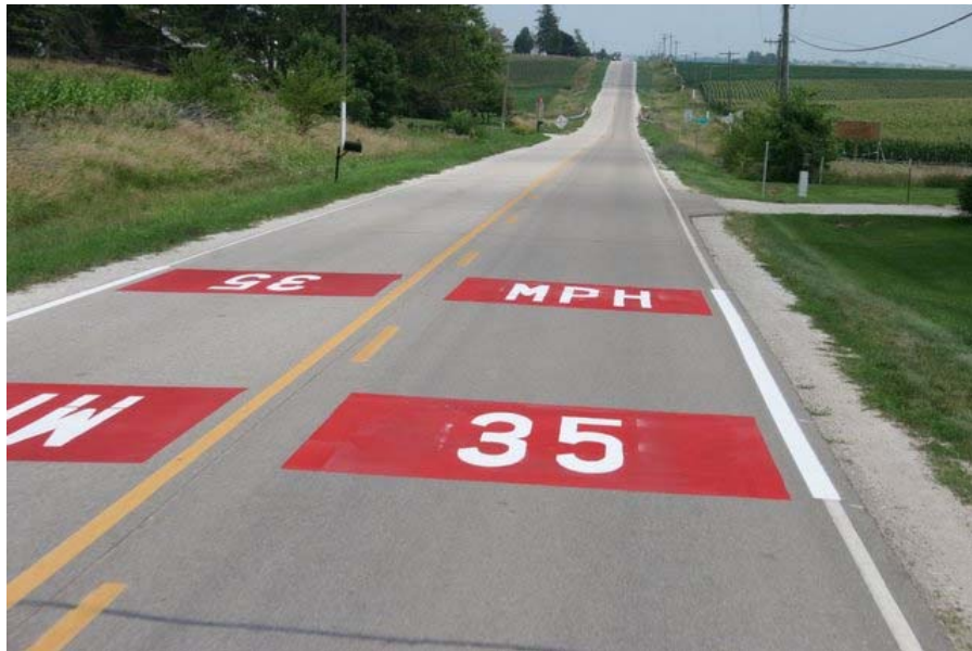
Figure 5.44. After installation of treatment
