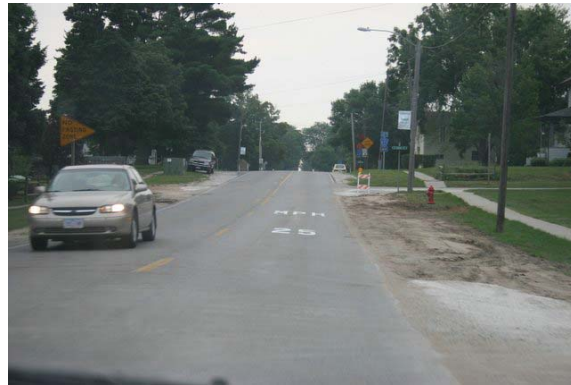
Figure 5.20. On-pavement speed signing
