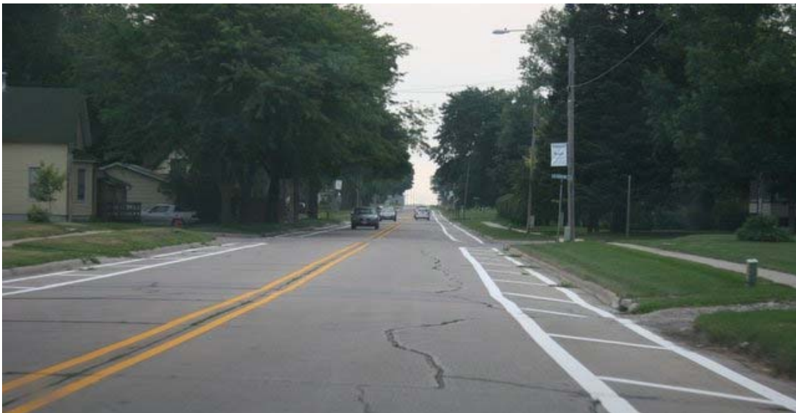
Figure 3.34. Use of shoulder widening in Roland, Iowa as part of gateway treatment
