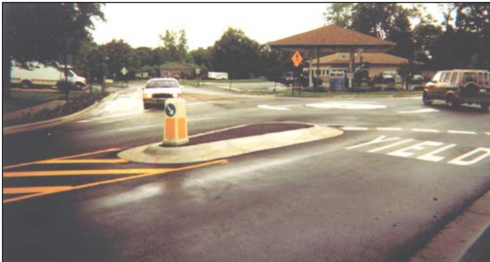
Figure 3.42. Mini-roundabout in Michigan
