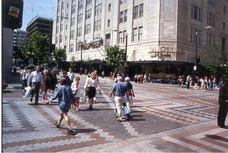
Figure 3.27. Textured surface treatment (source: DWS 2005)
