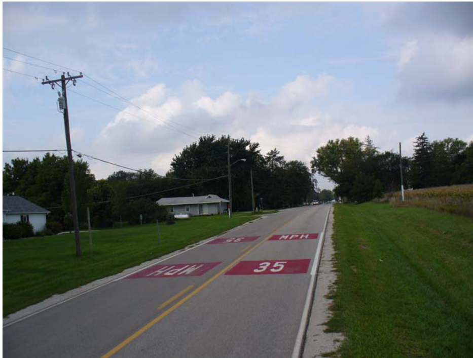
Figure 3.28. Colored pavement markings creating an entrance treatment in Dexter, Iowa
