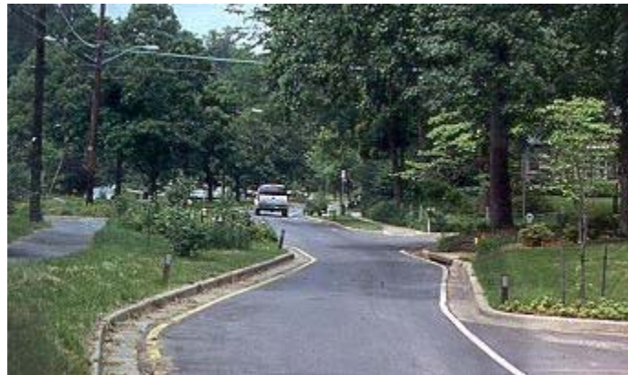
Figure 3.4. Chicanes (source: DSW 2005)
