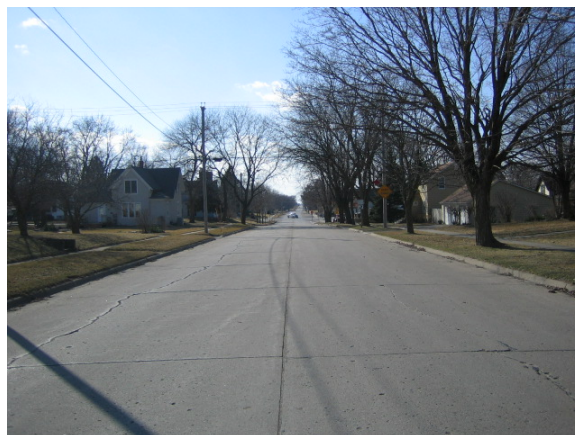
Figure 5.18. East side of E-18 before lane narrowing
