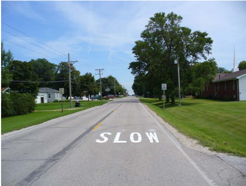
Figure 5.32. Final treatment for western section of SH 210
