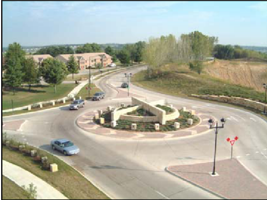
Figure 3.39. Roundabout in Coralville, Iowa (source: Runge 2005)
