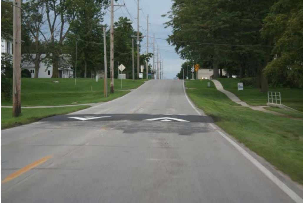
Figure 5.27. Gilbert after installation of speed table
