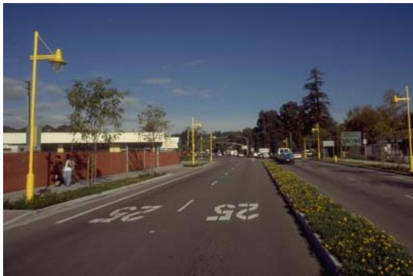
Figure 3.36. Speed limit pavement markings (source: CWS 2005)
