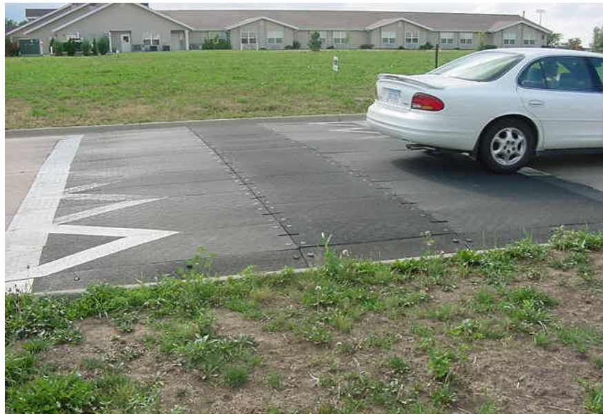
Figure 3.41. 30 mph speed table used in a Center for Transportation Research and Education (CTRE) study for residential traffic calming in small Iowa communities
