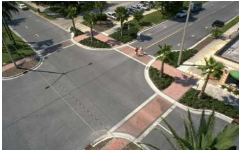
Figure 3.1. Bulb-outs (source: DWS 2005)
