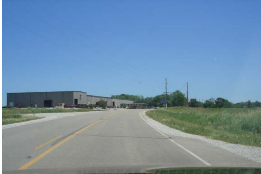
Figure 5.41. Before installation of treatment outside of Dexter industrial plant
