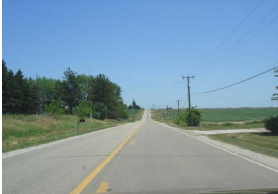
Figure 5.43. Before installation of treatment at Dexter eastern entrance
