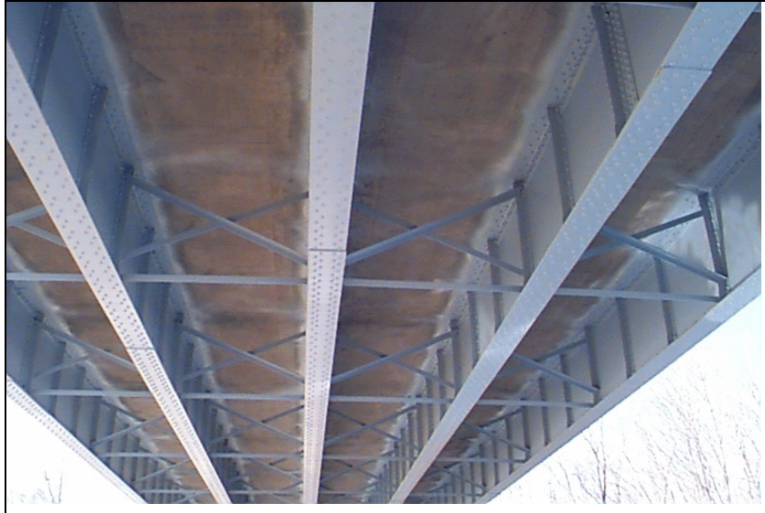
Figure 3: River Rd. over I-90, with no deck cracking (Crowl and Sutak 2002)
