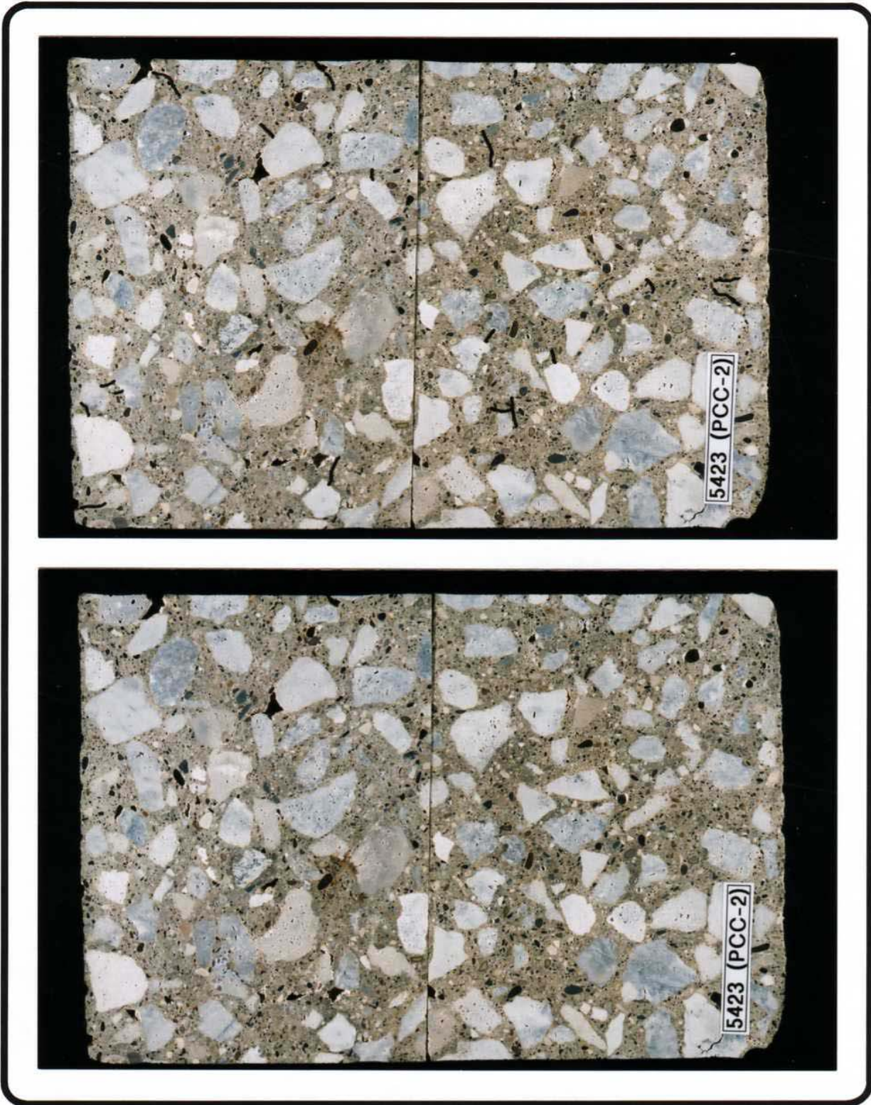
Figure 6.13 - Section View of Core PCC-2
