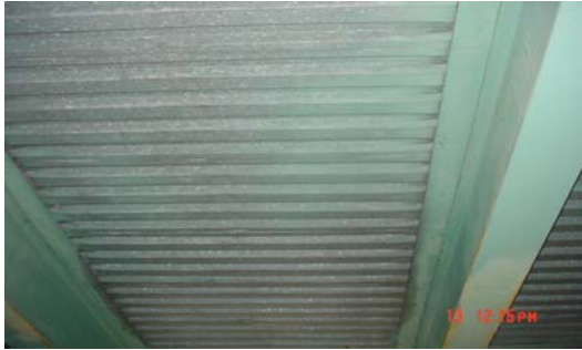
Figure 4. 40-year old SIPMF on Steel Girders
