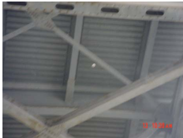
Figure 3. 40-year old SIPMF on Steel Girders
