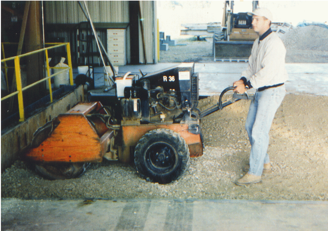
Figure 4.2 Roller Soil Compaction for ATL-Exp #7
