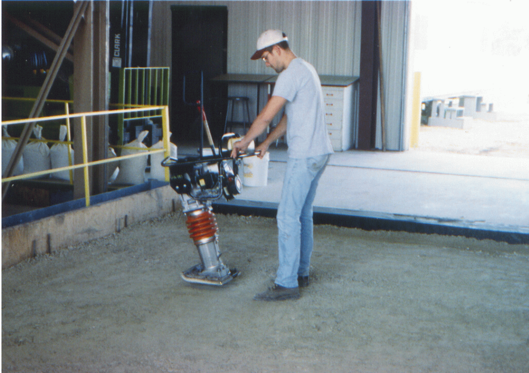
Figure 4.3 Plate Soil Compaction for ATL-Exp #7
