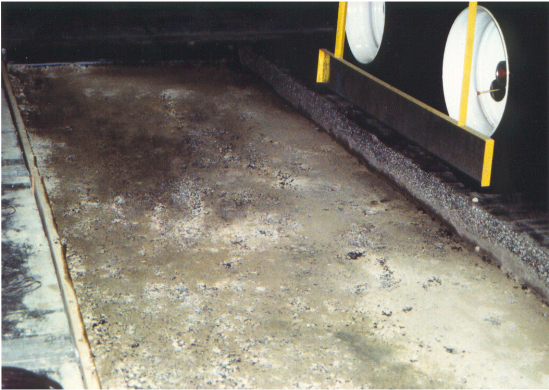
Figure 4.4 Construction of Control Sections in the North Pit of the K-ATL
