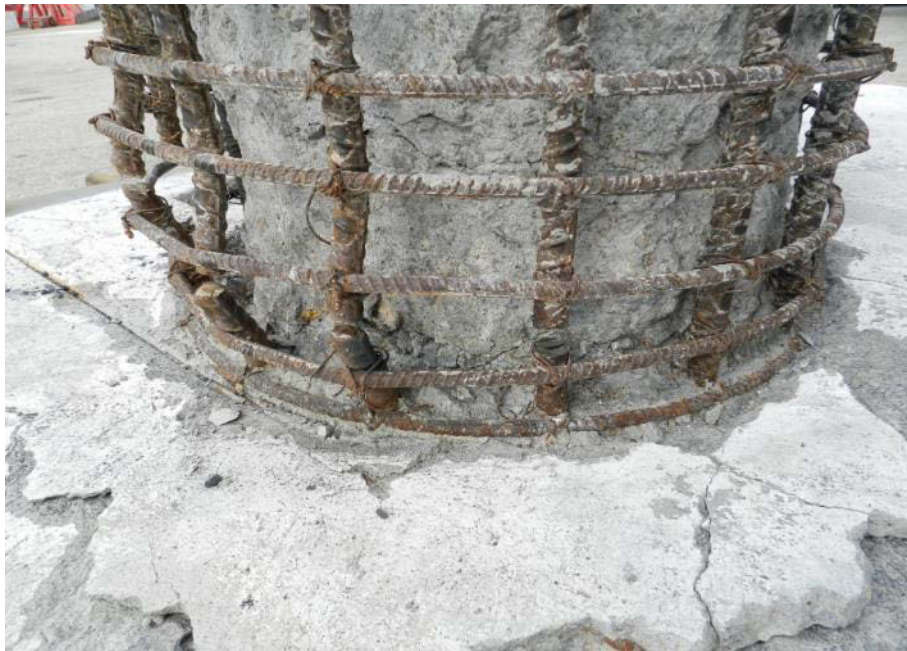
Figure 4.2: Removal and Cleaning of Loose Core Concrete
