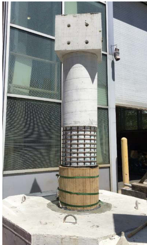
Figure 5.17: Form Work Application
