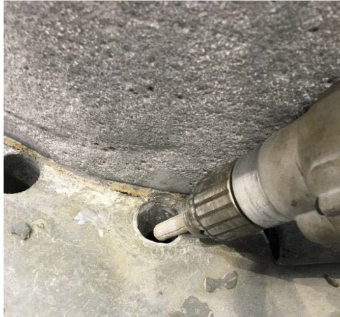
Figure 5.18: Rounding Edges of Anchor Holes
