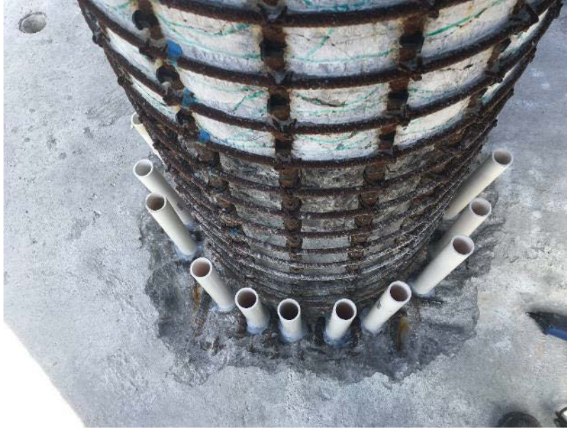
Figure 5.15: PVC Pipe Placed at the top of Anchor Holes with Silicone
