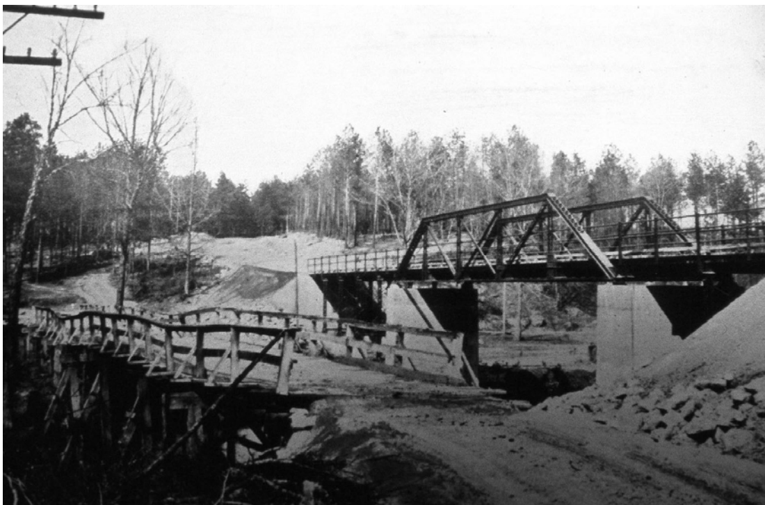
Standardization of bridge plans in the early 1900s resulted in substantial improvement in the condition of Virginia's bridges. This photograph is from the Sixth Annual Report of the State Highway Commissioner (1912).
