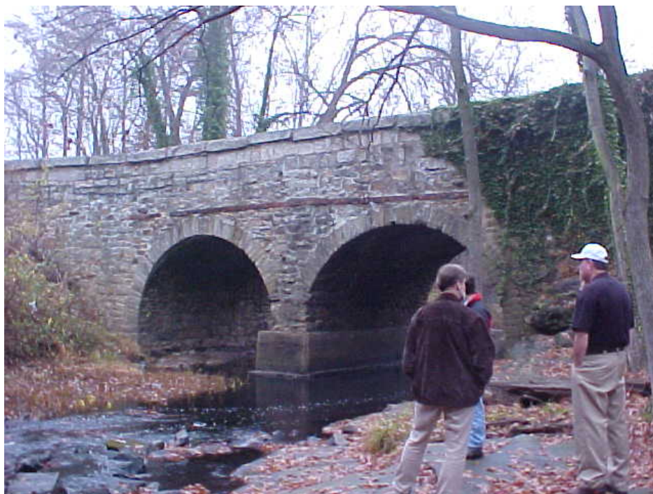
The Falling Creek bridge three years before the storm.
