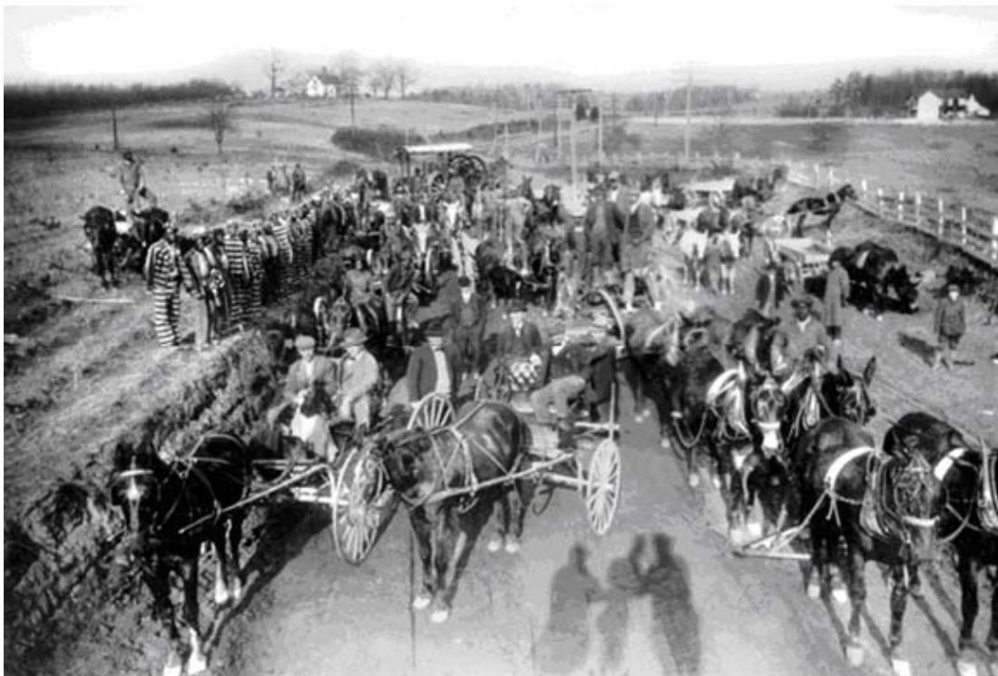
A road crew in the 1910s included hired hands, convict labor, supervisors, and mule teams for the heavy work. The two horses in the photo (foreground) are hitched to light two and four wheel vehicles, and were for speedy transportation, not draft work.
