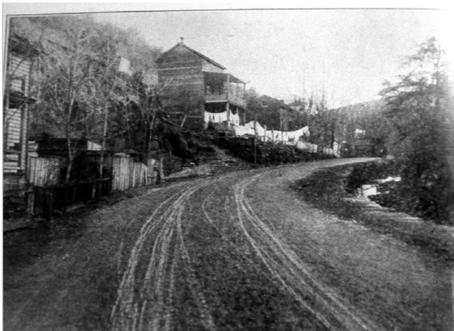
(Above) Section of road in Amherst County. (Below) The same section of road three months later after improvement. These photographs are taken from the First Annual Report of the State Highway Commissioner (1907).
