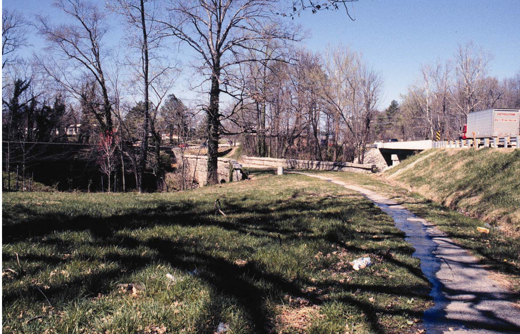
The Falling Creek Wayside before the flooding in August 2004.
