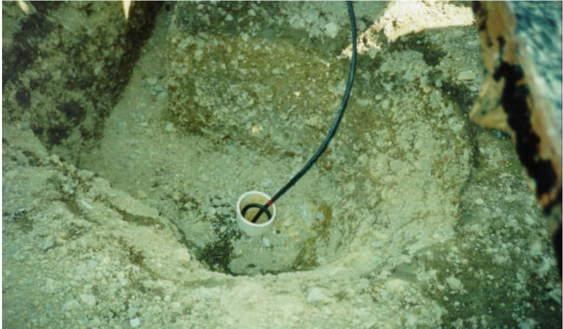
Figure 4.1. Exposed top of 25-ft (7.6 m) casing after installation of FBA; note loop of cable in the casing to provide slack and assure that later operations did not accidentally pull on the cable and lift the FBA from the bottom of the casing
