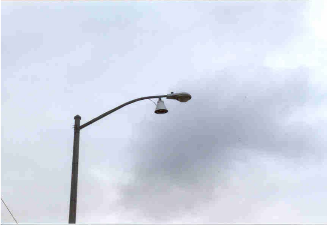
FIGURE 4.1: Camera Mounted on a Lamp Pole (Photo courtesy: Dr. Russell)
