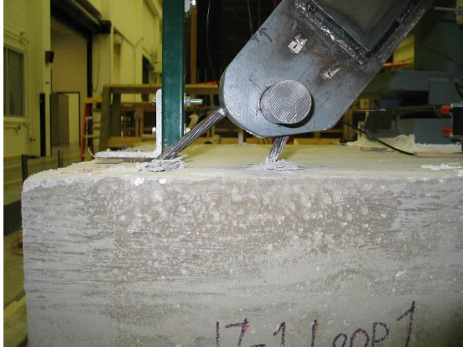
Figure 1: First Cracking (Stage 1)
