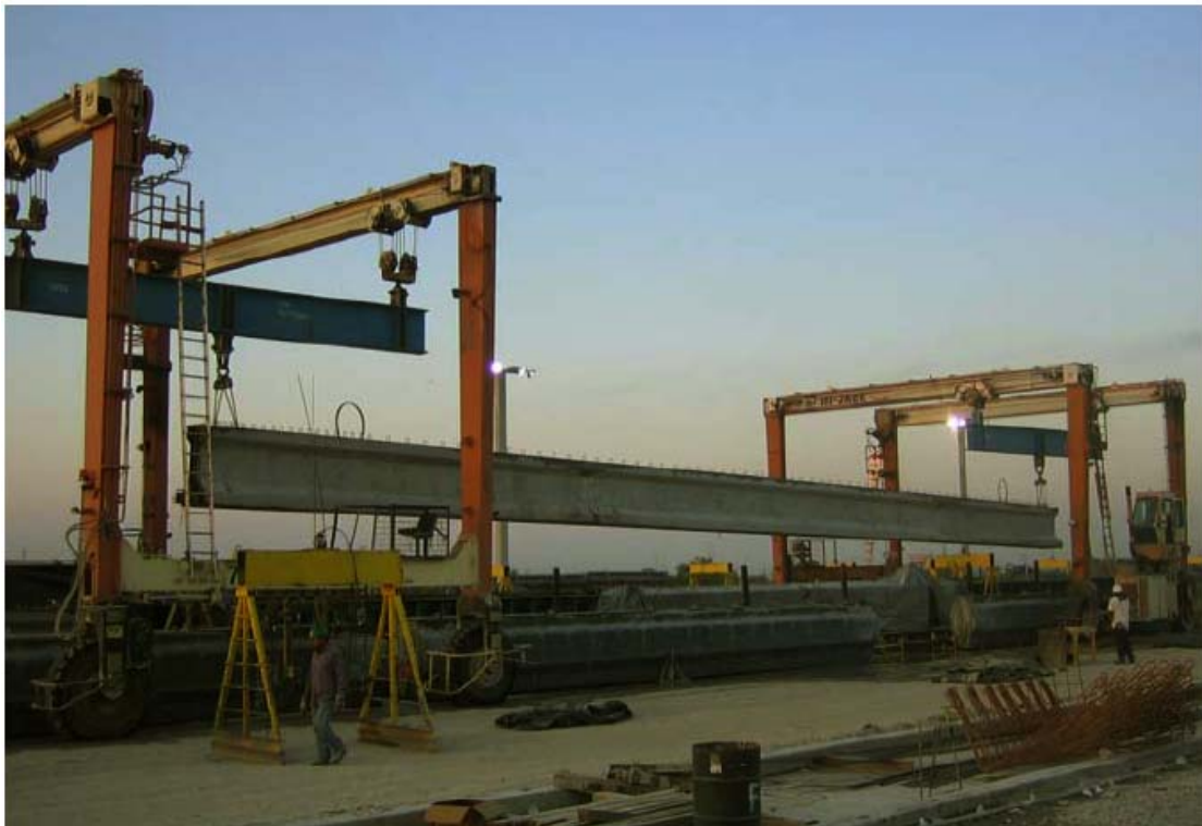
Figure 2. Girder suspended by two out of four lifting loops (Birrcher).
