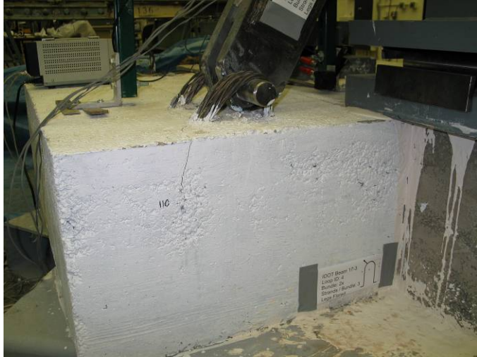
Figure 1: First Cracking (Stage 1)
