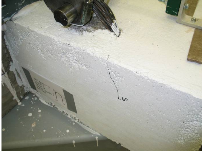
Figure 1: First Cracking (Stage 1)
