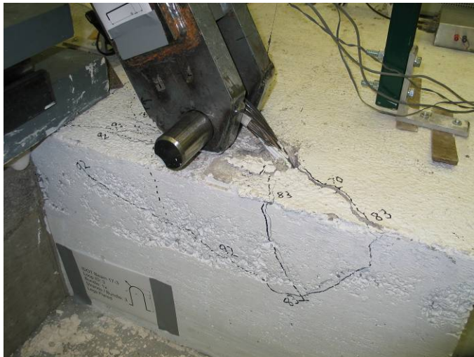
Figure 2: Triangle Wedge Cracking (Stage 2)
