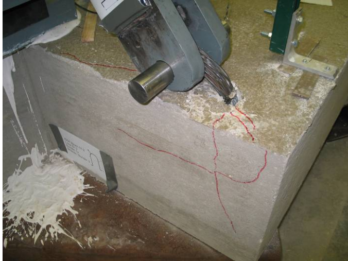
Figure 1: First Cracking (Stage 1)
