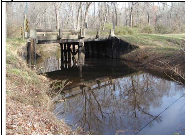
Figure 2.10. This older constricting bridge has caused significant scour downstream
