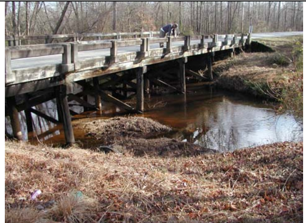
Figure 2.9. A widened channel at this bridge in the Upper Coastal Plain/Piedmont soil system creates some local deposition but does not constrict the channel and scour downstream habitat.
