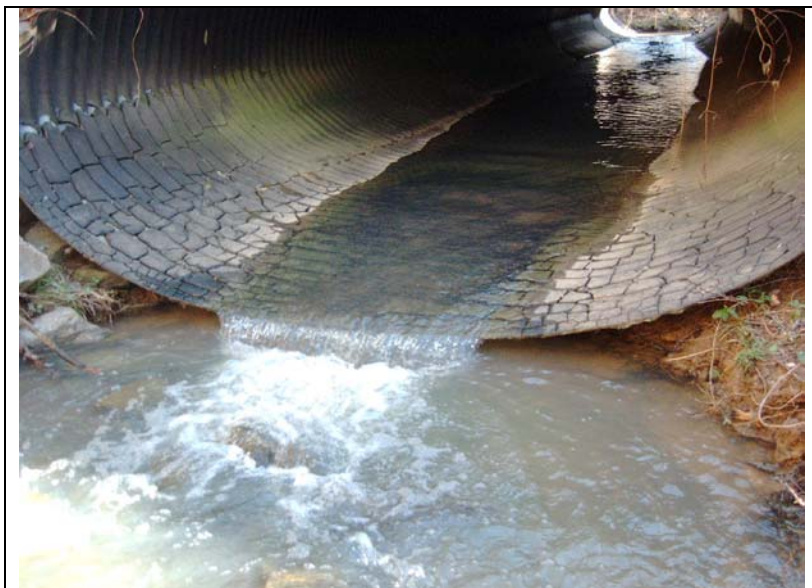
Figure 1.5. Perched Pipe Culvert.
