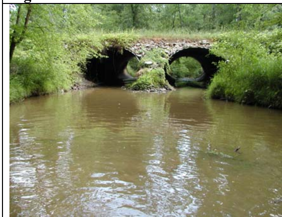
Figure 3. Upstream side of culvert
