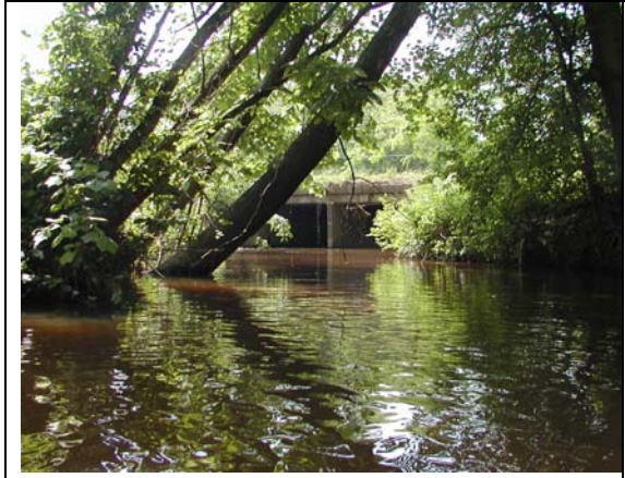
Figure 3. Downstream scour hole
