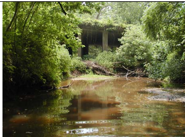
Figure 2. Debris upstream culvert
