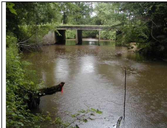
Figure 1. Downstream scour hole
