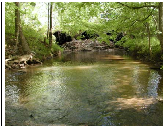
Figure 1. Debris upstream of culvert
