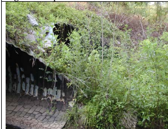
Figure 3. Downstream - perched culvert
