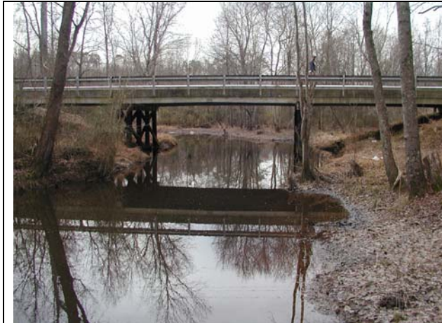
Figure 2.8. A well constructed bridge in the Upper Coastal Plain/Piedmont soil system that does not constrict channel. Downstream habitat appears very similar to upstream.
