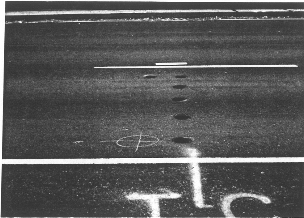
Figure 48. Typical View of C7-C11 Coring Site
