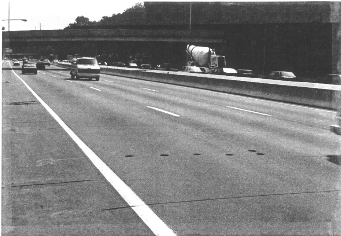
Figure 70. Project 24, Schuylkill Expressway (Section 420)
