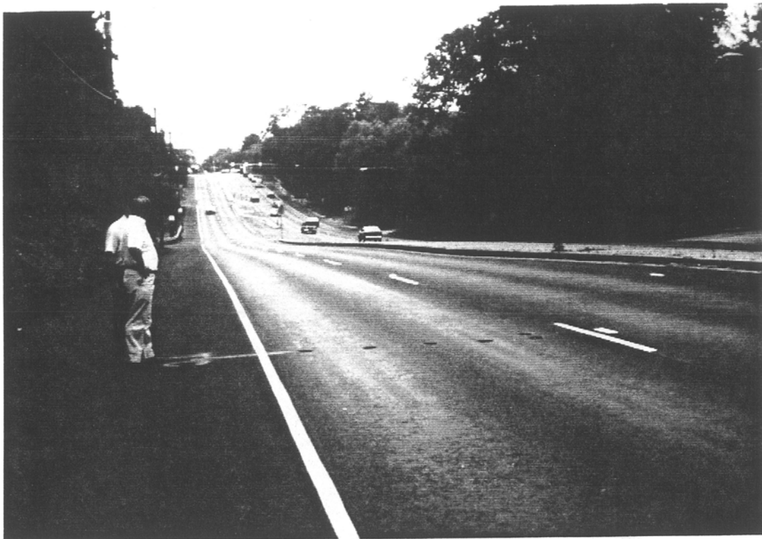
Figure 76. Project 29, Route 11, Camp Hill By-Pass
