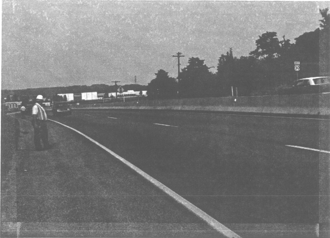
Figure 53. Project 5, Route 30 (E.B.)
