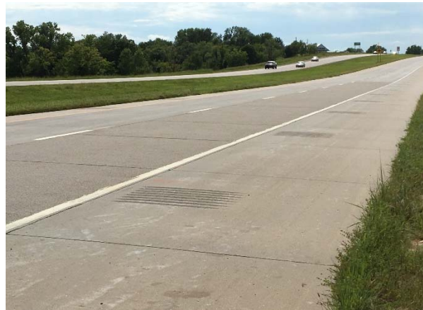
Figure 6.8: Test Strip and Shoulder
