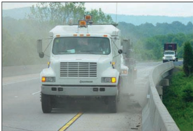
Figure G1.2 Bridge sweeping mechanically (DBi Services, n.d.).
