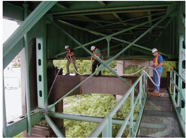
Figure G11.2 Washing superstructure elements with pressure water (Snowden, 2012).
