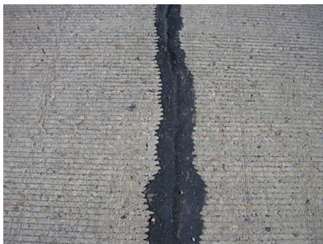
Figure G4.1 Finished deck crack sealing (NYSDOT, 2008).
