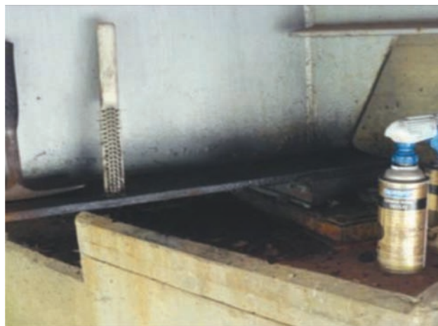
Figure G8.1 Bridge bearing after lubricating (PennDOT, 2010).
