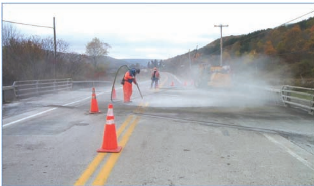
Figure G3.1 Sandblasting concrete deck surface (Fijones & Picard, 2005).
