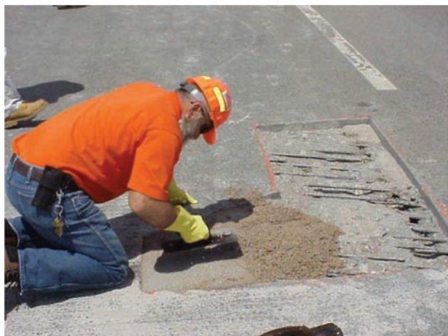
Figure G5.1 Partial deck patching (NYSDOT, 2008).
