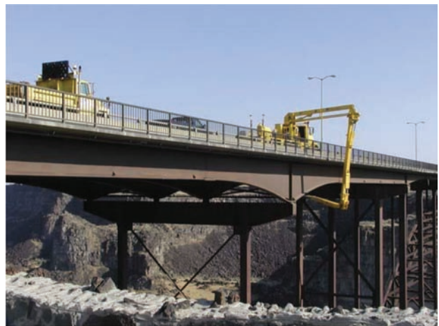
Figure G7.1 Snooper trucks may be required to reach bearings (DBi Services, n.d.).
