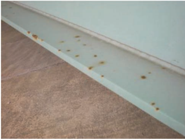
Figure F7.2 Steel girder candidate for spot painting (MoDOT, 2010).
