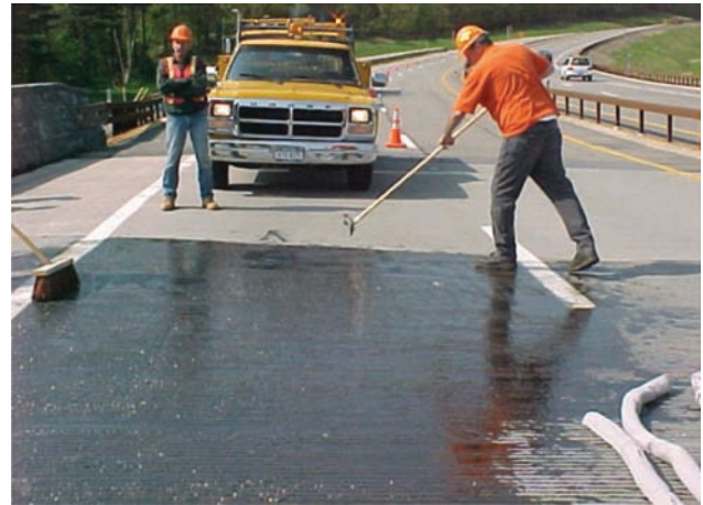
Figure G3.2 Topical application of sealer on deck surface (NYSDOT, 2008).
