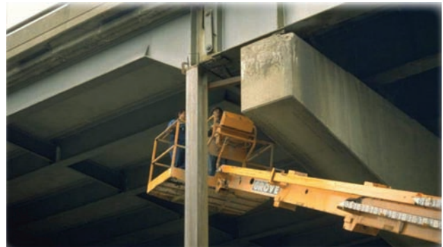
Figure G15.1 Maintenance to pin and hanger connection (Caltrans, 2008).
