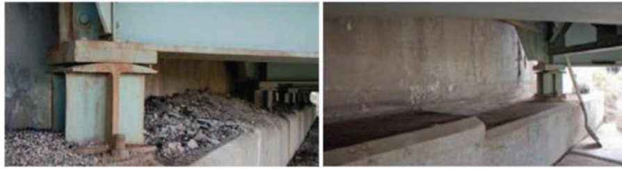
Figure F4.3 Before (left) and after (right) cleaning/washing bridge bearing (Hartman, 2012).
