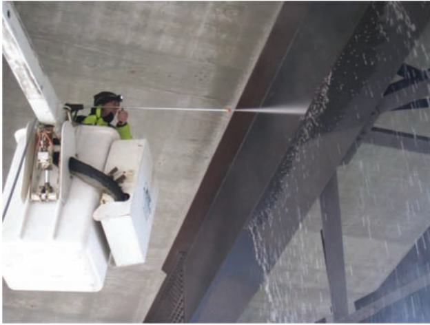
Figure F6.2 Steel bridge superstructure washing (Crampton et al., 2013).
