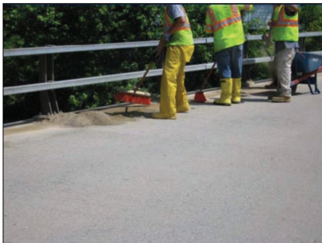
Figure G1.1 Bridge sweeping manually (Marracino & Fox, 2009).
