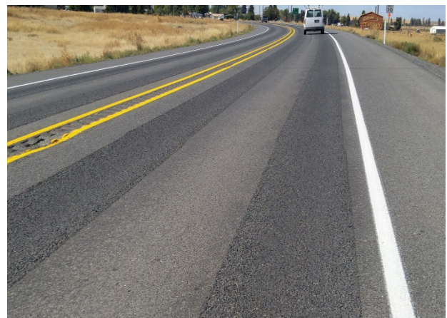
Figure 34. Formula 2 wheel path chip seal after 1.4 months (43 days).
