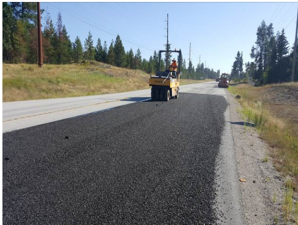
Figure 9. Rolling of chips with pneumatic rollers prior to application of choke stone.
