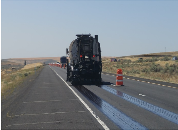
Figure 57. Distributor applying CRS-2P on the I-90 control section.
