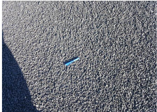
Figure 8. Close-up view of chips prior to rolling.
