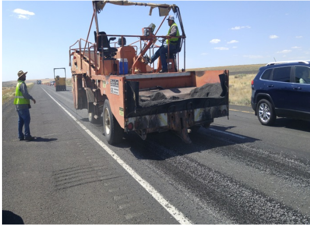
Figure 63. Second chip spreader applying the choke stone.
