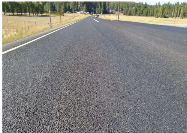
Figure 15. Formula 1 seal after 1.3 months (40 days). A slight hint of flushing in the wheel paths.
