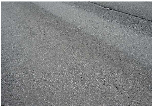
Figure 42. Rutting 4/8 – 5/8 inch at MP 215.00 in WB travel lane.
