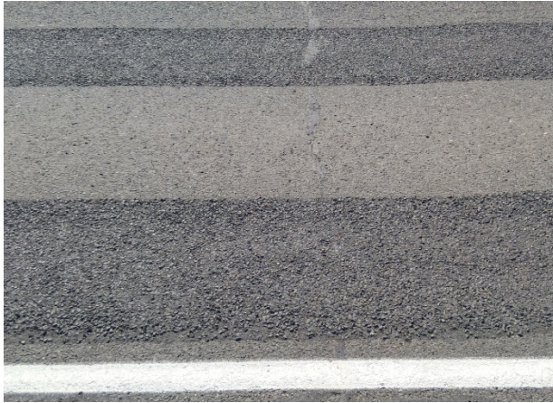
Figure 35. Side view of Formula 2 wheel path chip seal after 1.4 months (43 days) showing no problems.
