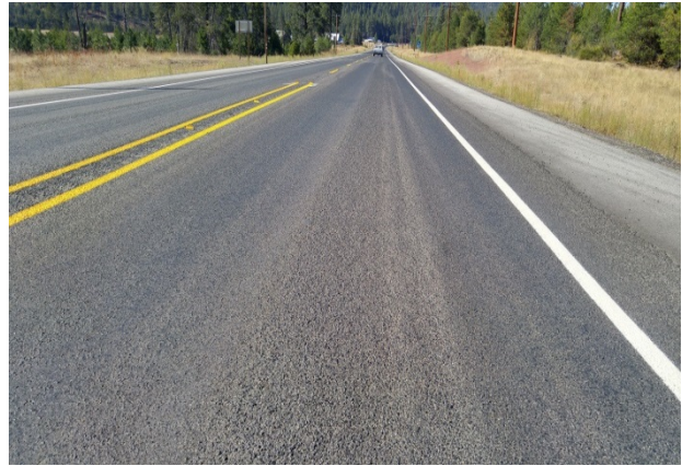
Figure 19. Flushing in the wheel paths of the Formula 1 chip seal after 1.3 months (40 days).
