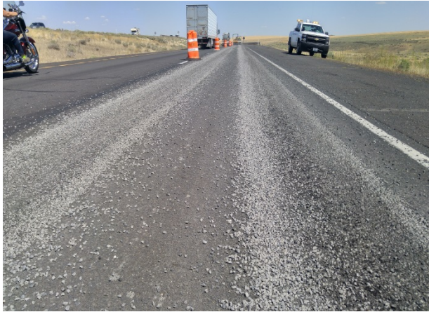
Figure 69. BST during the rolling operation.
