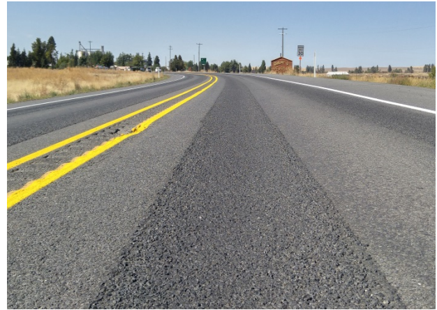
Figure 36. Close-up of the Formula 2 wheel path chip seal showing no problems at 1.4 months (43 days).
