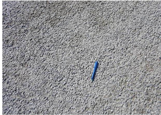
Figure 12. Close-up of the Formula 1 chip seal after application of choke stone.
