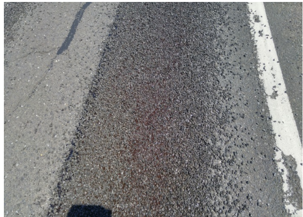
Figure 62. Close-ups of chip seal prior to applying the choke.
