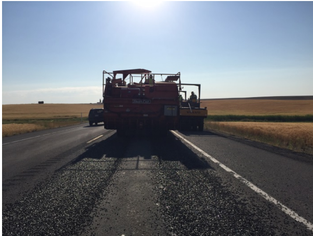
Figure 28. Chips in wheel paths behind the spreader.
