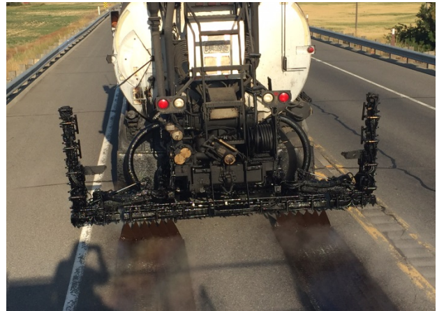
Figure 25. Close-up of distributor spraying the Formula 2 CVRS-2P.
