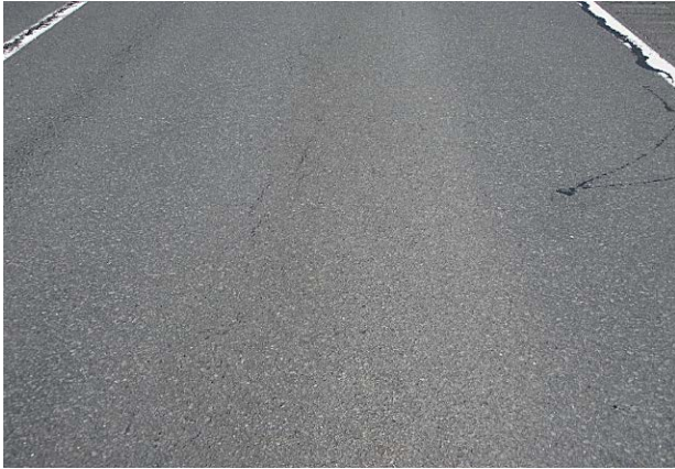
Figure 38. Rutting 3/8 – 4/8 inch at MP 218.00 looking WB travel lane.
