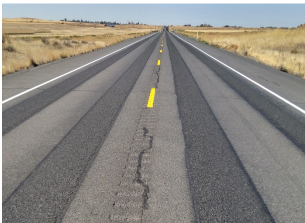
Figure 33. Formula 2 wheel path chip seal after 1.4 months (43 days).
