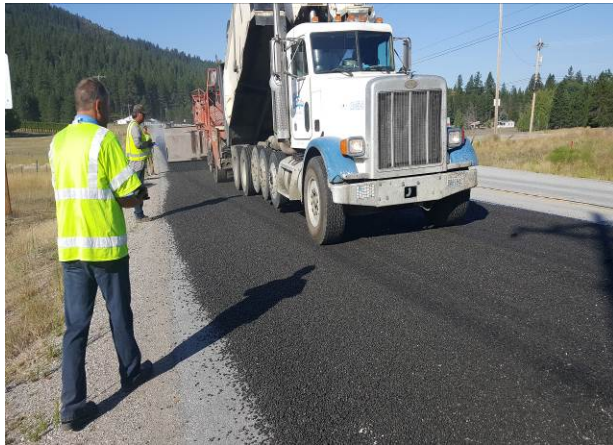
Figure 7. Aggregate applied to the emulsion with a chip spreader fed by a dump truck.
