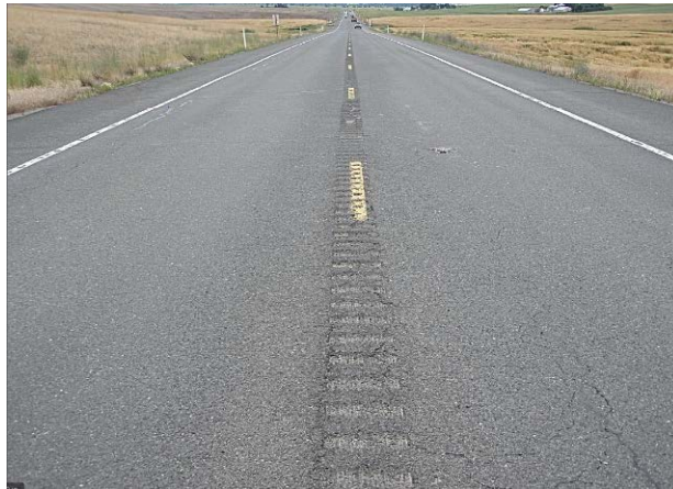
Figure 23. Rutting 5/8 inch at MP 269.00 looking East.
