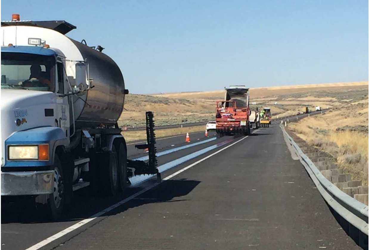
Figure 46. Paving train for Formula 3 test section showing distributor, chip spreader, dump truck and pneumatic rollers.
