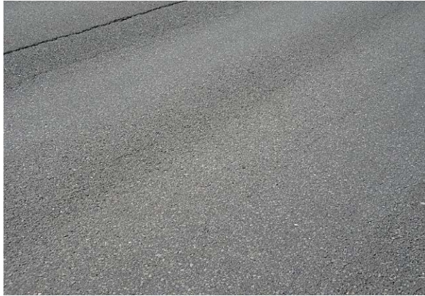
Figure 44. Rutting 3/8 – 5/8 inch at MP 210.55 in the WB travel lane.
