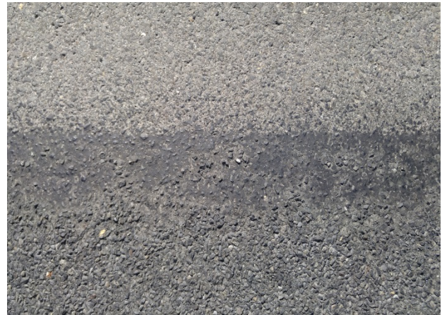
Figure 32. Formula 2 wheel path chip seal after 1.4 months (43 days). Close-up showing missing chips.
