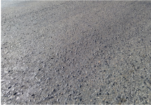
Figure 18. Tight surface of the Formula 1 chip seal. After 1.3 months (40 days).
