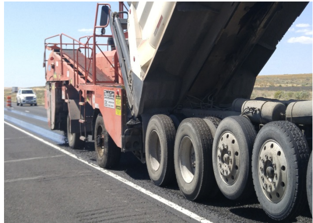
Figure 60. Dump truck loading chip spreader with aggregate.
