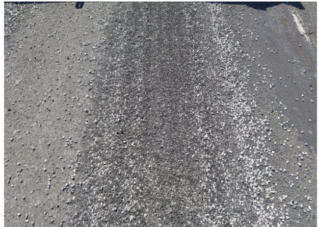
Figure 66. Choked chip seal prior to rolling or sweeping.
