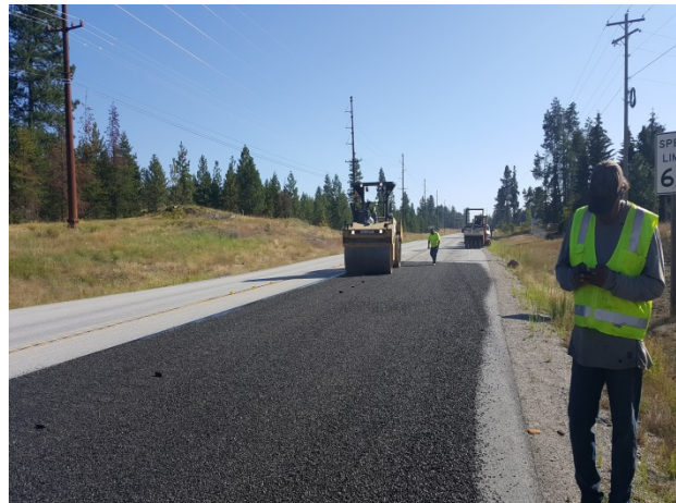
Figure 10. Steel wheel roller used after the application of the choke stone.
