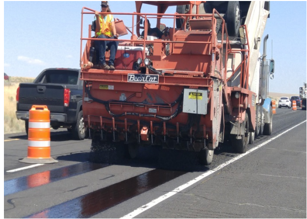
Figure 58. Chip spreader applying aggregate on the I-90 control section.
