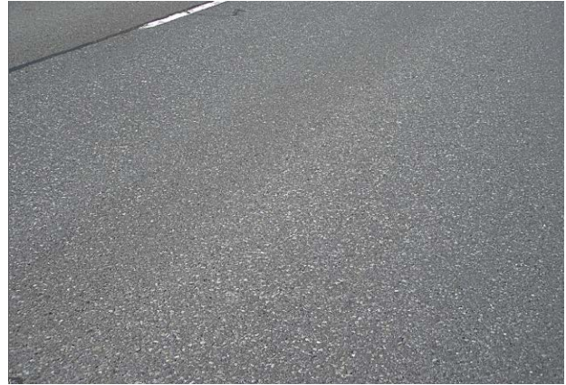
Figure 45. Rutting 3/8 – 3/8 inch at MP 208.25 in the WB travel lane.
