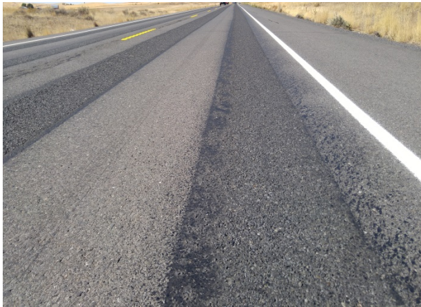
Figure 31. Formula 2 wheel path chip seal after 1.4 months (43 days). Edges of wheel path chip seals have lost chips.
