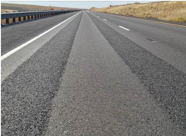
Figure 55. Very minor loss of chips at the edges of the wheel paths on the Formula 3 test section after 1 month.
