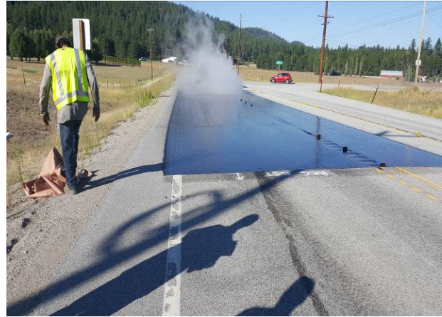
Figure 6. Application of the Formula 1 CVRS-2P.
