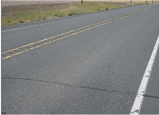
Figure 21. Rutting 5/8 inch at MP 266.00 looking East.
