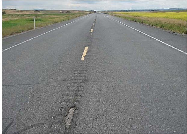
Figure 22. Rutting 5/8 inch at MP 267.00 looking East.
