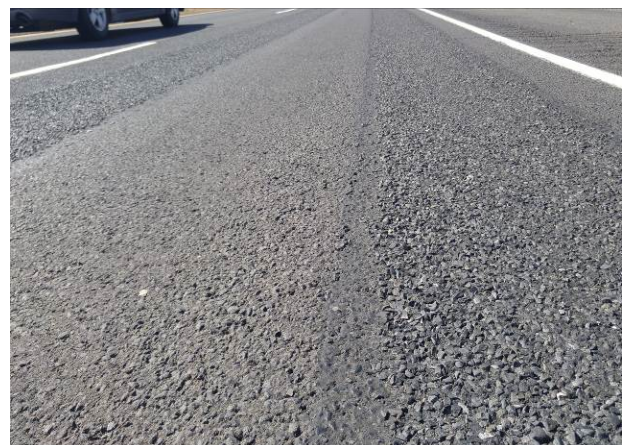
Figure 52. Loss of chips at the wheel path edges. Formula 3 test section after 1 month.
