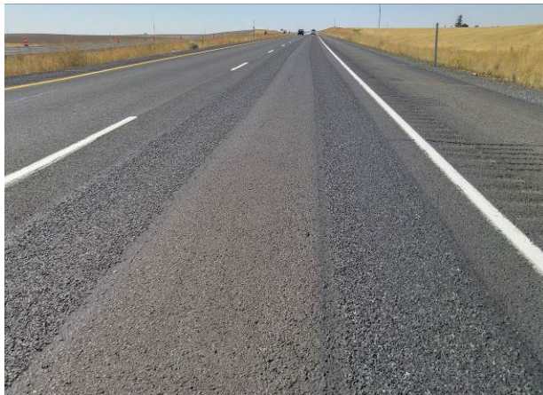
Figure 49. Minor chip loss at the edges of the Formula 3 wheel path chip seal after 1 month.
