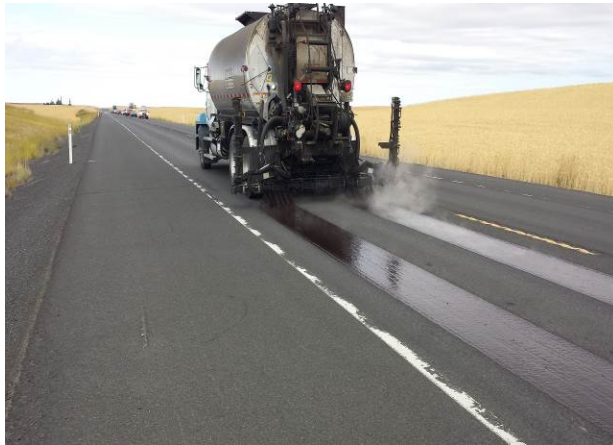
Figure 24. Distributor applying the Formula 2 CVRS-2P in the wheel paths of US 2.
