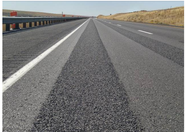
Figure 56. Very minor loss of chips at the edges of the wheel paths on the Formula 3 test section after 1 month.
