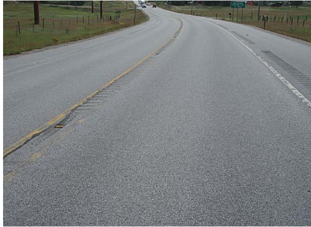
Figure 4. Rutting 1/8 inch at MP 322.5 looking East.
