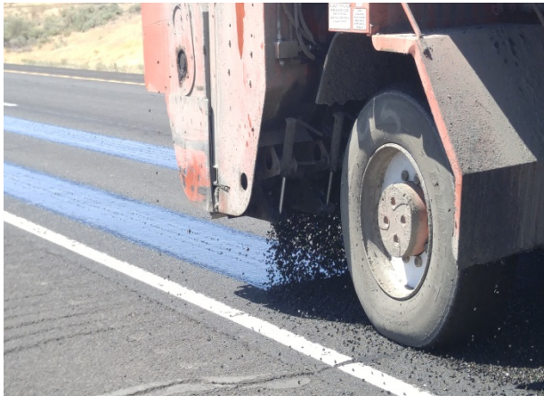
Figure 59. Close-up of chip spreader dropping chips on the CRS-2P.
