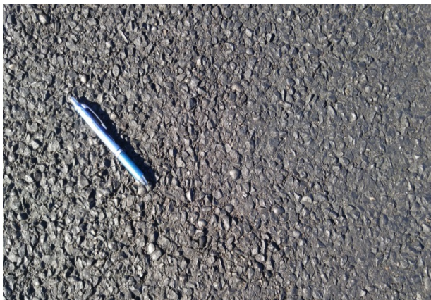
Figure 16. Close-up of the surface of the Formula 1 chip seal after 1.3 months (40 days).
