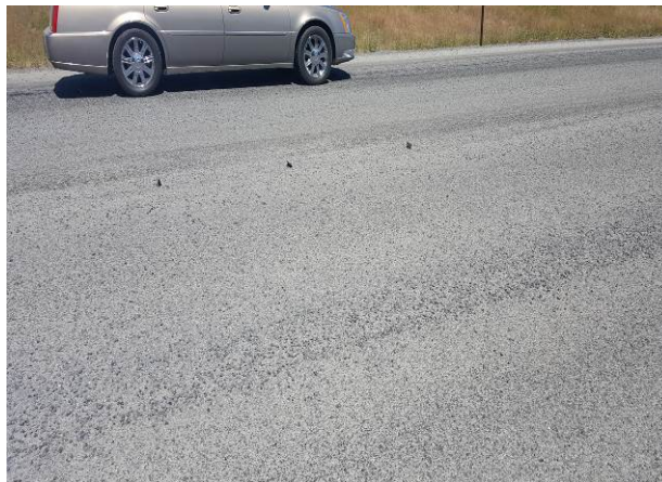
Figure 13. Finished Formula 1 CVRS-2P chip seal.
