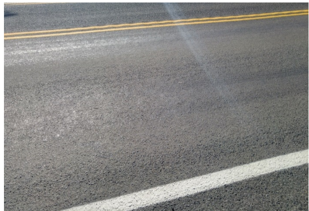
Figure 17. Hint of flushing in the wheel paths of the Formula 1 seal after 1.3 months (40 days).
