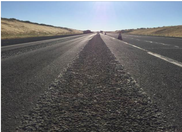
Figure 47. Finished Formula 3 wheel path chip seal with choke.
