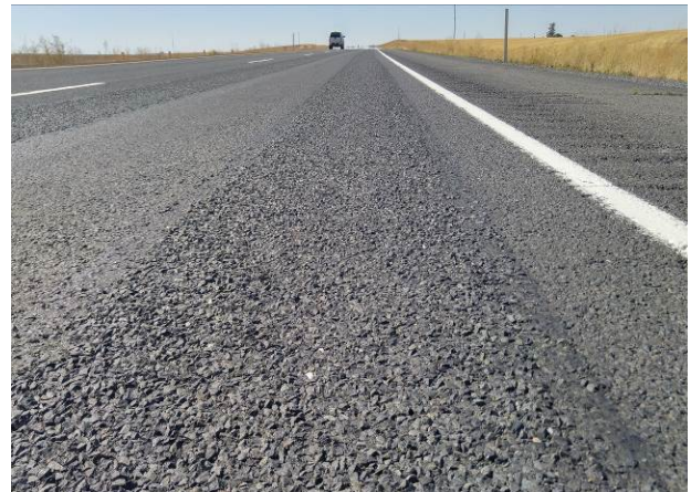
Figure 50. Minor chip loss at edges of the wheel paths Formula 3 chip seal after 1 month.
