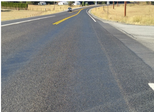
Figure 14. Formula 1 chip seal after 1.3 months (40 days). Some flushing in the wheel paths.
