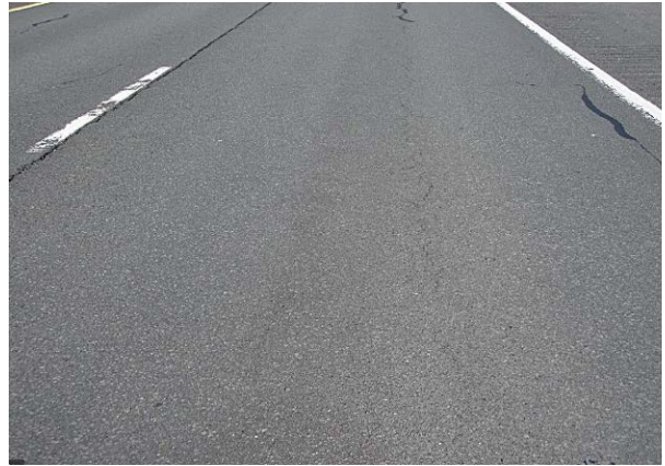
Figure 39. Rutting 3/8 – 4/8 inch at MP 217.00 in WB travel lane.
