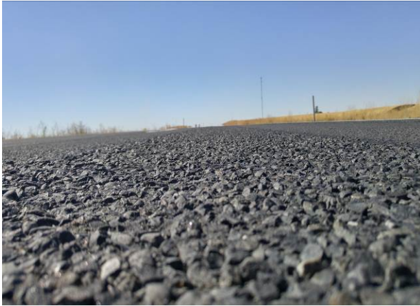
Figure 53. Coarse nature of the Formula 3 chip seal after 1 month.
