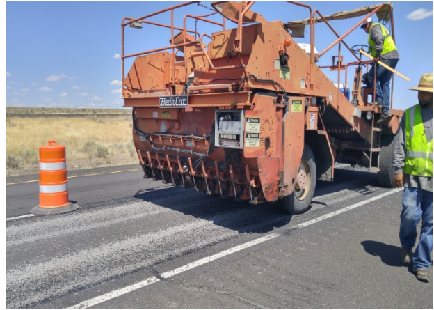
Figure 64. Close-up of the chip spreader for the choke stone.
