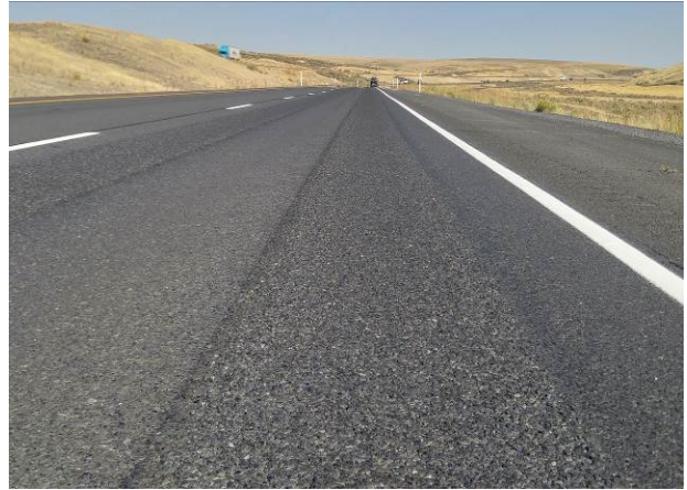
Figure 54. Minor loss of chips at the edges of the wheel paths on the Formula 3 test section after 1 month.
