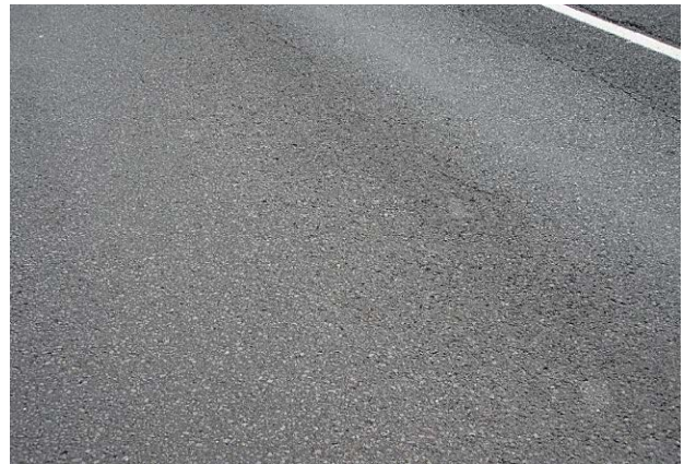
Figure 41. Rutting 3/8 – 6/8 inch at MP 215.29 in WB travel lane.
