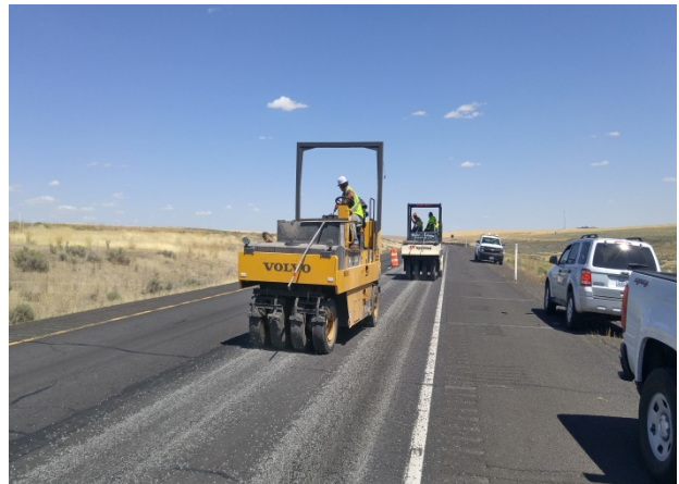
Figure 68. Pneumatic rollers at work.
