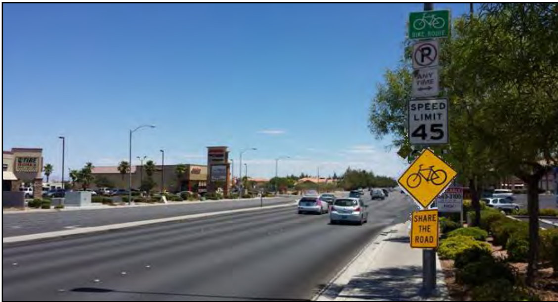
Figure 7. Share the Road Concept: A Slightly Wider Right Lane that is Shared by Both Bicycles and Vehicles
