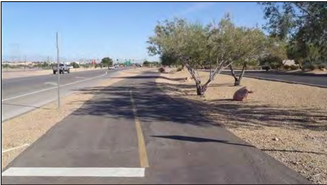
Figure 8. Paved Multiuse Trail: A Paved Bike Trail that is Completely Separated from Traffic
