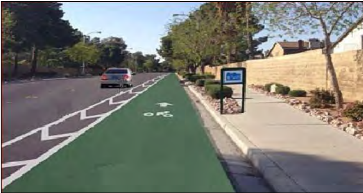
Figure 4. Enhanced Buffered Lane: An 8-Foot Bike Lane, with 3-Foot Buffers, Located on a Minor Roadway (Collector Street)
