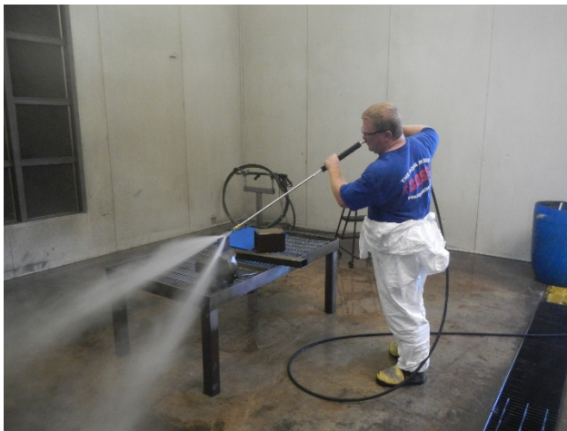
Figure 9. Pressure washing surface preparation.
