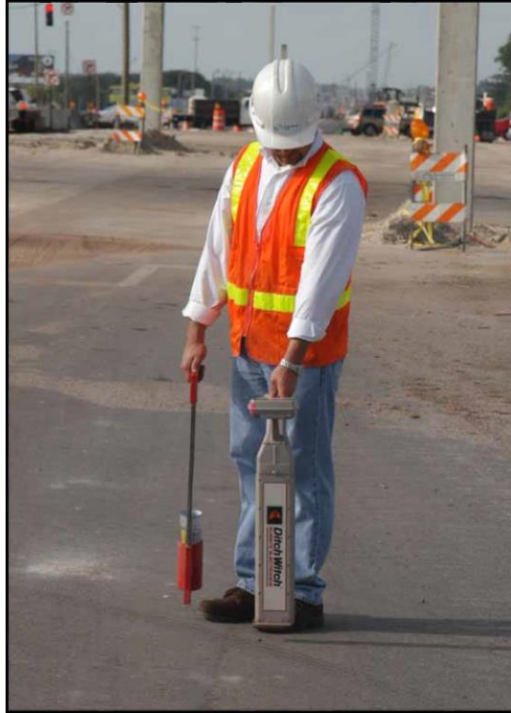
Figure 6. Photo. EMI pipe and cable locator.
