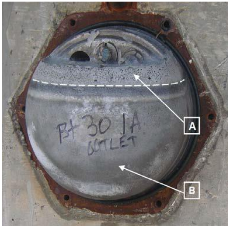
Figure 144. Photo. Anchorage region of a tendon from the Carbon Plant Road Bridge subsequent to endcap removal. Part A was soft, segregated, and wet grout, and part B was gray, hardened, and dry grout. (15)
