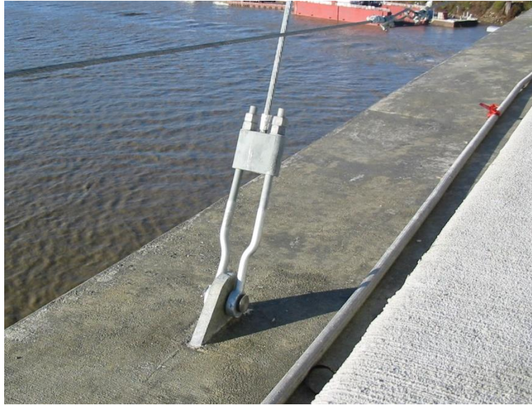
Figure 18. Photo. Anchorage attaching the line of crossies to the deck.
