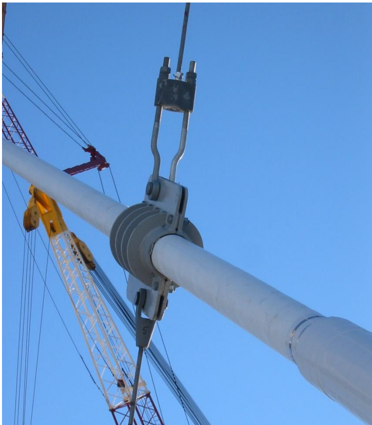
Figure 17. Photo. Close-up view of the crosstie cable clamp and bolt assembly.
