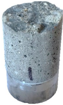
Figure 108. Photo. Interface failure mode in direct tension pull-off tests.
