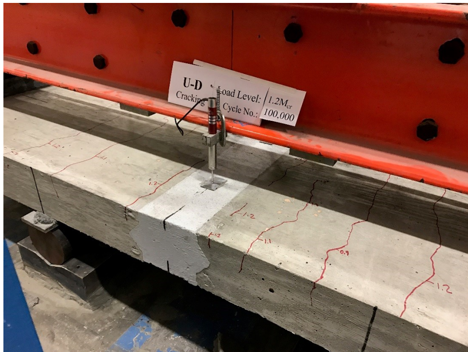
Figure 167. Photo. Observed cracking in specimen U-D after pre-cracking cyclic loading.
