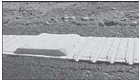
Figure 1. Photo. Raised profiled thermoplastic marking. (1)
