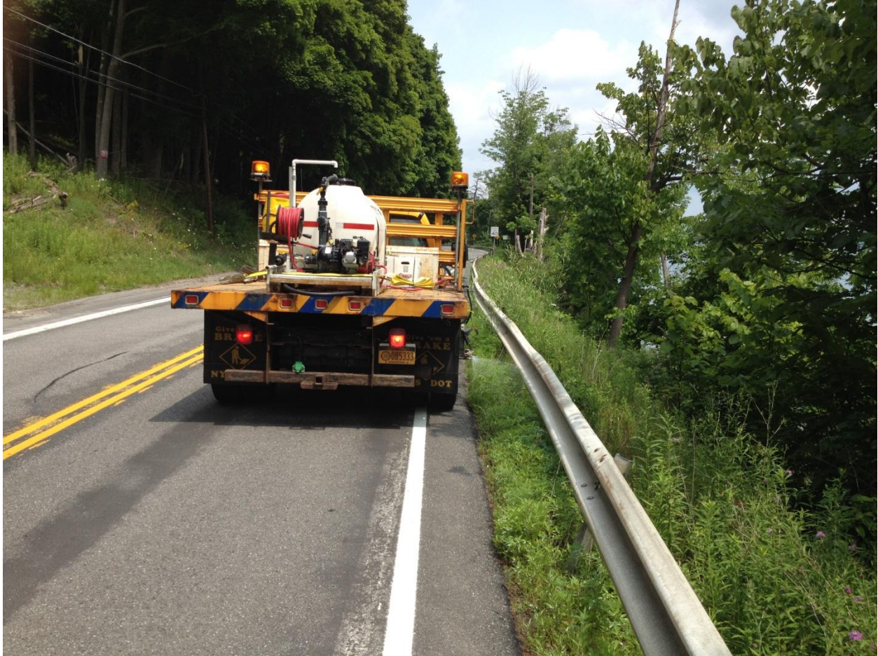
Figure 6. The NYSDOT spray operation as observed during the application of Scythe herbicide in the Route 80 corridor, July 22, 2014.
