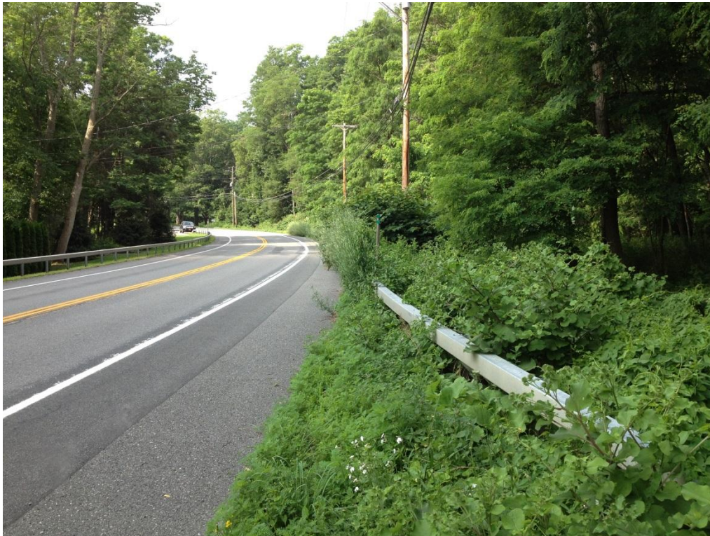
Figure 2. Photos of Route 80 alongside Otsego Lake (top) and just north of the Village of Cooperstown (bottom), Summer 2014.
