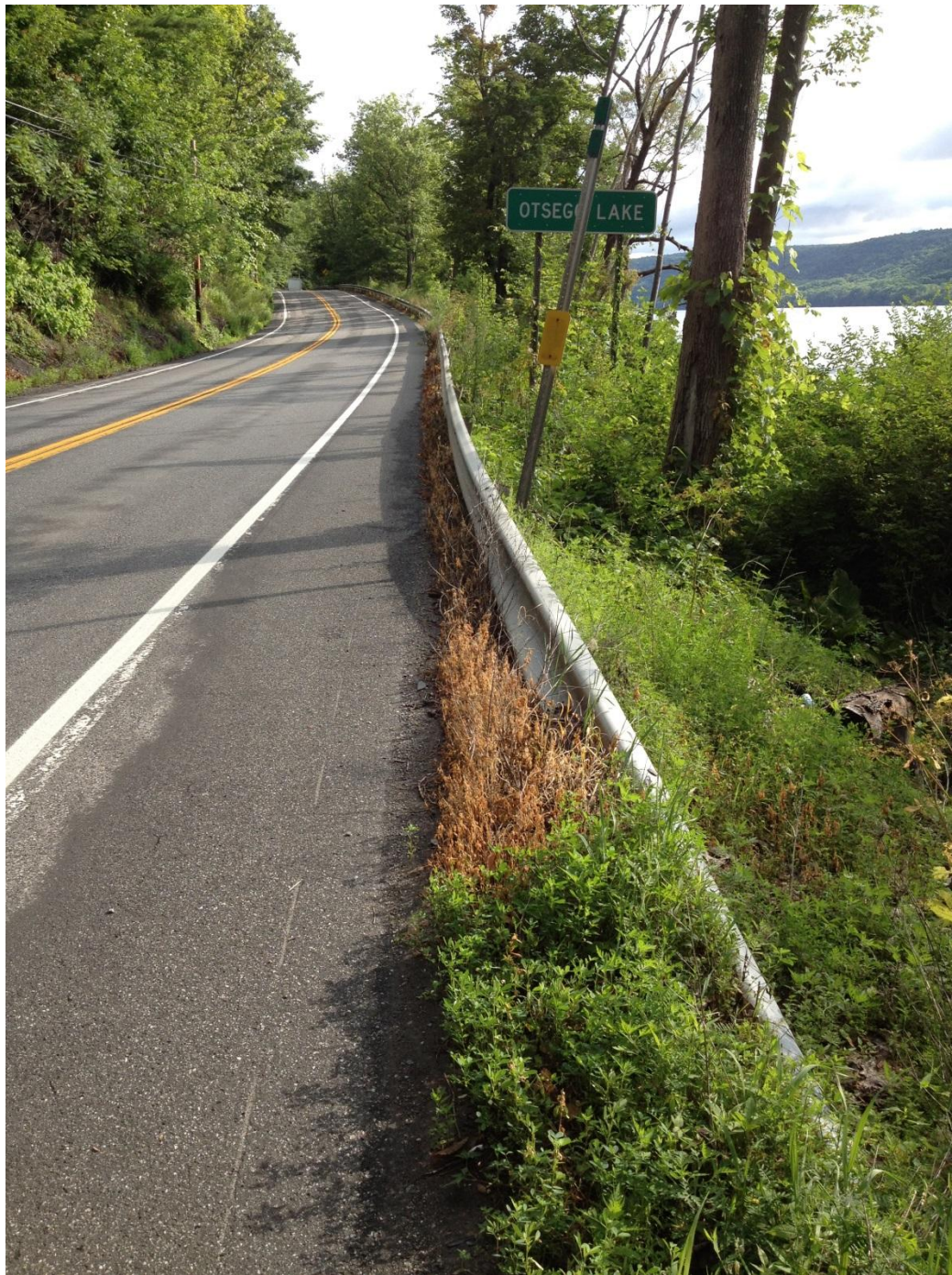
Figure 8. Plant damage as browned, necrotic tissue along the inside, western edge of guiderail, observed 5 days after treatment (July 27, 2014). Note that the Scythe herbicide was applied beginning ~5 feet north of the start of the guiderail.
