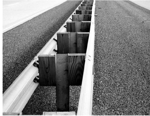
Fig. 1.3: A double-faced W-beam guardrail.
