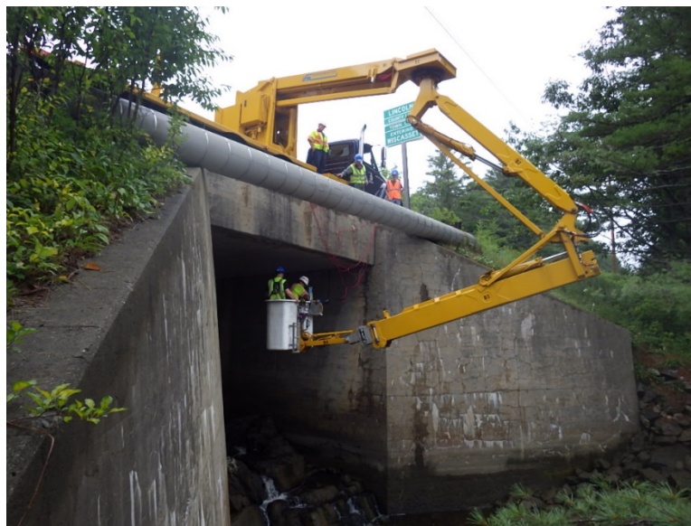
Figure 3: MaineDOT UBIT utilized to install sensors
