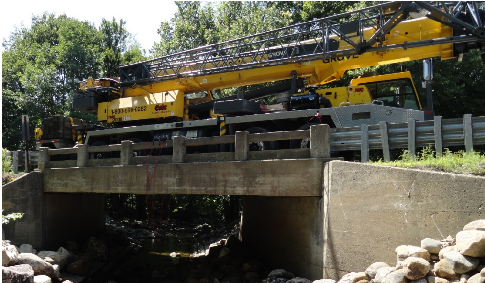
Figure 4: Grove TMS 900E crane used for bridge loading
