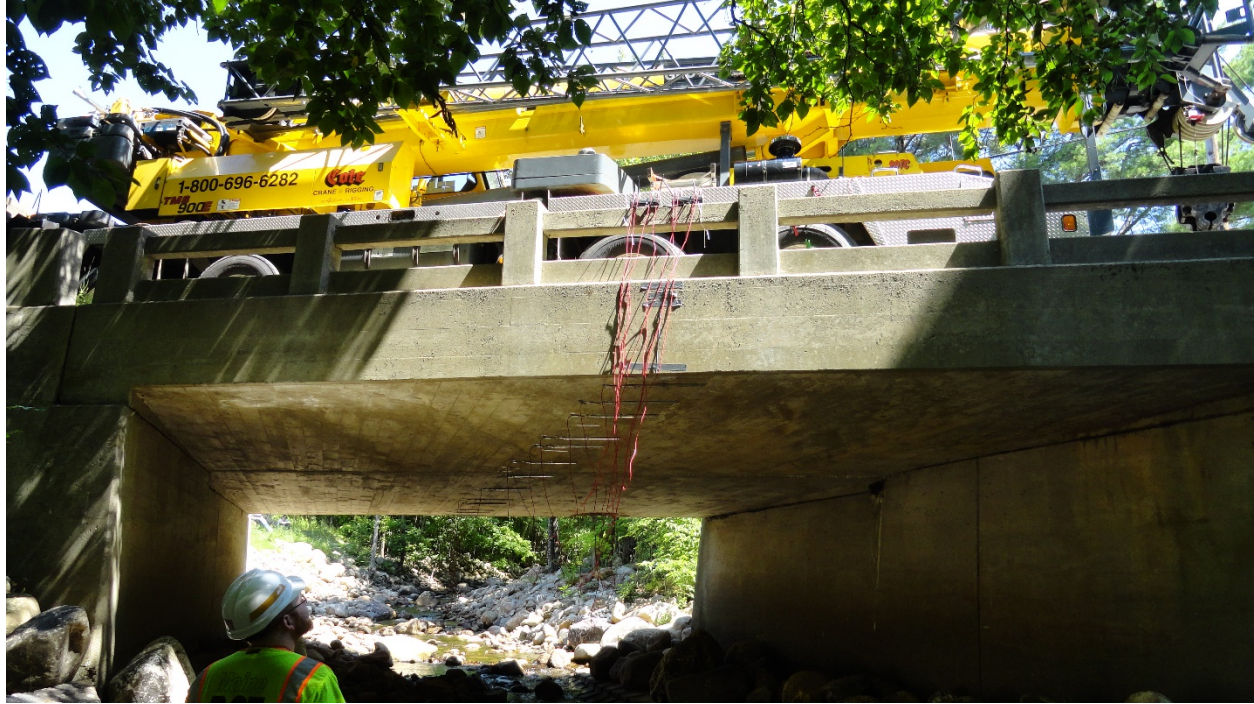
Figure 7: Weld No. 5361 general condition
