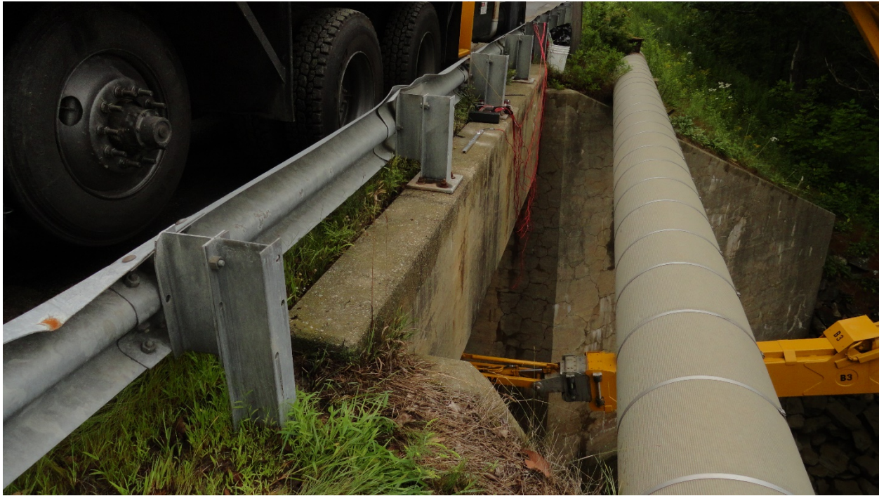
Figure 10: Woolwich No. 2577 showing integral curb and fill thickness
