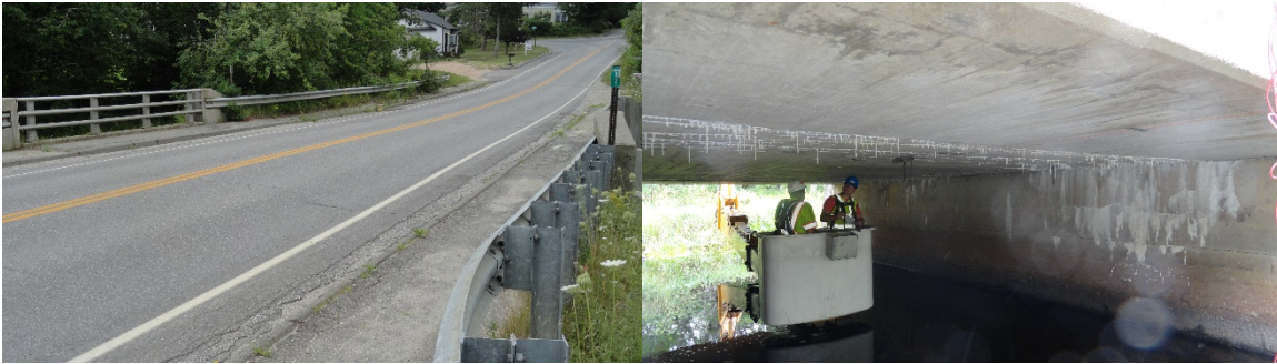
Figure 14: Penobscot No. 3297 overall configuration with sidewalks and new/ old/ new underneath
