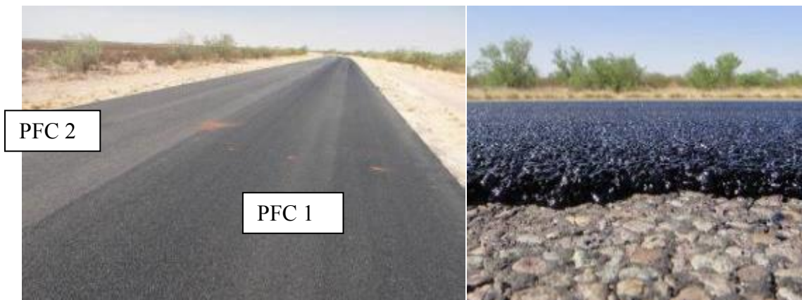
Figure 24. PFC Mix on Pecos Facility Entrance Road.
