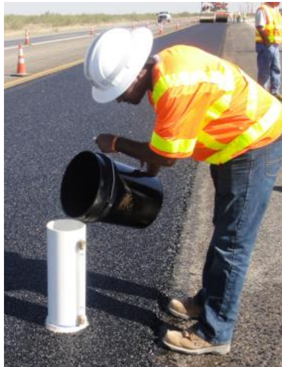
Figure 33. Water Flow Being Conducted on the New PFC.
