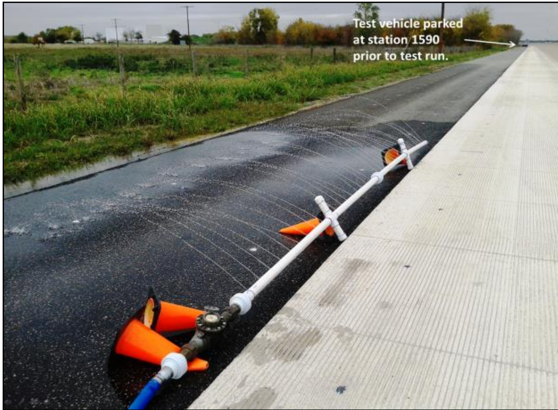
Figure 45. West Wheel Path Wetted prior to Test Run between Stations 555 and 575.
