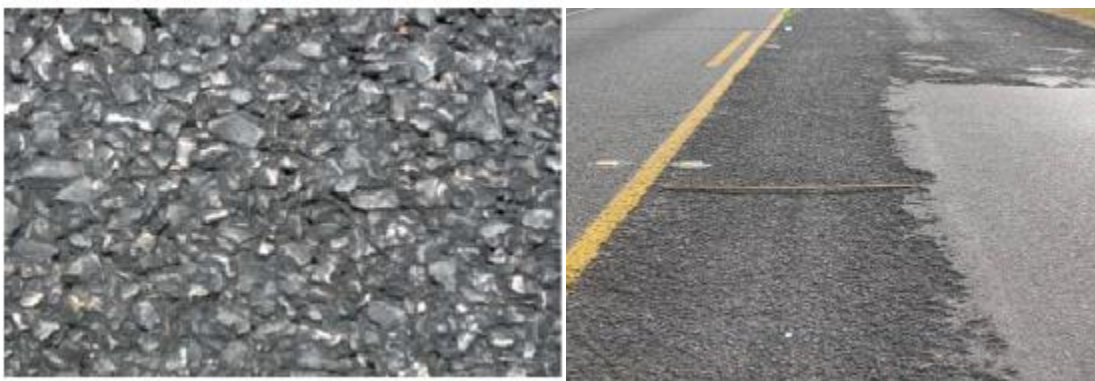
Figure 20. Nondraining and Raveling PFC Reported by Houston with AR PFC Binders.
