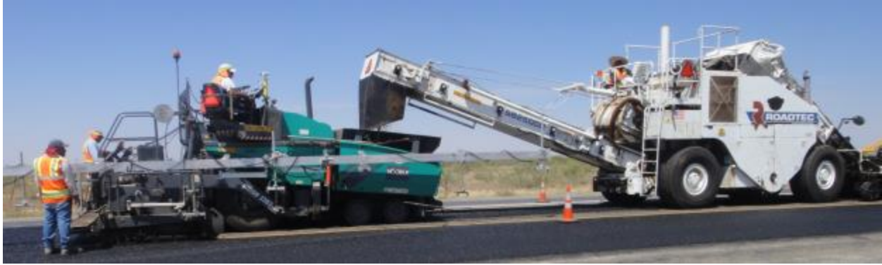
a) Belly dump trucks with RoadTec pickup
