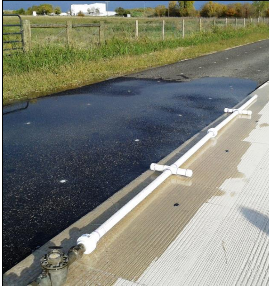
Figure 42. Test Setup between Stations 390 to 410.
