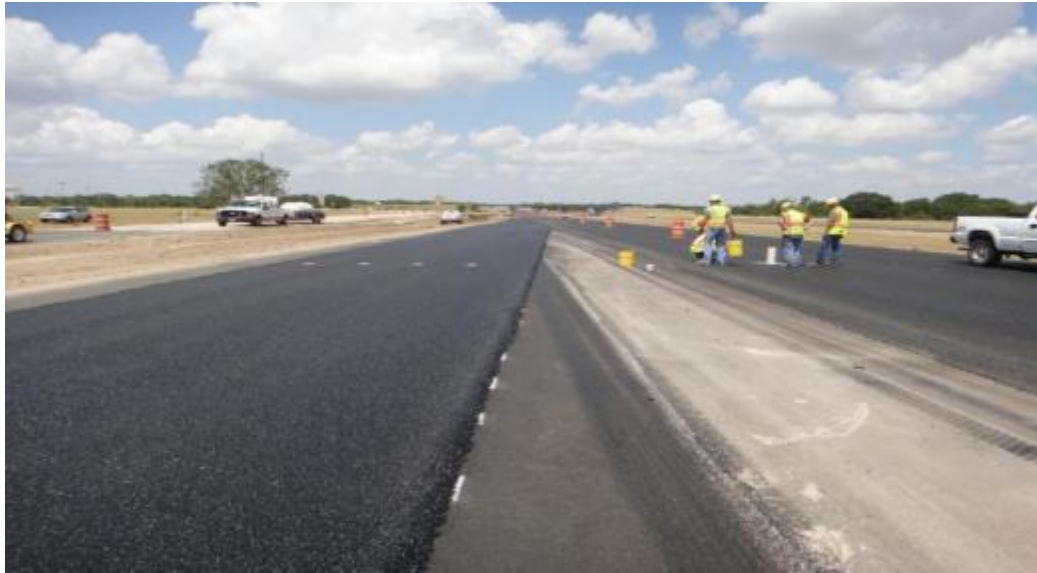
Figure 27. Construction of the Bryan Fine PFC Exit Ramp.
