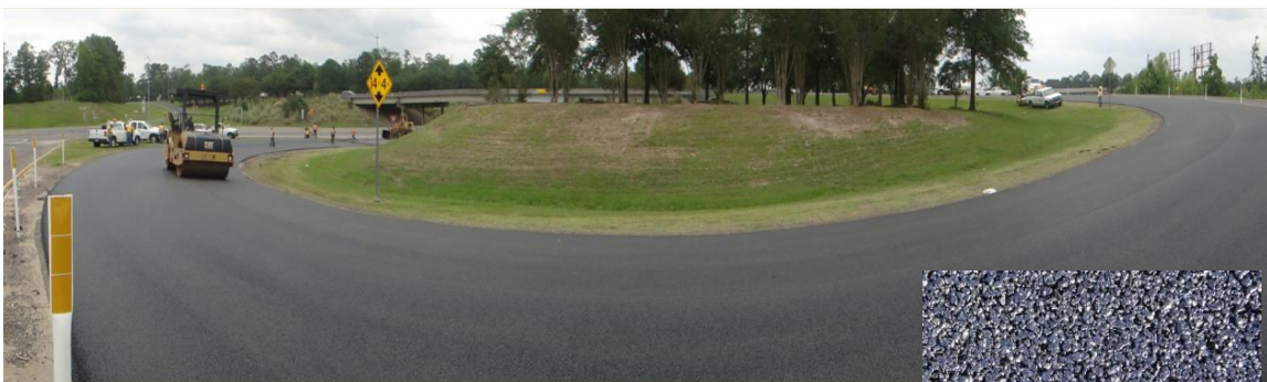
Very Thin, Fine-Graded PFC Placed on Cloverleaf Exit Ramp of US 59 Near Lufkin District Office. Maintenance needed a mix to address the numerous wet weather accidents occurring on this ramp.
