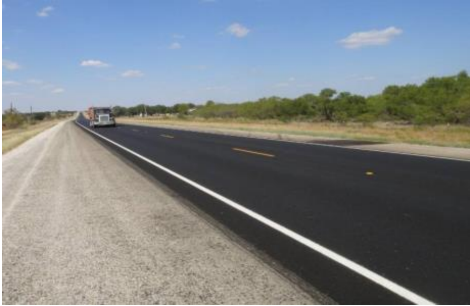
Figure 30. US 183 PFC Three Months after Construction.
