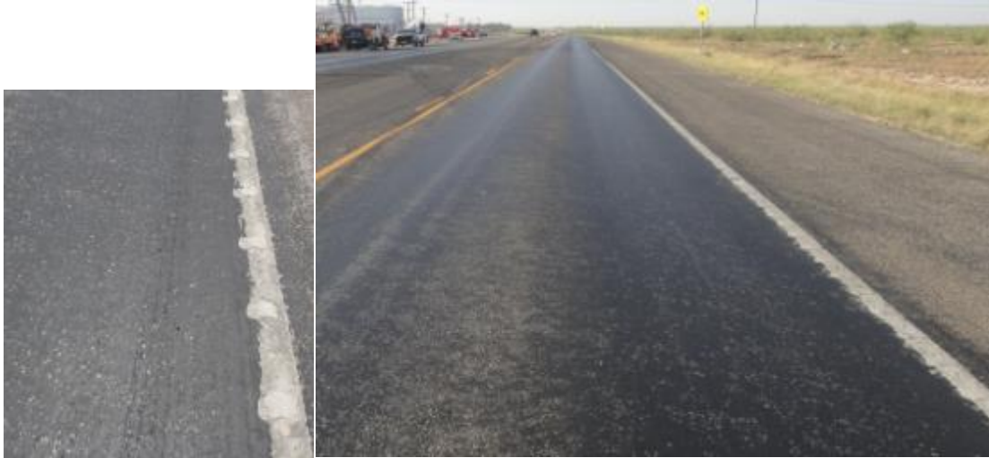
Figure 31. Preexisting Condition for Loop 338 Odessa District.
