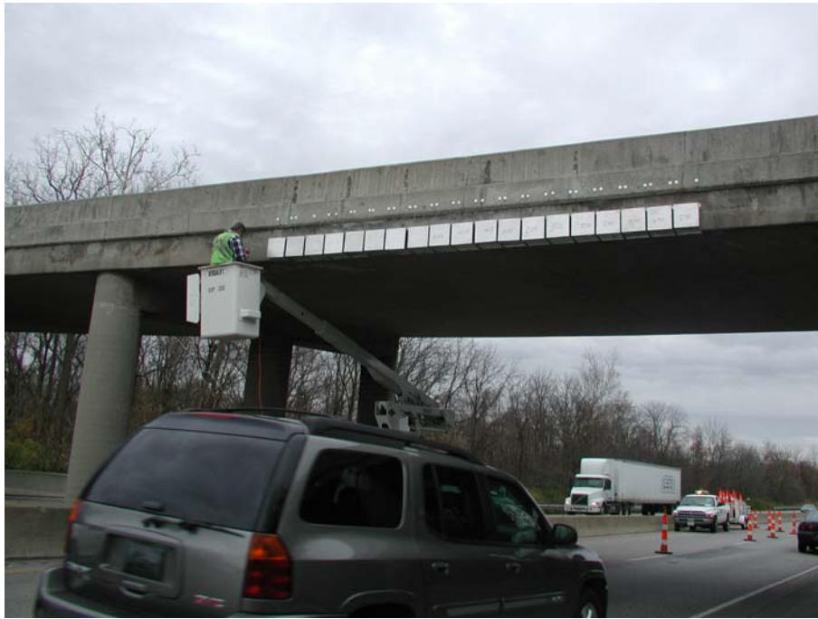
Figure 79 Final installed I-Lam panel on the bridge (DEL-23-12.99)
