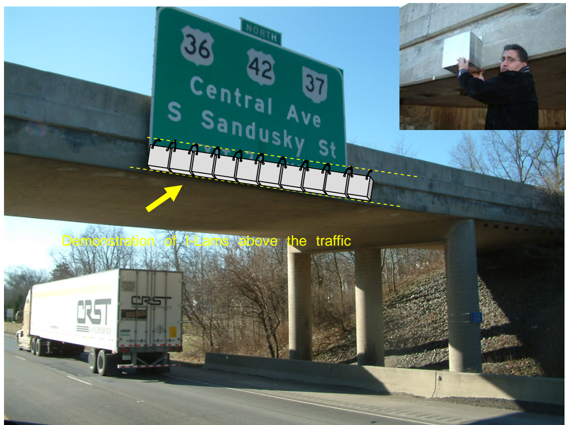
Figure 77 Schematic of I-Lam installation in DEL-23-12.00
