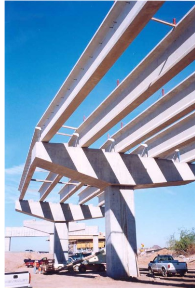
Figure 10. General view during construction of high occupancy vehicle (HOV) lanes (ADOT, 2001)
