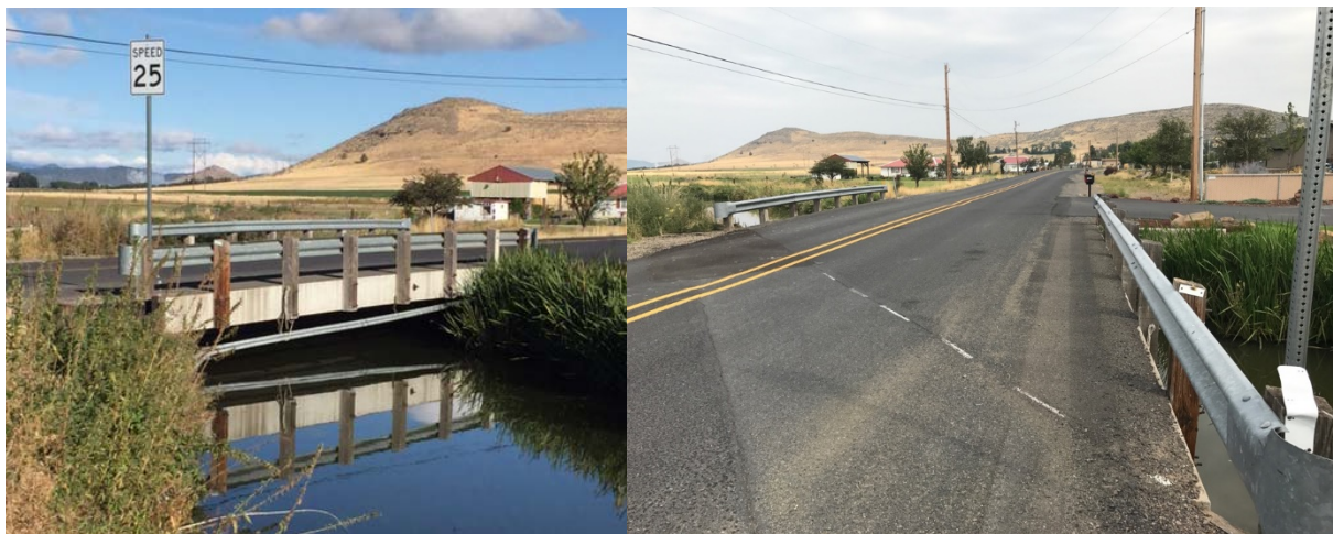
Figure 4.36: Elevation and northbound views of Washburn Way bridge.
