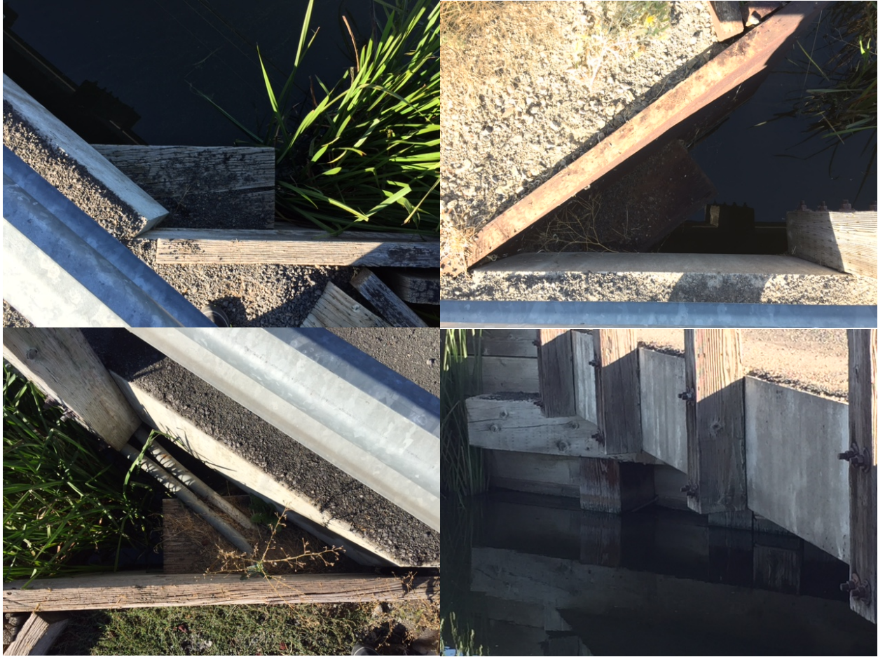
Figure 4.37: Views of timber pile abutments on Washburn Way bridge.
