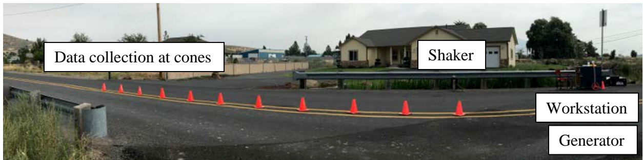
Figure 4.35: Test setup on Washburn Way bridge.
