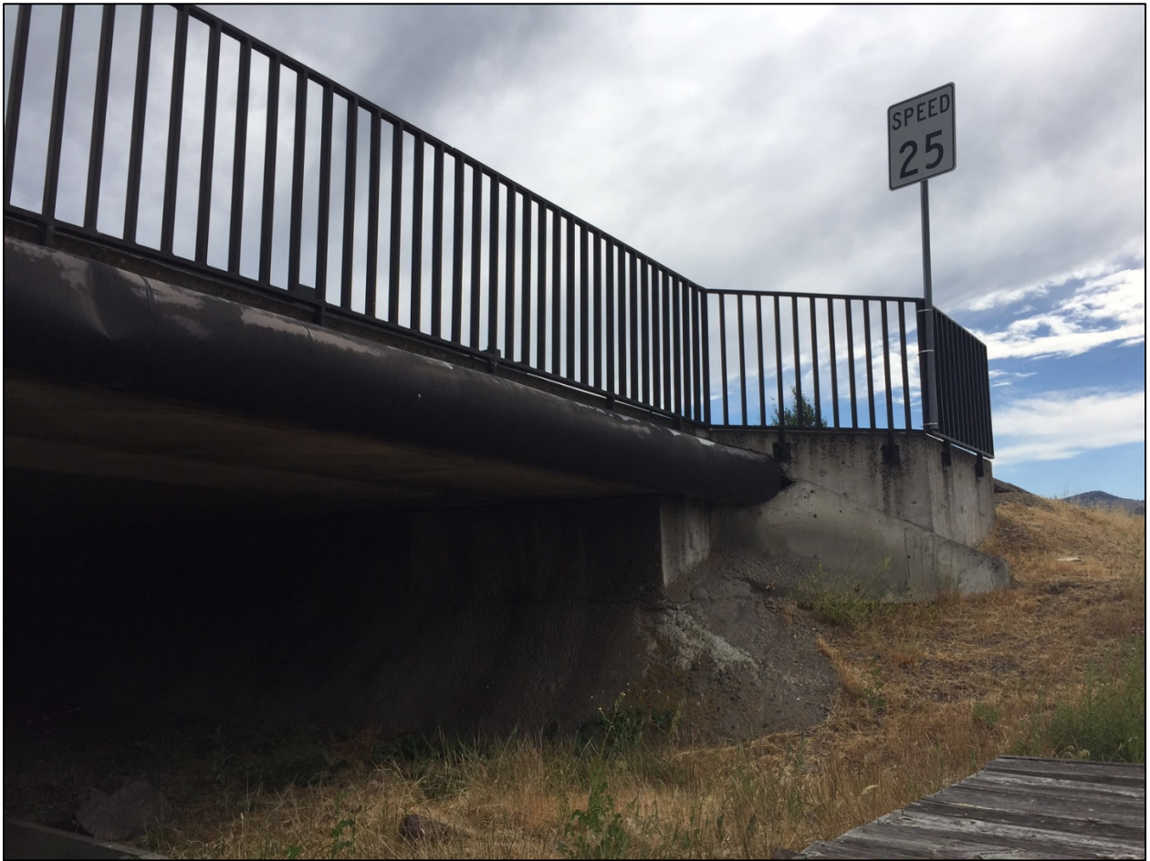
Figure 4.29: Northwest abutment of Harbor Isles Boulevard bridge.
