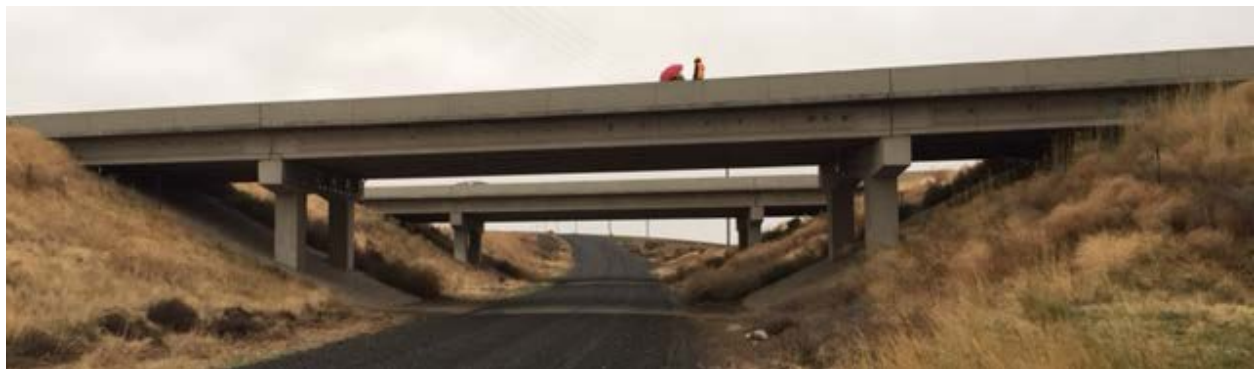
Figure 4.41: Elevation view of I-84 WB bridge looking south.
