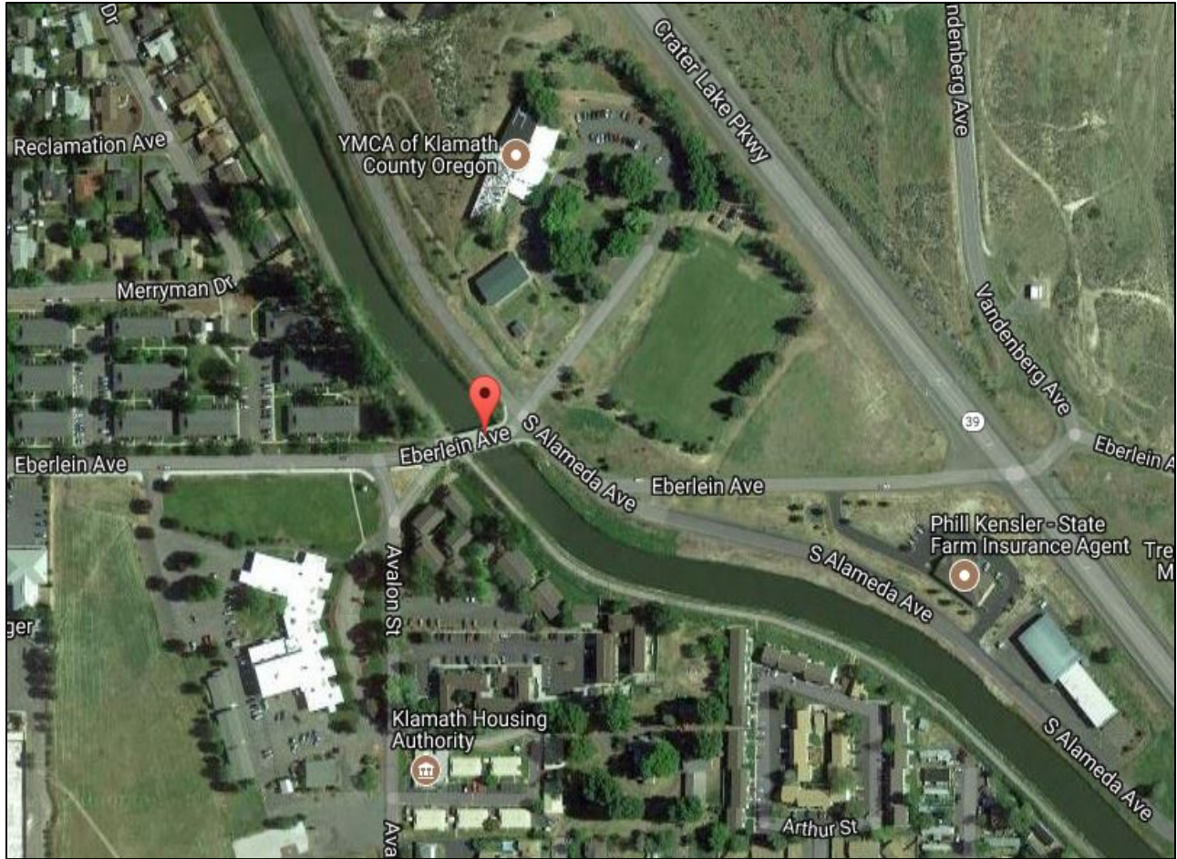
Figure 4.8: Vicinity of Eberlein Avenue bridge
