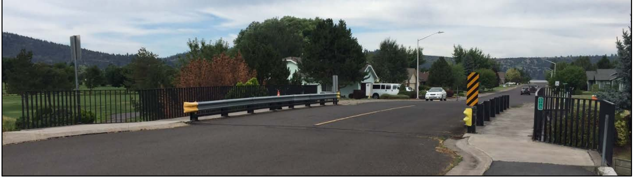
Figure 4.28: Harbor Isles Boulevard bridge looking west.
