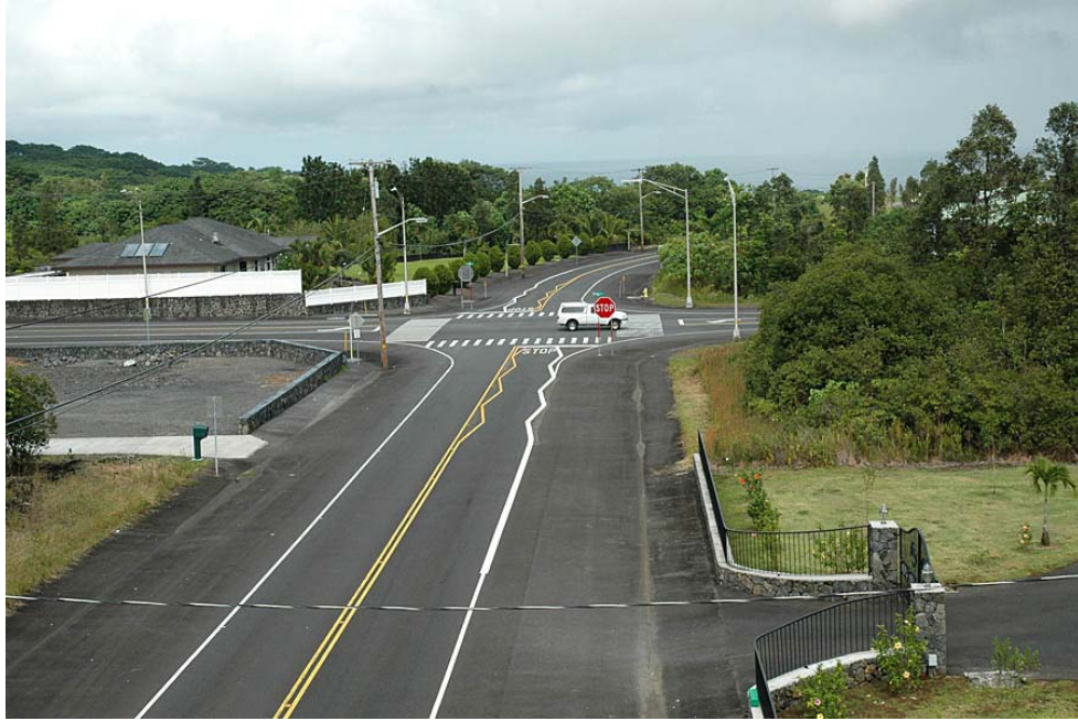
Figure 15. Zig-zag Pavement Markings at Intersection of Wilder and Puainako in Hawaii. From Ron Thiel. Reprinted with permission.
