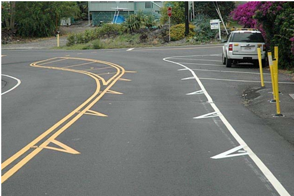
Figure 14. Shark's Teeth Pavement Markings Installed in Hawaii. From Ron Thiel. Reprinted with permission.
