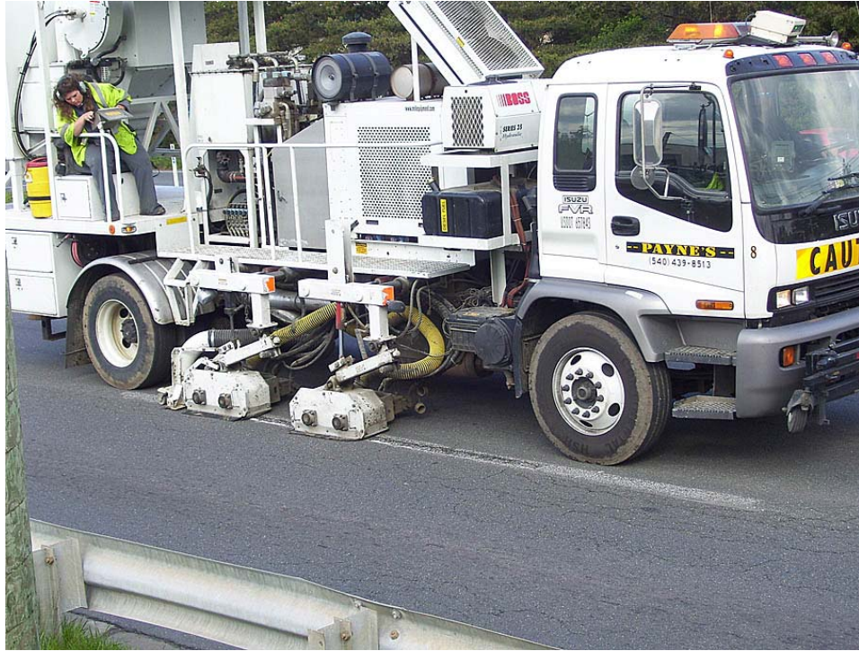
Figure D-3. Eradication of Skip-Lines on Sterling Boulevard
