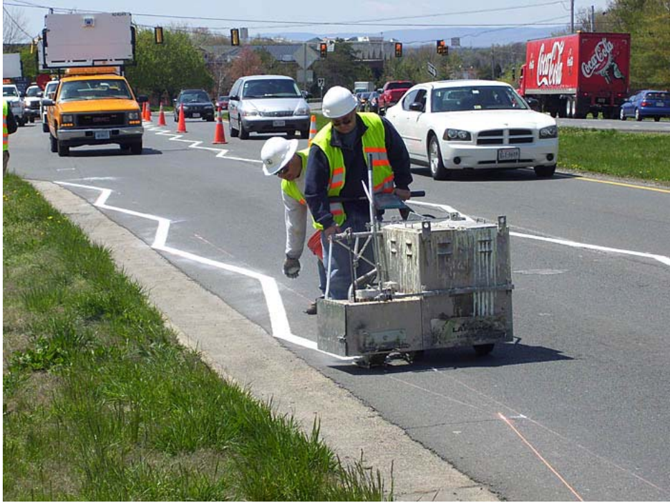
Figure D-5. Marking Painting on Eastbound Approach of Sterling Boulevard
