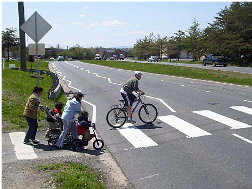
Figure 11. Zig-zag Markings on Eastbound Approach at Sterling Boulevard
