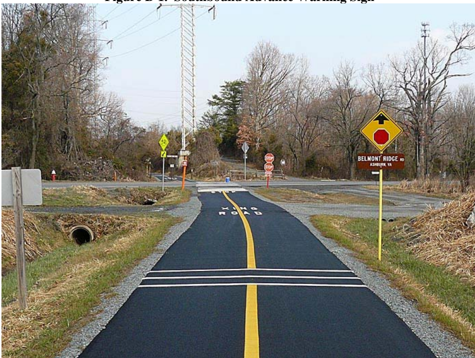
Figure B-2. W&OD Trail Signage and Pavement Markings
