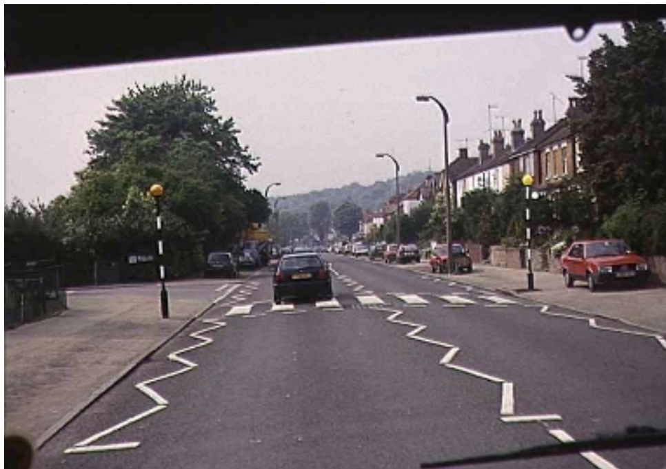
Figure 1. Zig-zag Pavement Markings in England Observed by U.S. Traffic Engineers. From Scott Wainwright.
