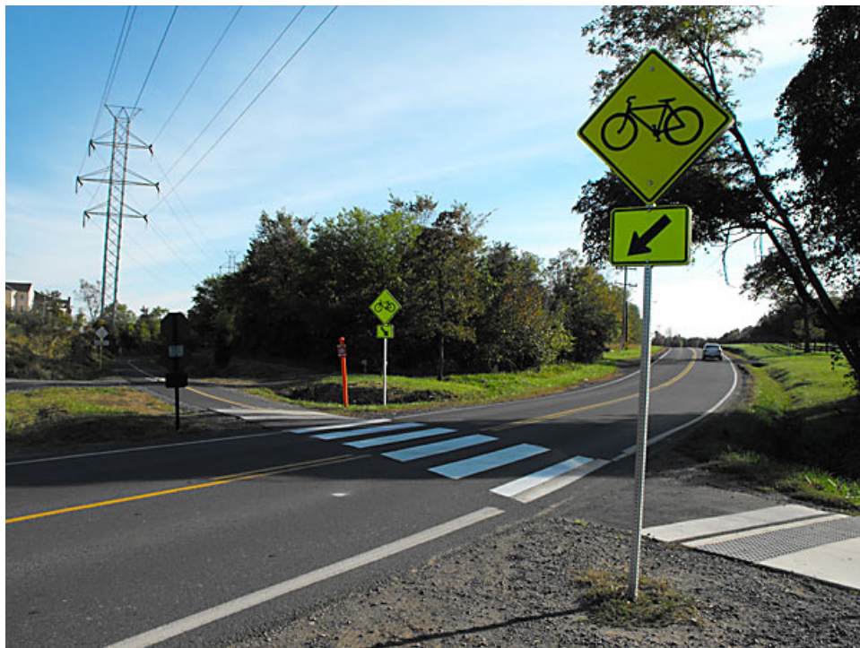
Figure 3. Trail Warning Signs at Belmont Ridge Road W&OD Crossing
