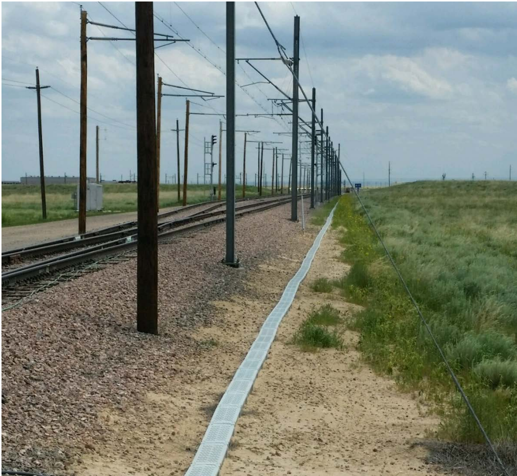
Figure 4. Cable Management System
