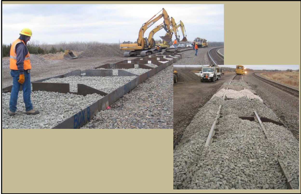
Figure 13. Installation of the UP Ballast Box Test
