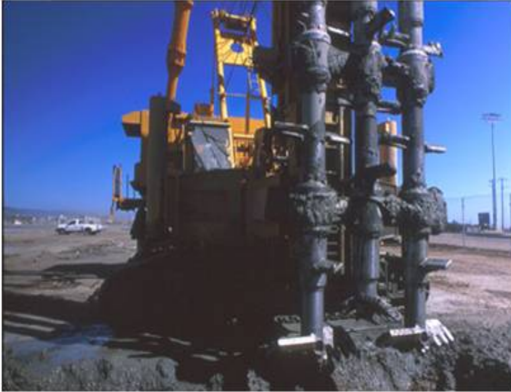
Figure 143. Photo. WRE mixing equipment.
