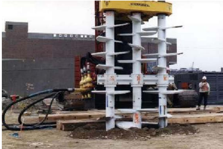
Figure 140. Photo. Typical blade-based tooling for WRS mixing. (127)
