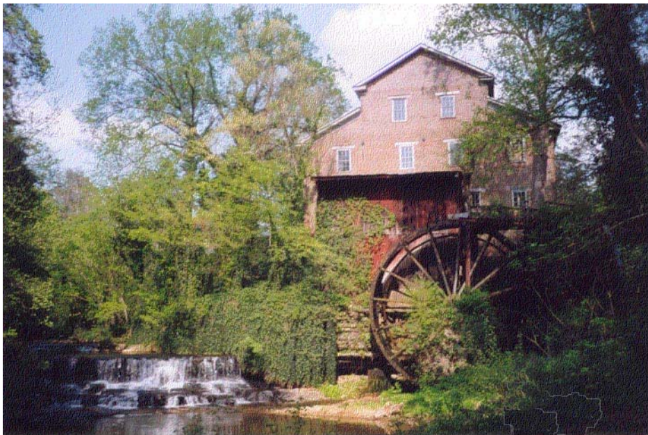
Figure 22. Falls Mill is spared from floods by its position high on a natural bluff.
