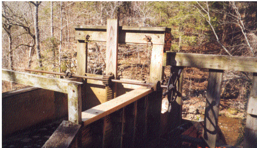
Figure 32. The wheel gate at Falls Mill in Franklin County, Tennessee.
