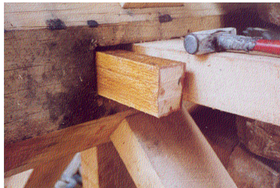
Figure 54. Wedges were driven into the axle mortises to secure the spokes.
