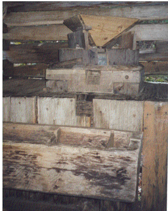
Figure 37. Primitive millstones, platform, and meal box inside Ogle Tub Mill.
