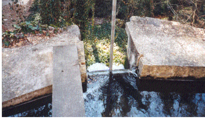
Figure 33. Spillway plug at Falls Mill in Franklin County, Tennessee.
