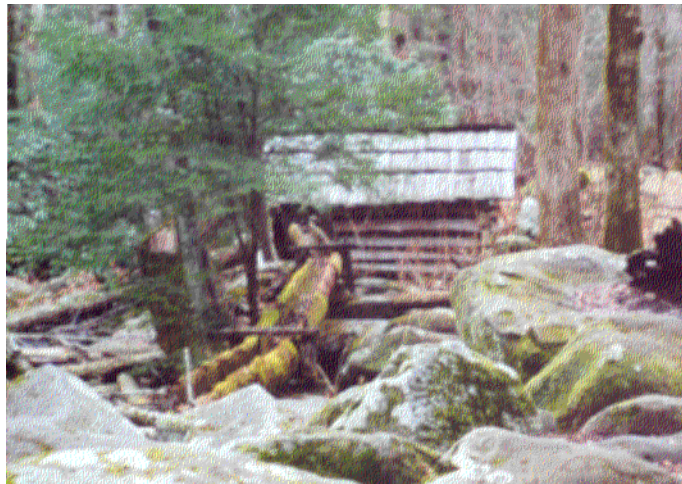
Figure 30. Flume of hollowed logs leading to the tub wheel at Ogle Mill.
