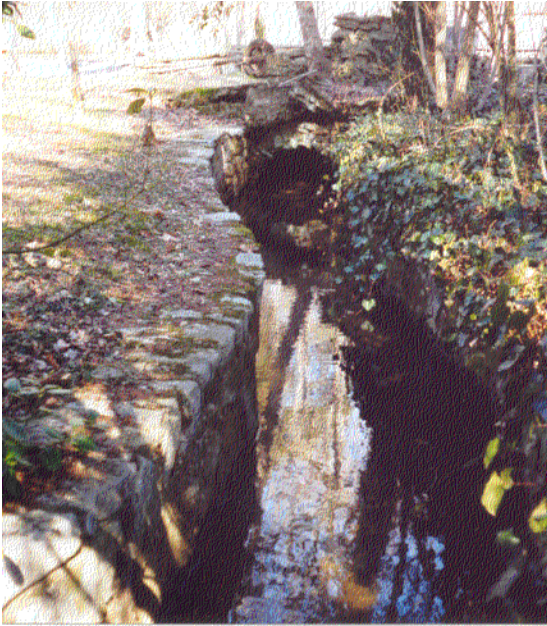
Figure 29. Examples of dug and elevated millraces, Falls Mill and Evins Mill.
