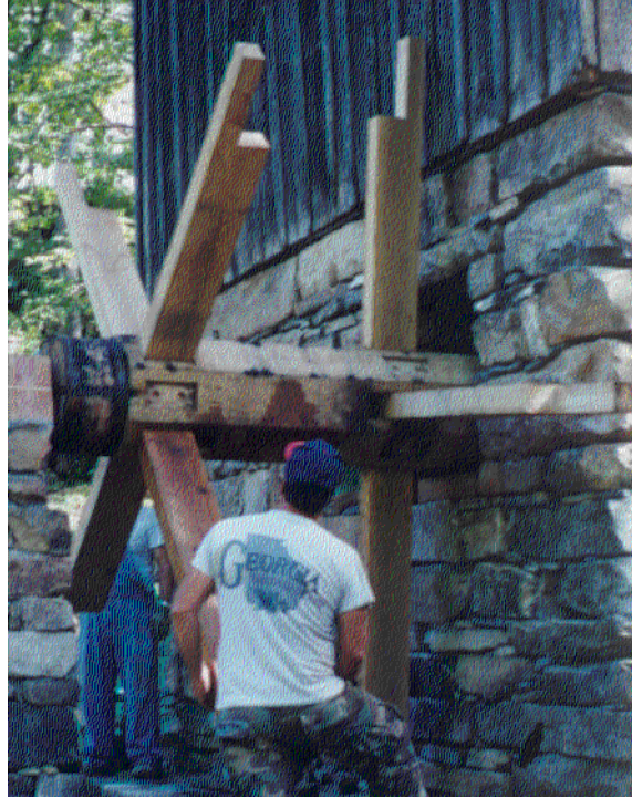
Figure 53. Installing the spokes into the mortise holes in the axle.
