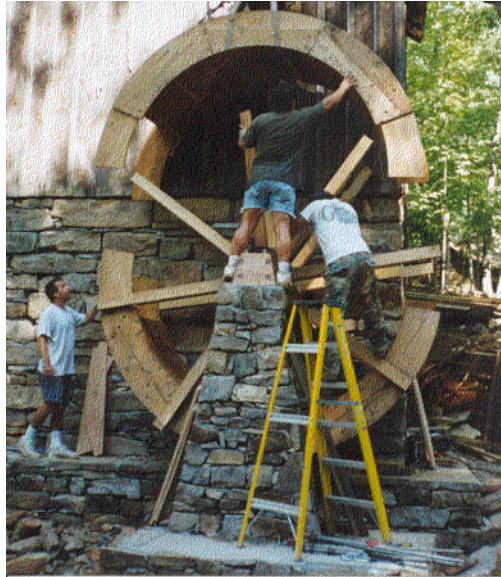
Figure 55. Attaching sections of a wooden water wheel built in two parts.
