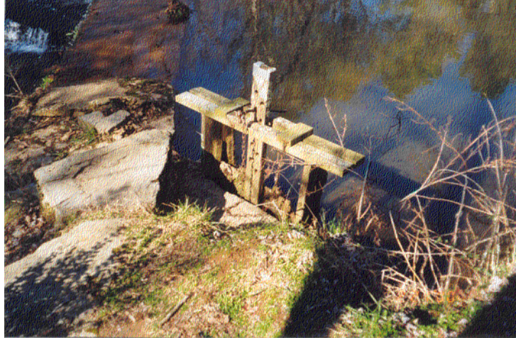
Figure 31. The head gate at Falls Mill in Franklin County, Tennessee.
