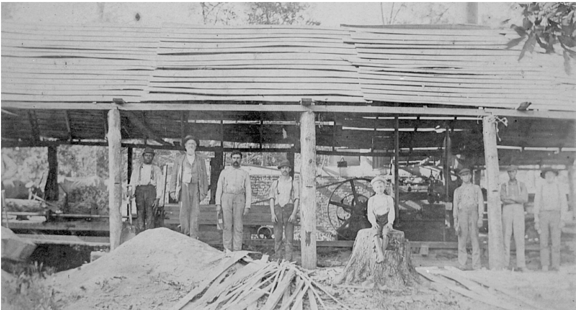
Figure 129. Calvin Sweeney's steam sawmill in Henry County, Tennessee, ca. 1900. Mr. Sweeney is second from left. The stationary steam engine is in the right background.
