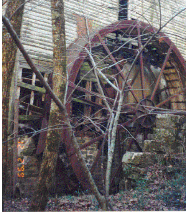
Figure 144. Savage Company water wheel on the Virtue Creek Mill in Knox County, Tennessee. This wheel is unusual in that it has two pinion gear drives off the same wheel.
