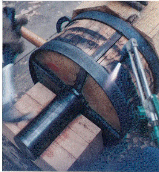
Figure 47. Securing the gudgeon by shrink fitting iron bands onto the axle.
