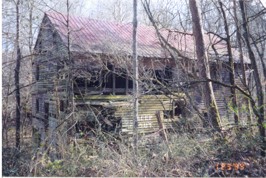
Figure 63. Massengill Mill in Grainger County, Tennessee, before its move.
