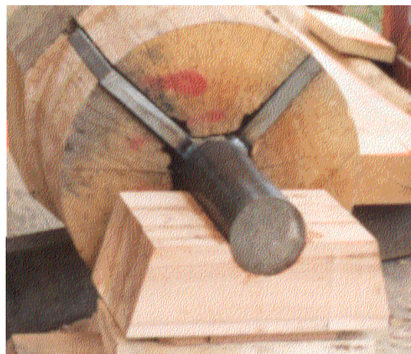
Figure 112. A hard maple shaft bearing, with cap removed.
