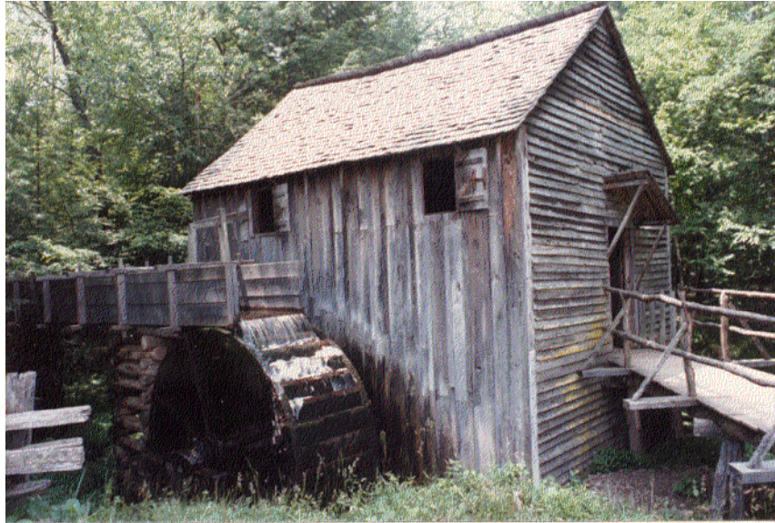
Figure 43. Overshot water wheel of John Cable Mill, Great Smoky Mountains.
