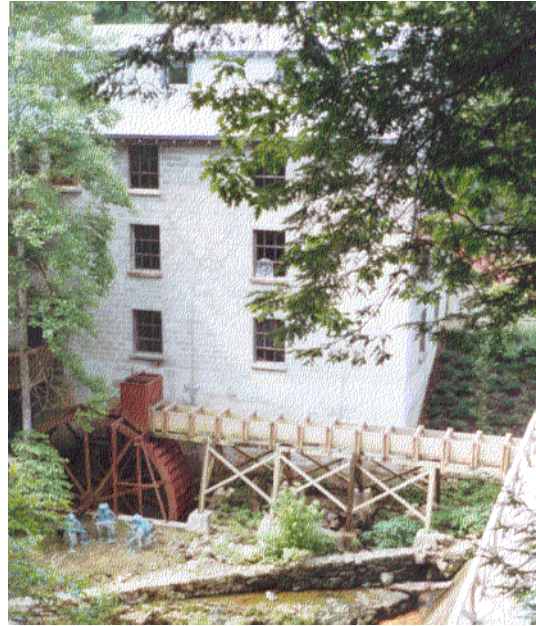
Figure 29. Examples of dug and elevated millraces, Falls Mill and Evins Mill.
