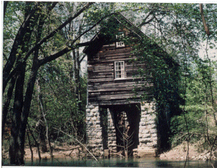
Figure 23. Lower Mill in Hamilton County, Tennessee, situated on high rock piers.
