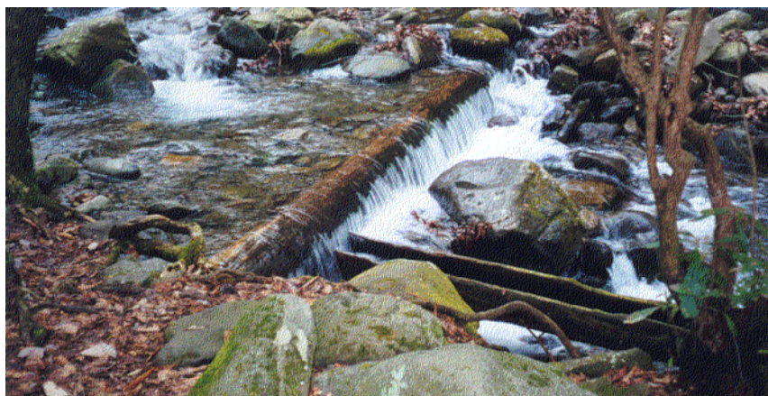
Figure 17. Log water diversion and beginning of wooden trough flume to mill.
