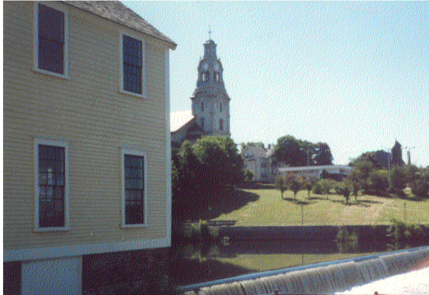
Figure 7. Samuel Slater's cotton mill and dam in Pawtucket, Rhode Island.
