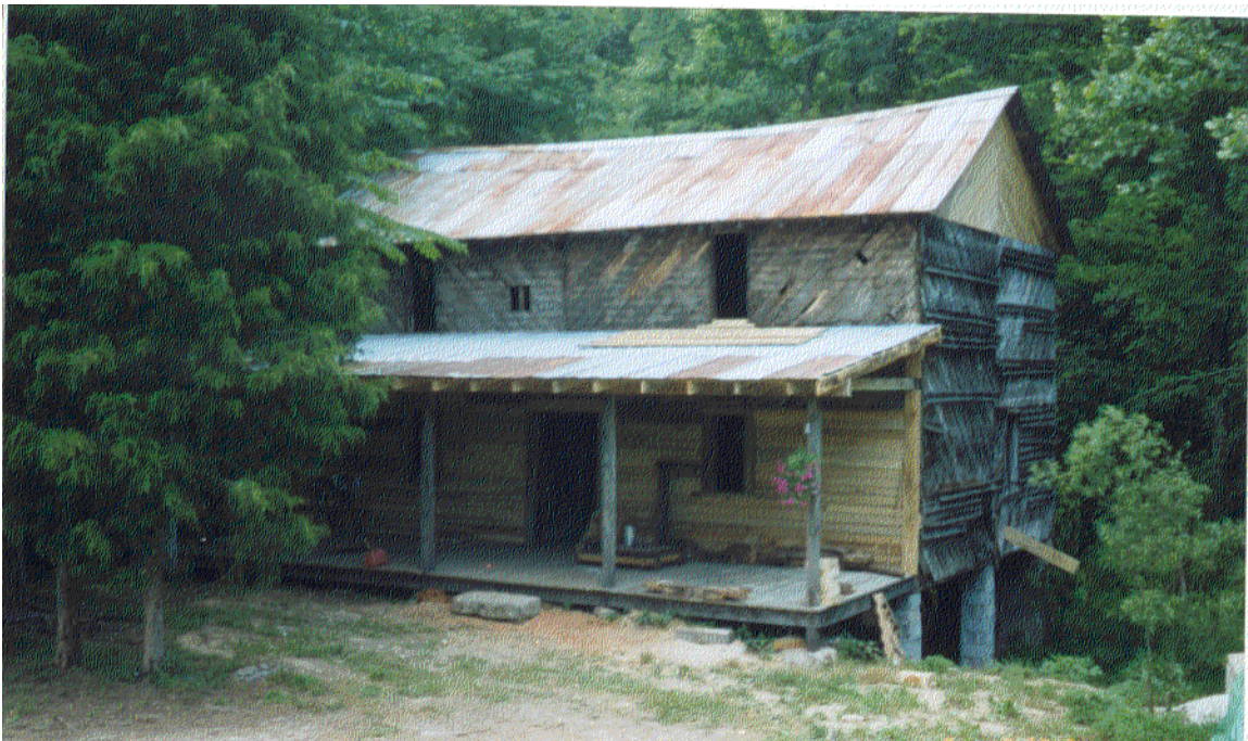
Figure 152. Old Spencer Mill returned to its original location.
