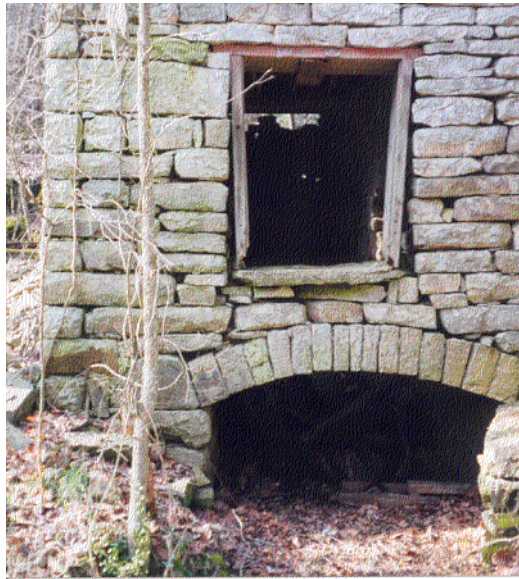
Figure 64. Original enclosed wheel room at Massengill Mill, showing tailrace arch.
