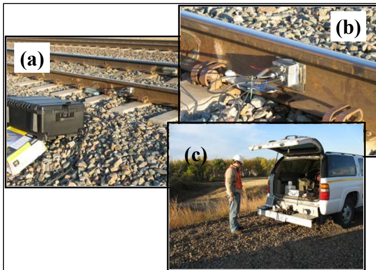
Figure 44. Portable Ultrasonic System Operated from a Rail Vehicle Next to the Testing Locations
