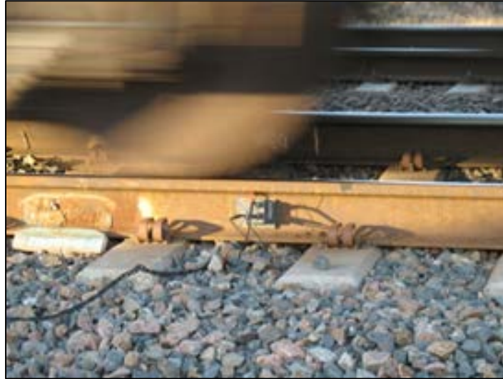
Figure 45. Ultrasonic Transducers Attached to the Web of the Rail, Remaining in Place While the UP Track Was in Service
