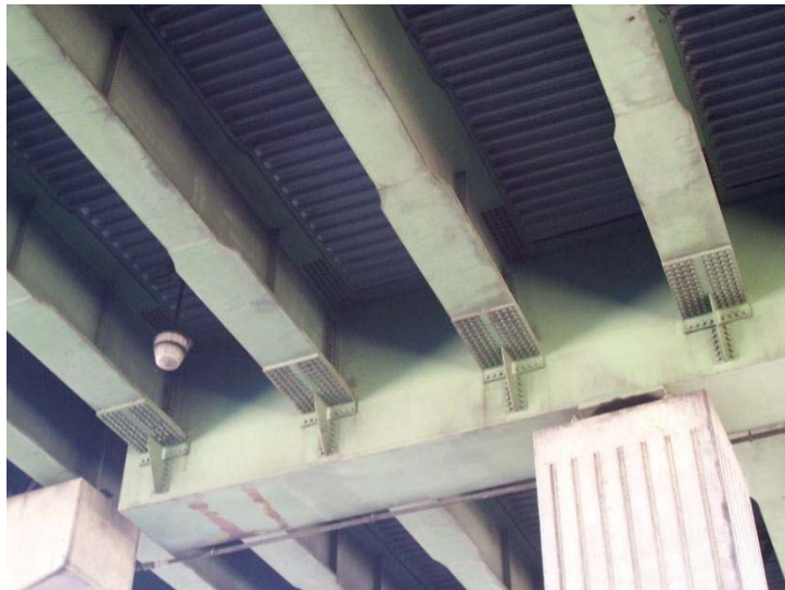
Figure 2: Close-up view of the girder to cross girder connection.
