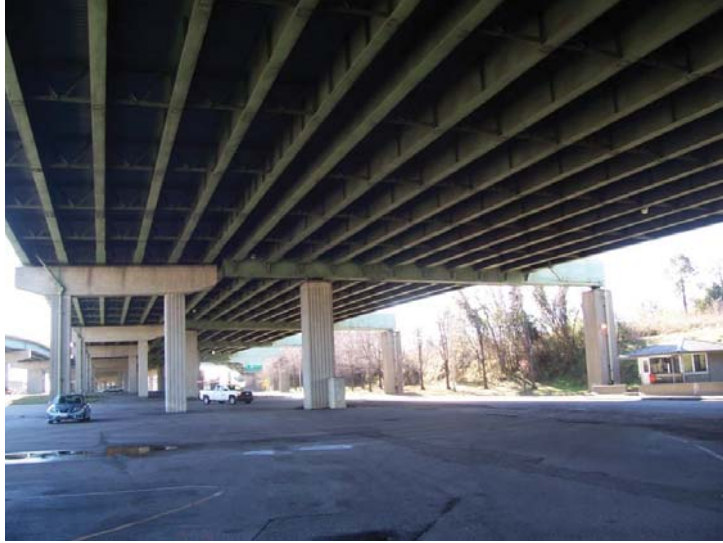
Figure 1: General view of the I-664 bridge crossing over Terminal Ave. in Newport News, VA.
