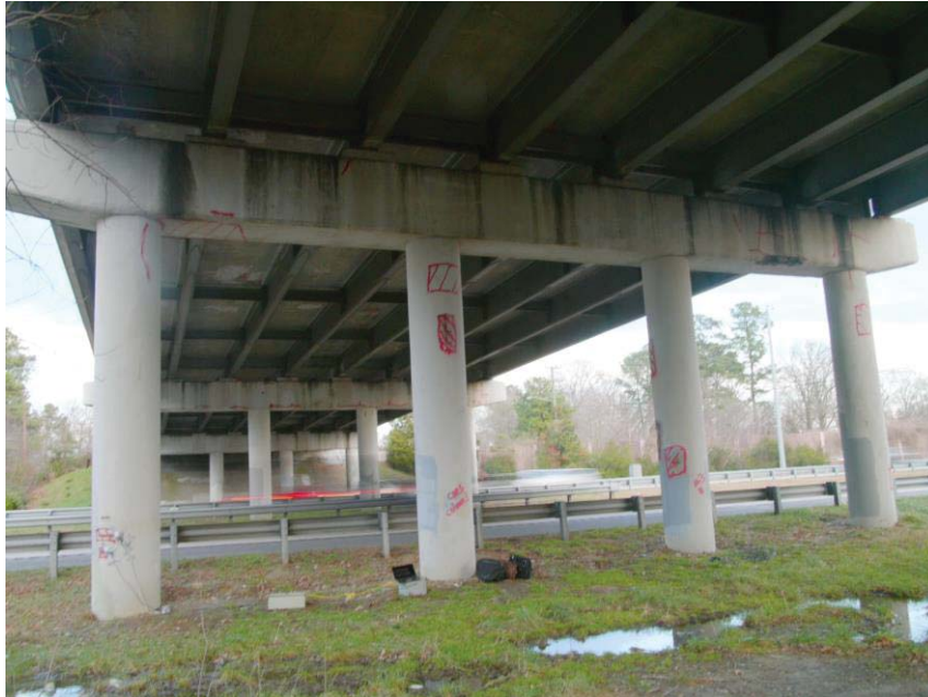
Figure 2: Concrete columns of Denbigh Boulevard Bridge affected by corrosion. Pieces of concrete fallen off from the column are shown in figure 3.
