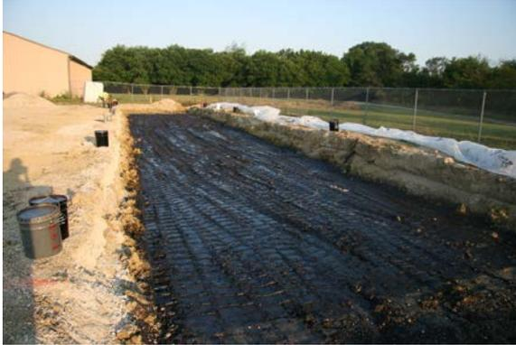
Subgrade Surface after Application of Tack Coat
