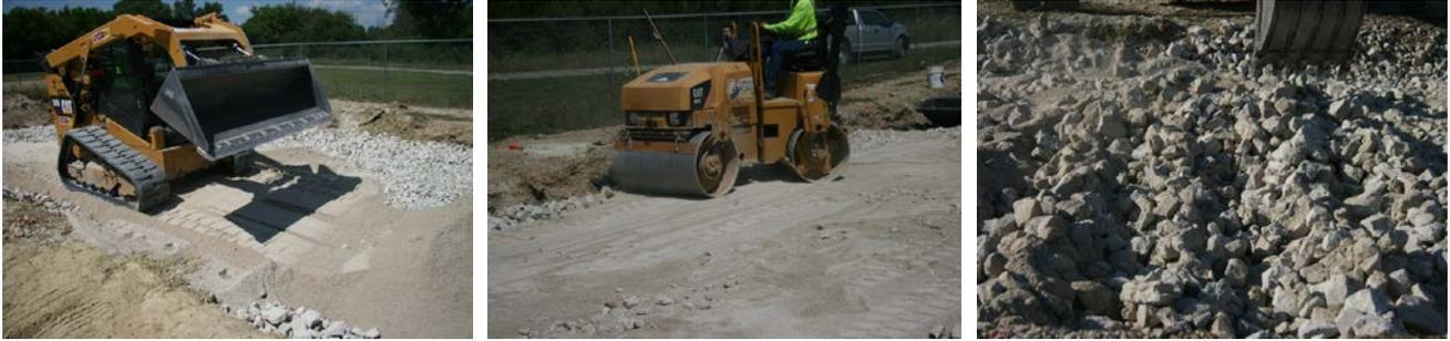
Construction of the first lift in the two-lift PCR/QB1 test section (C1S1)
