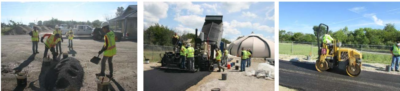
Figure 4.15. Hot mix asphalt sampling and paving.
