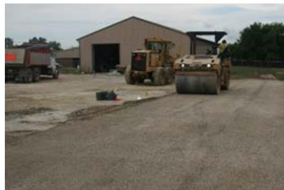
Placement of CA06\_R Capping layer for Cell 1
