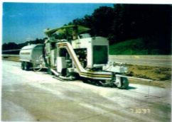
Photo #1 Machine used for Diamond Grinding
