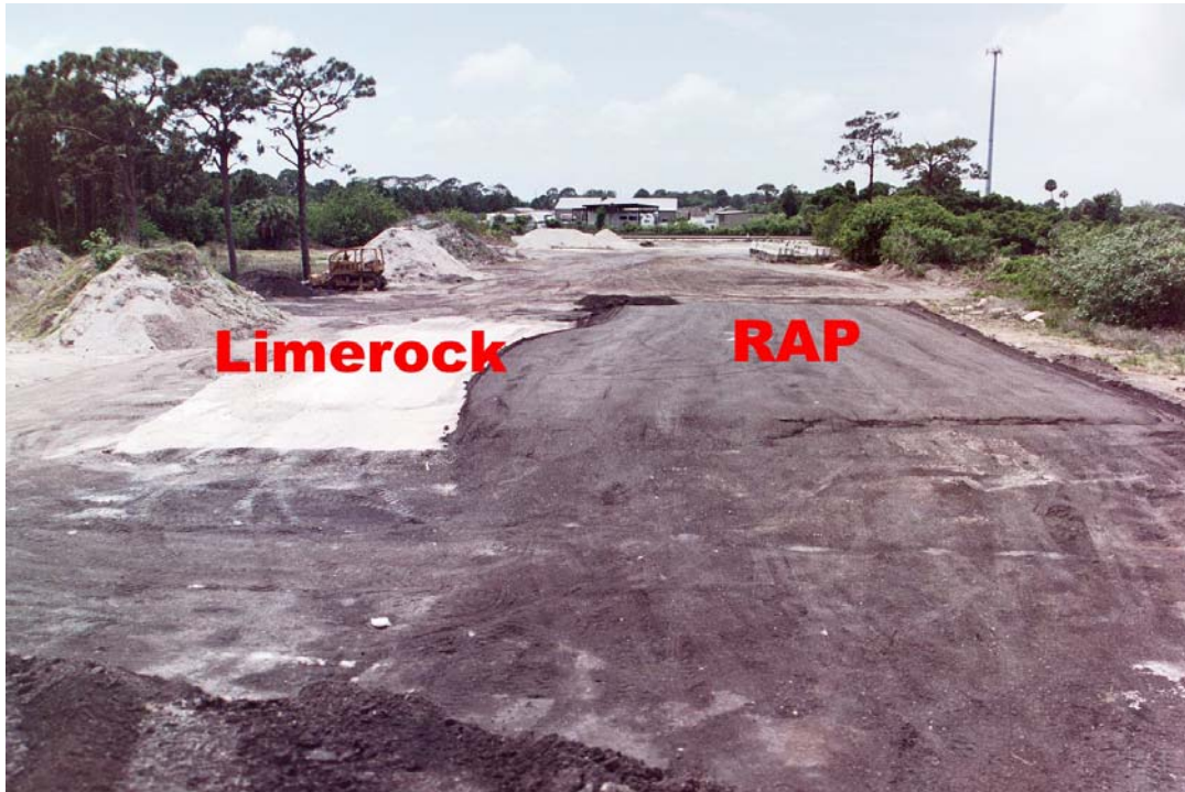
Figure 3.4 Completed Highway Materials Test Field Site
