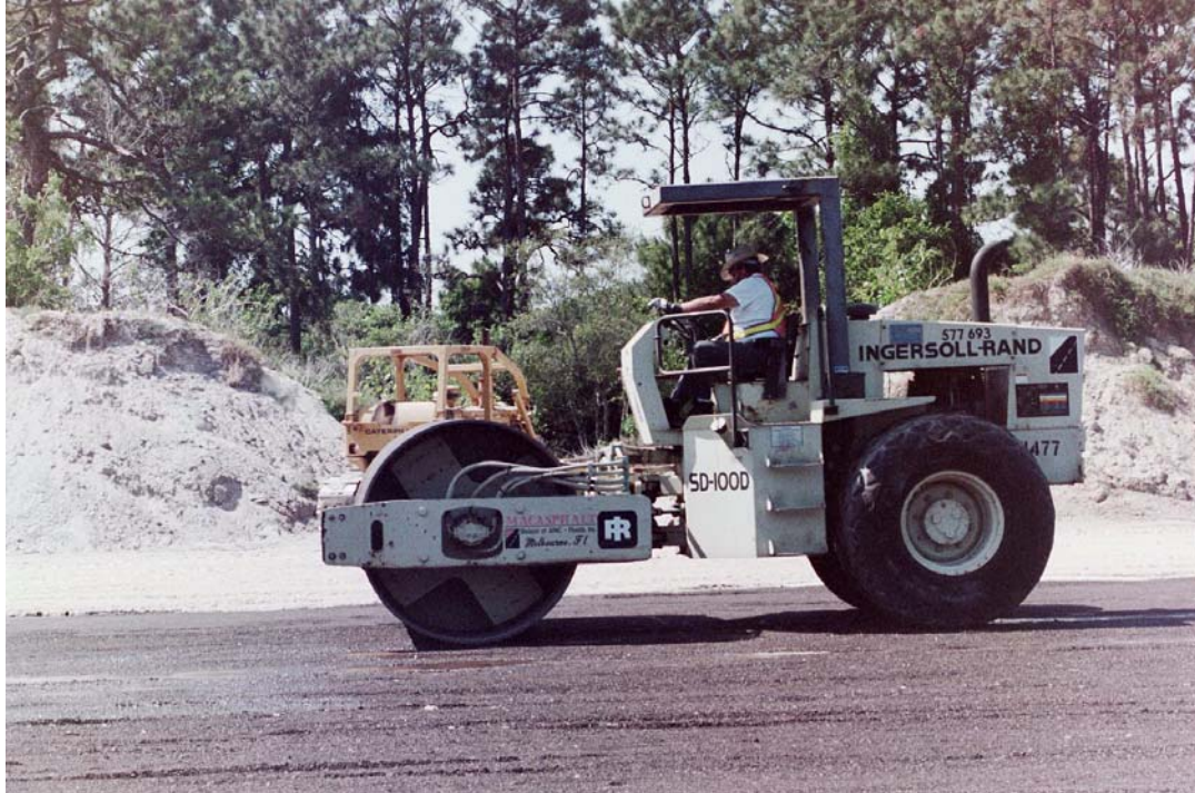
Figure 3.3 Vibratory Compaction of 1 st Lift
