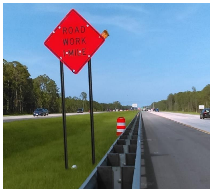
Figure 3-7. iCone #2 at “ROAD WORK 1 MILE” Sign
