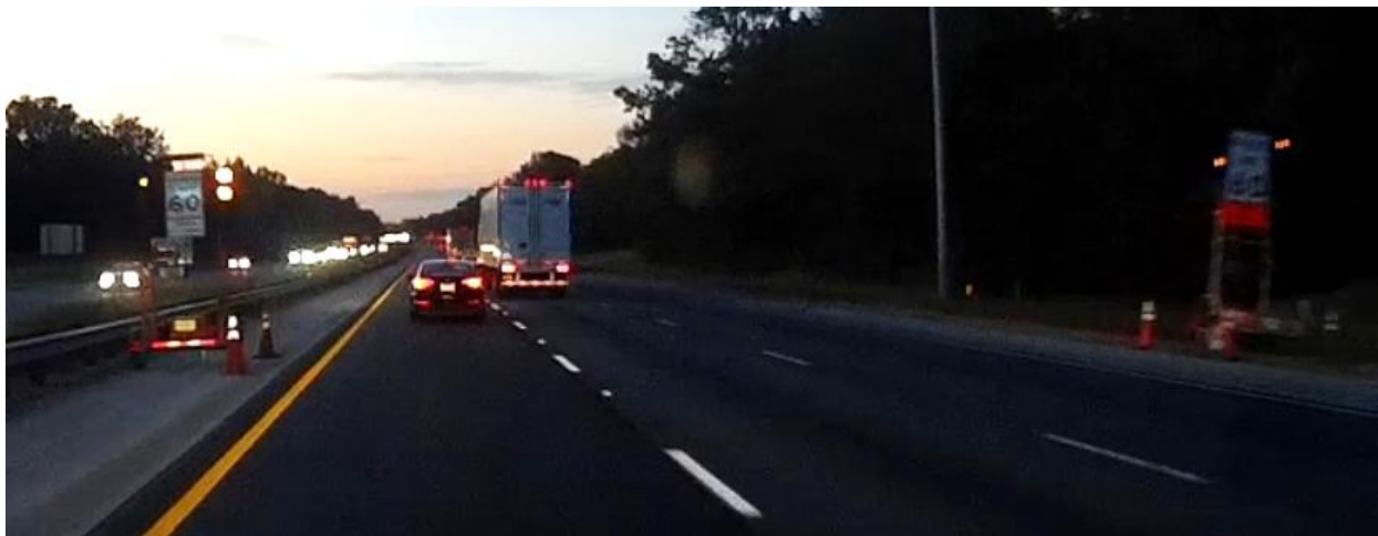
Figure 4-3. Reduced Work Zone Speed Limit Warning Sign
