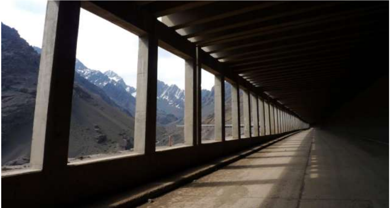
Figure 26. Inside an avalanche shed in the mountains of Chile. Note the impressive total length of avalanche shed at this site.
