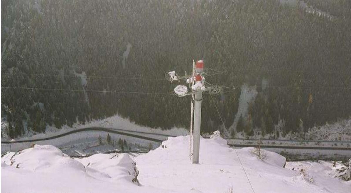
Figure 4. A light cableway or ‘bomb-tram’, (cable for transporting explosives, CATEX®), for delivering avalanche control explosives to the avalanche starting zone where they can be detonated remotely.
