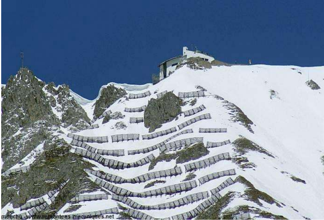
Figure 23. The extent of a typical deployment of snow supporting structures in the Alps.
