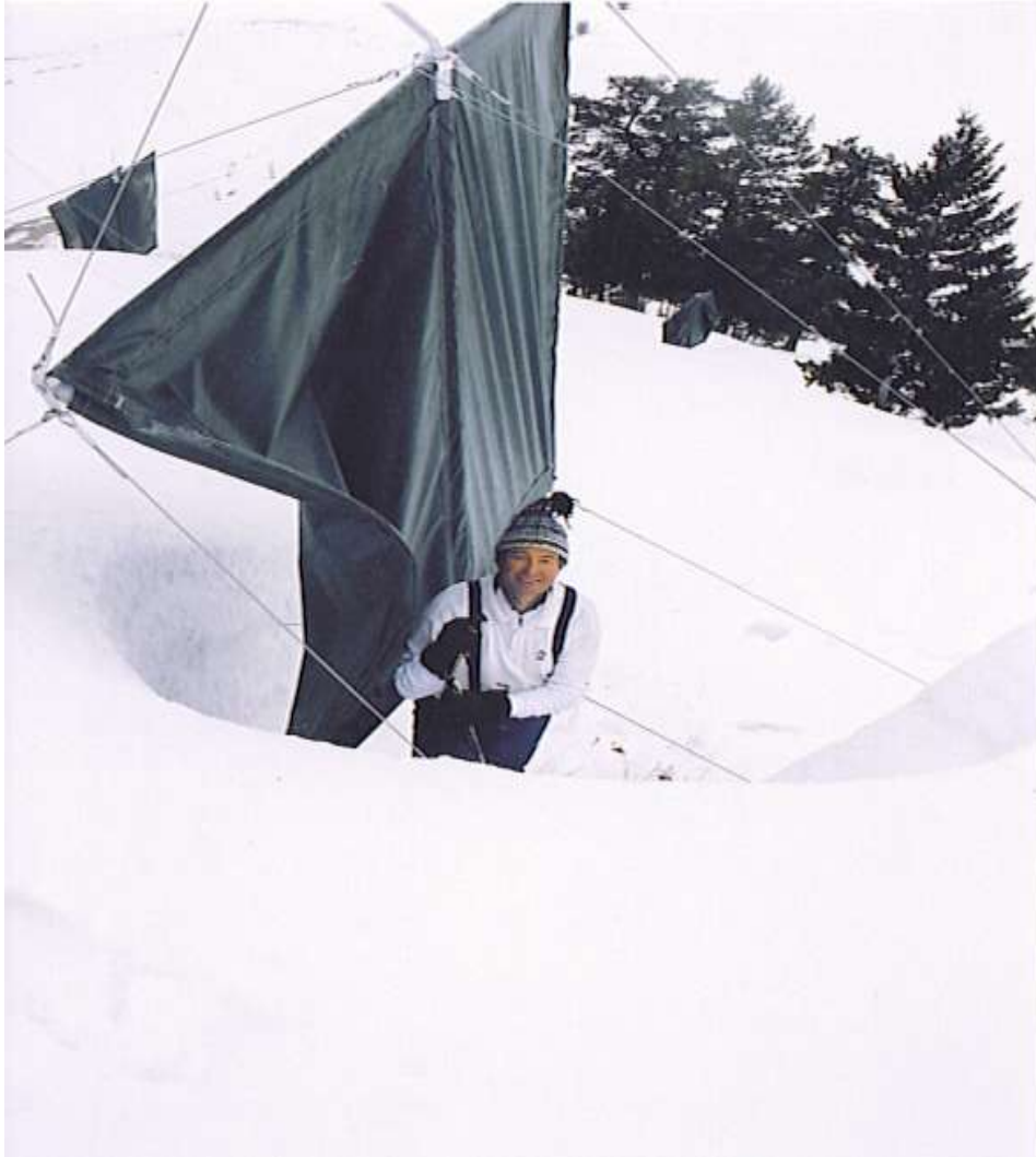
Figure 28. A snow sail in RM 151 Avalanche starting zone above US Route 189/191 in south Jackson.
