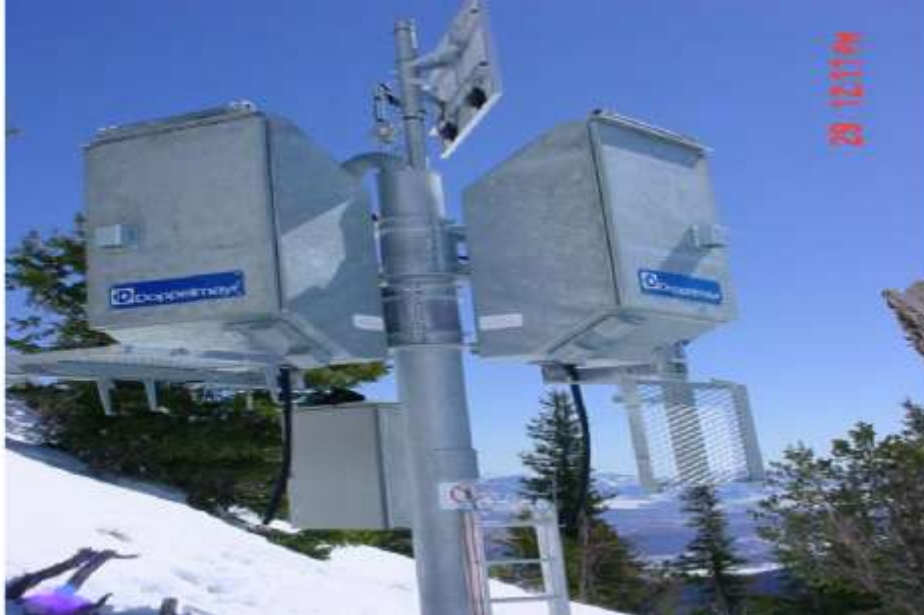
Figure 7. A remotely operable avalanche control ‘mortar’, a Doppelmayer® Avalanche Guard®, near multiple avalanche starting zones above State Route 22, on Teton Pass, Wyoming.
