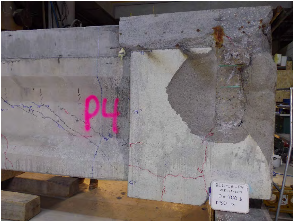
Figure B.48 Girder P4 Northside Section 1-Section 2 P=400 kips
