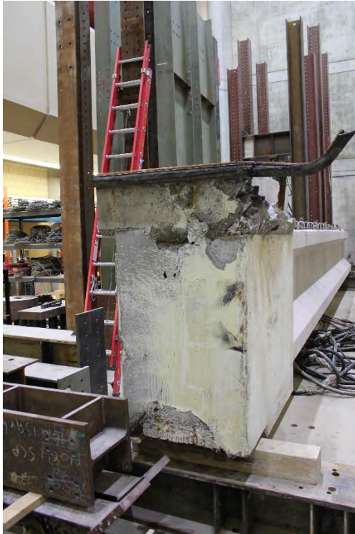
Figure B.83 Girder P26 Prior to Casting – Repair End View
