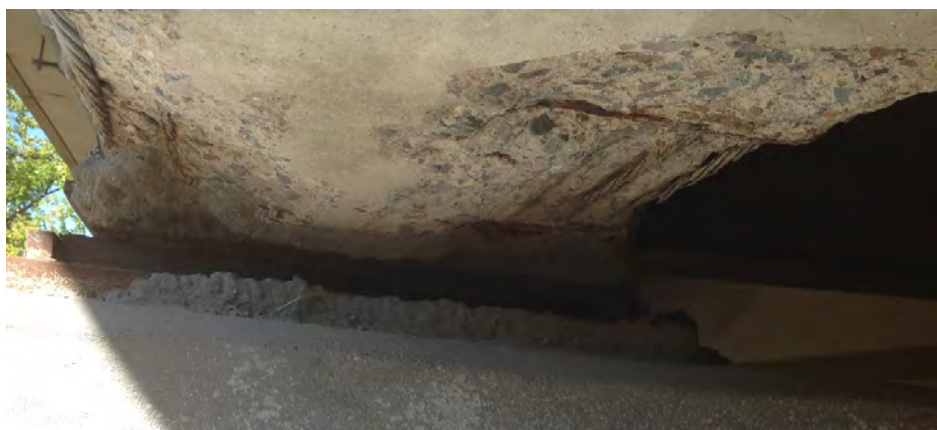
Figure A.9: Beam end at Pier 4 prior to preparation.
