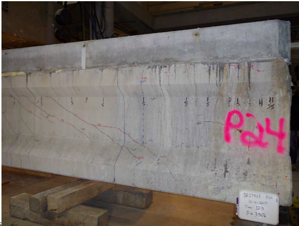
Figure B.78 Girder P24 Northside Section 1-Section 2 P=350 kips
