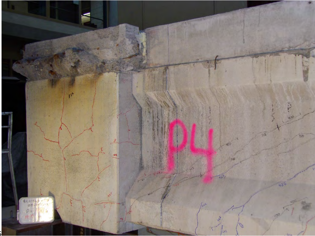
Figure B.55 Girder P4 Repair Section 1 P=450 kips
