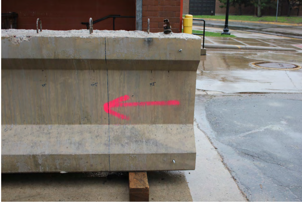
Figure B.8 Girder P2 Prior to Casting – Section 8 (Cut-End)
