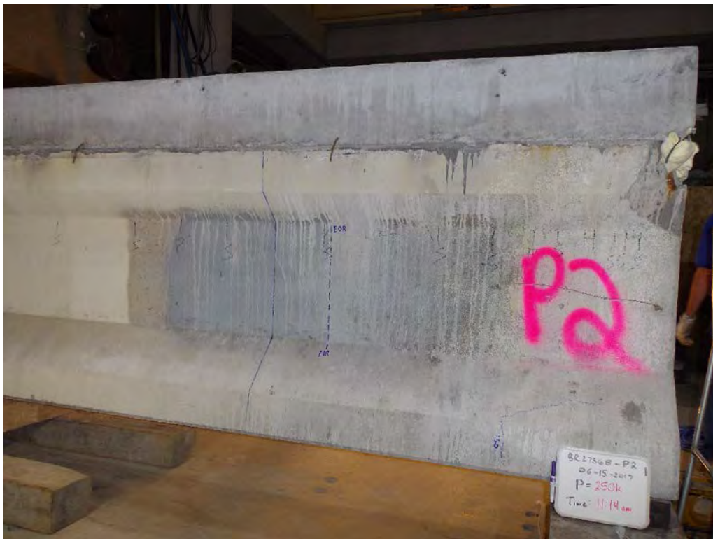
Figure B.17 Girder P2 Northside Section 1-Section 2 P=250 kips
