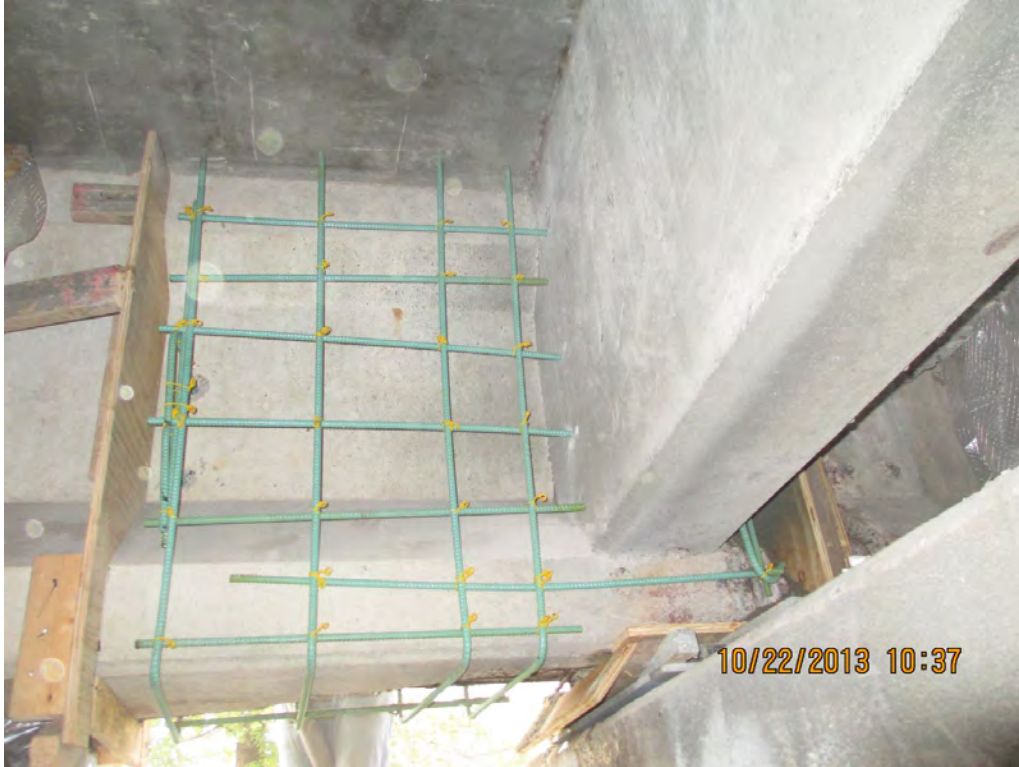
Figure 1.7 Supplemental reinforcement in place on interior side of girder at Pier 26
