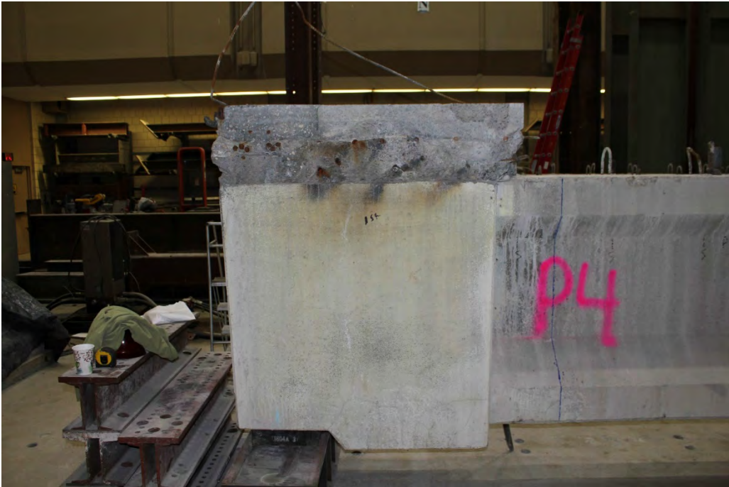
Figure B.26 Girder P4 Prior to Casting – Section 1
