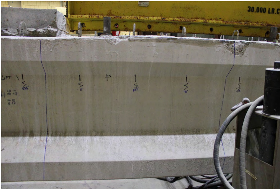
Figure B.58 Girder P24 Prior to Casting – Section 2
