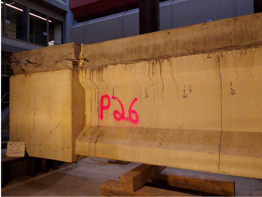
Figure B.110 Girder P26 Repair Section 1 – Section 2 P=325 kips
