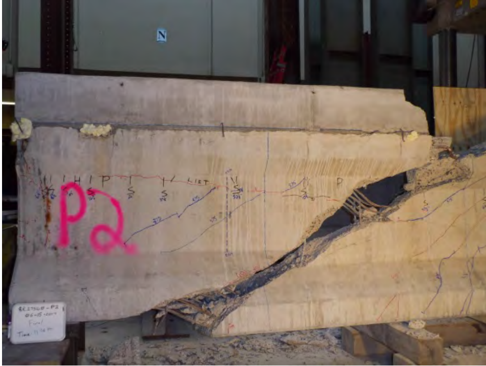
Figure 4.10 Girder P2 after failure
