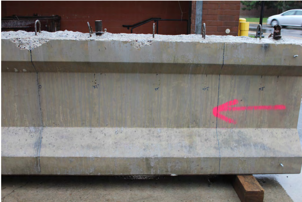
Figure B.7 Girder P2 Prior to Casting – Section 7
