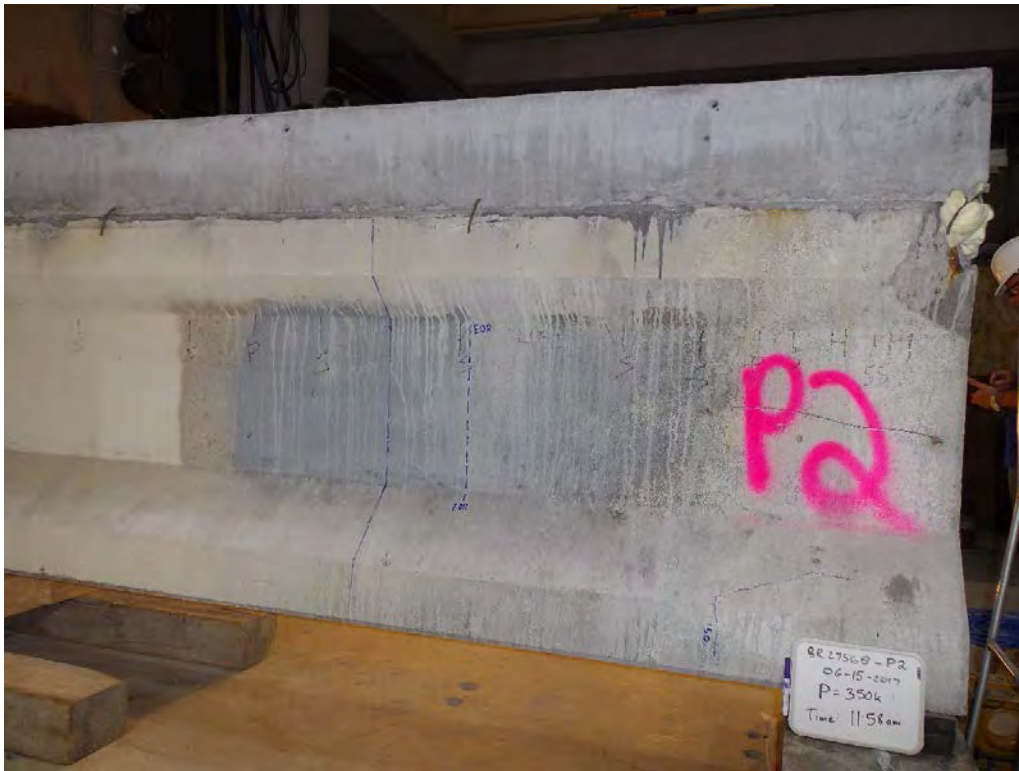
Figure B.21 Girder P2 Northside Section 1-Section 2 P=350 kips
