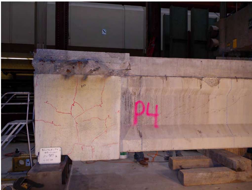
Figure B.36 Girder P4 Southside Section 1-Section 3 P=325 kips
