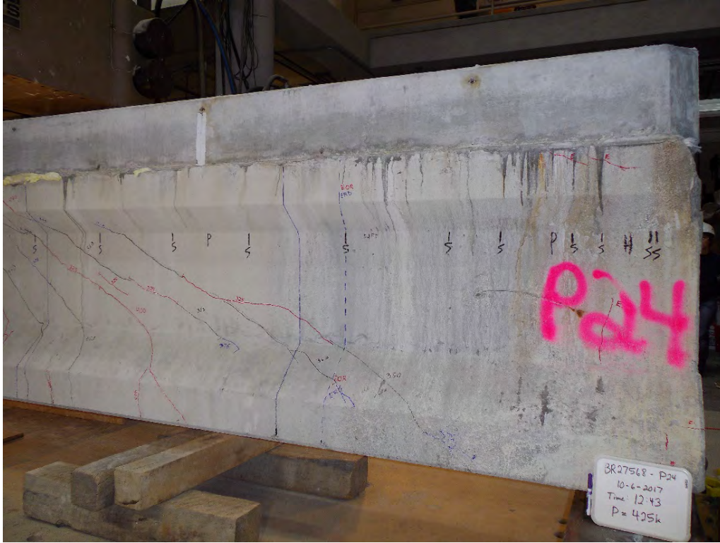
Figure B.81 Girder P24 Northside Section 1-Section 2 P=425 kips
