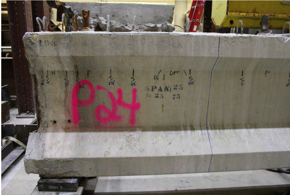
Figure B.57 Girder P24 Prior to Casting – Section 1
