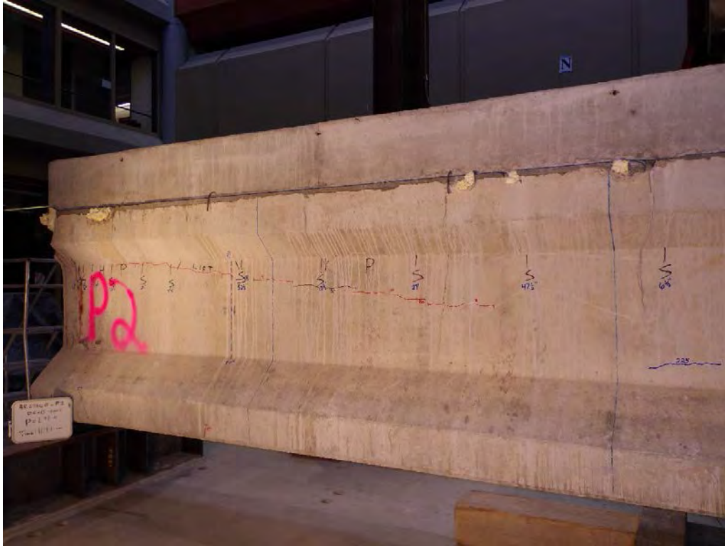
Figure B.10 Girder P2 Southside Section 1-Section 2 P=275 kips
