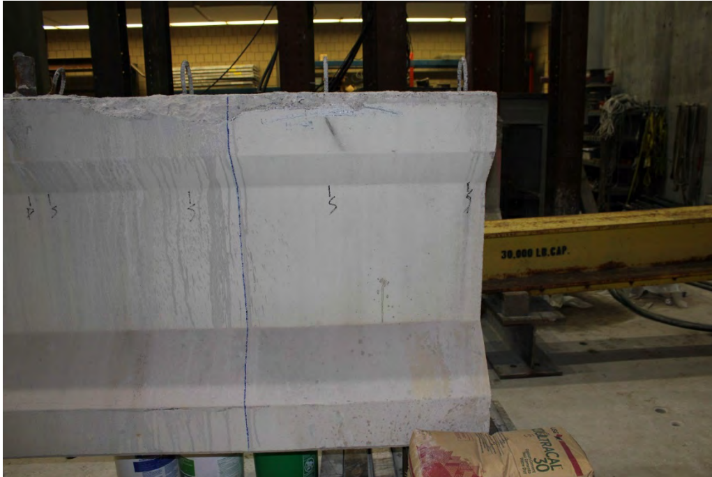
Figure B.33 Girder P4 Prior to Casting – Section 8 (Cut-End)
