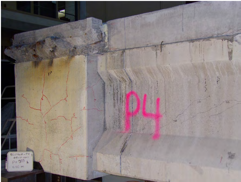
Figure B.54 Girder P4 Repair Section 1 P=325 kips
