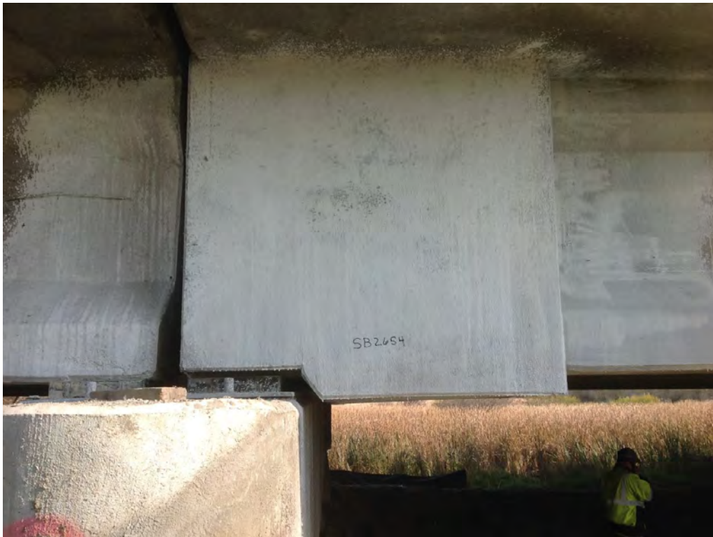
Figure 1.10 Finished repair on girder at Pier 26
