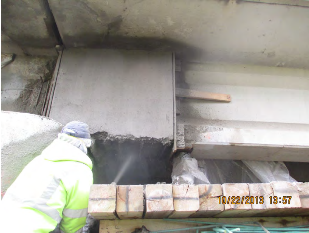
Figure 1.9 Shotcreting the bottom surface of the repair on girder at Pier 26
