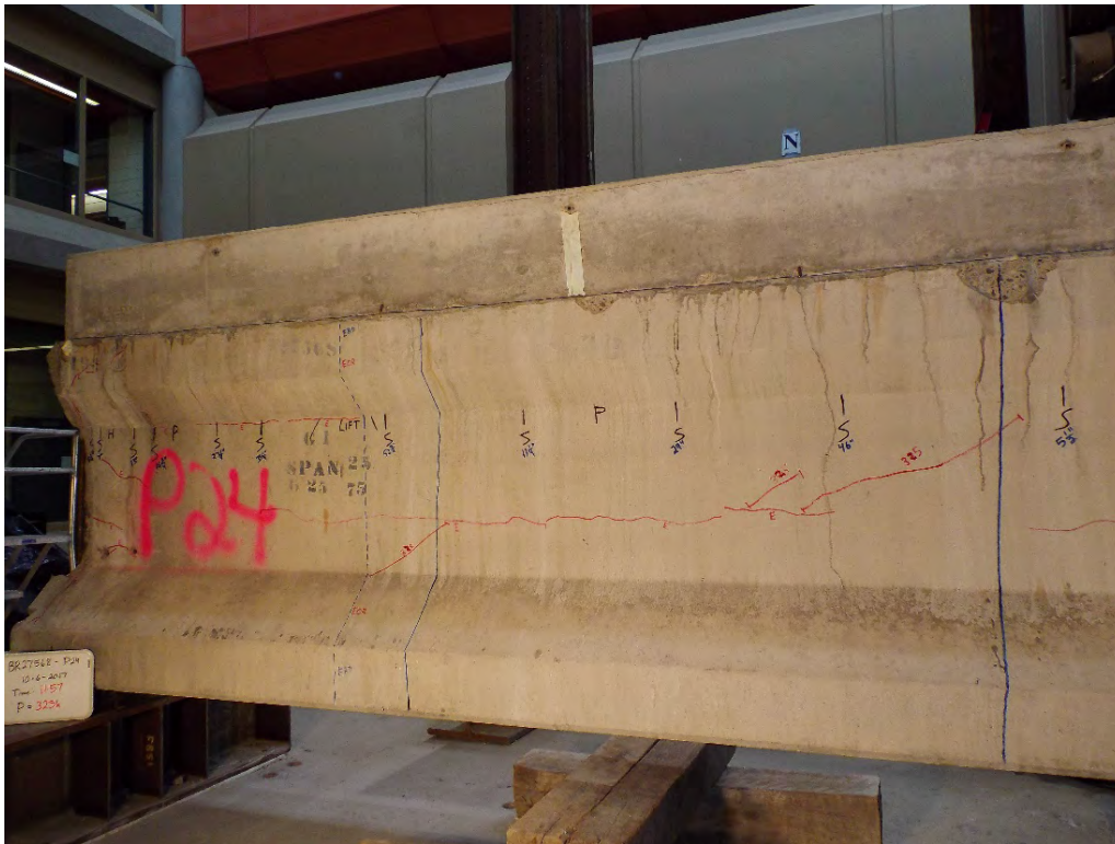
Figure B.68 Girder P24 Southside Section 1-Section 2 P=325 kips
