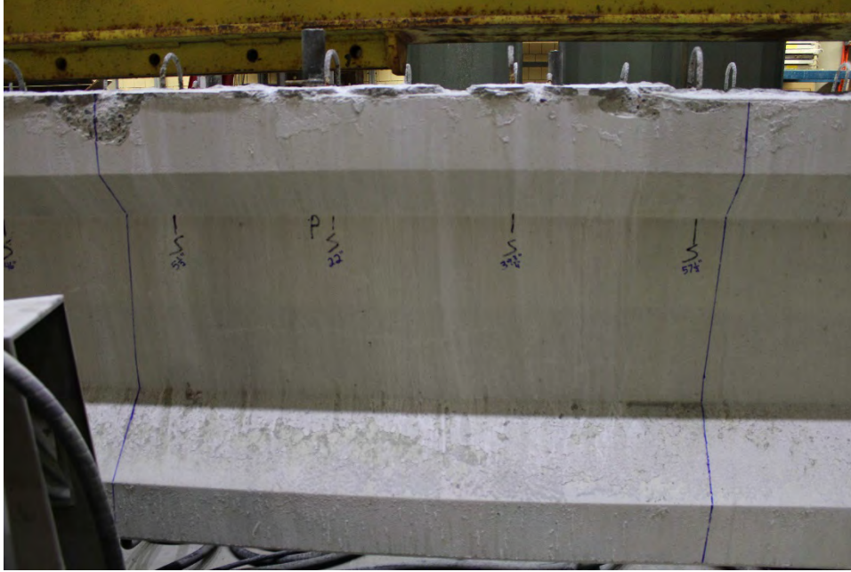
Figure B.59 Girder P24 Prior to Casting – Section 3
