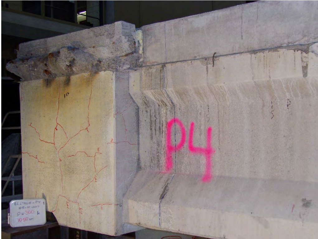
Figure B.53 Girder P4 Repair Section 1 P=300 kips
