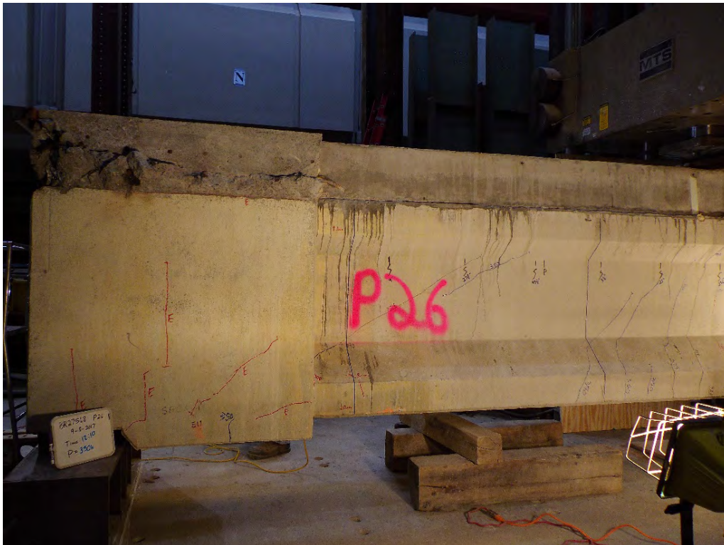
Figure B.95 Girder P26 Southside Section 1-Section 3 P=350 kips
