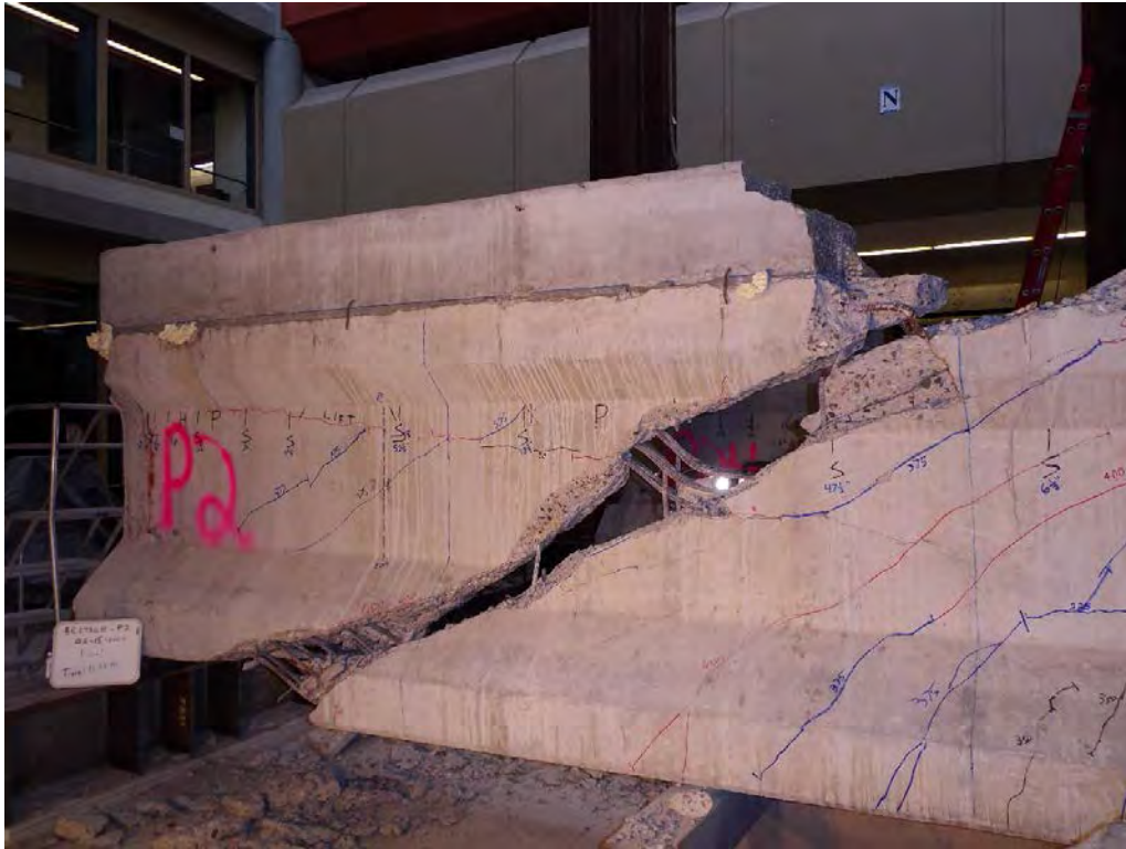
Figure B.16 Girder P2 Southside Section 1-Section 2 Failure
