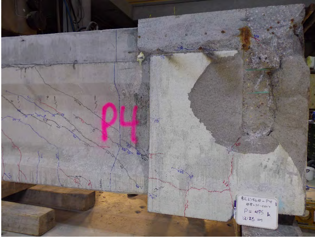
Figure B.51 Girder P4 Northside Section 1-Section 2 After Peak = 465 kips (load incorrectly labeled on white board)
