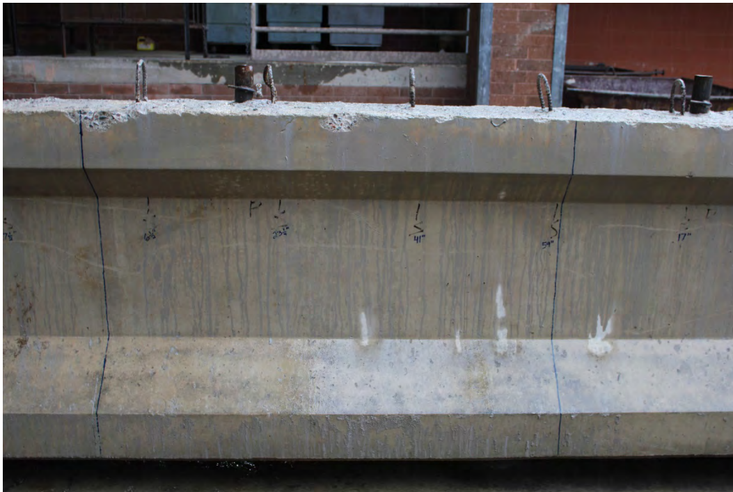
Figure B.3 Girder P2 Prior to Casting – Section 3
