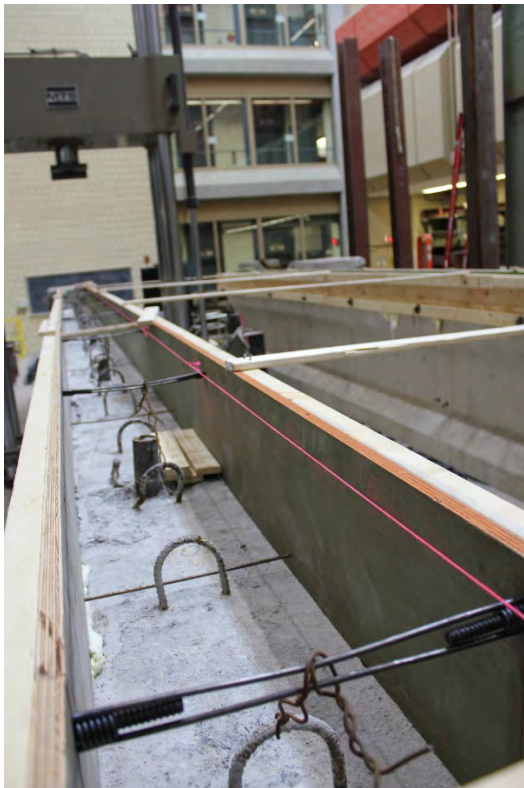
Figure 3.1 Installed formwork for the deck
