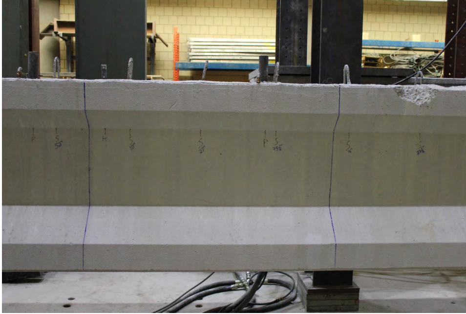
Figure B.88 Girder P26 Prior to Casting – Section 5
