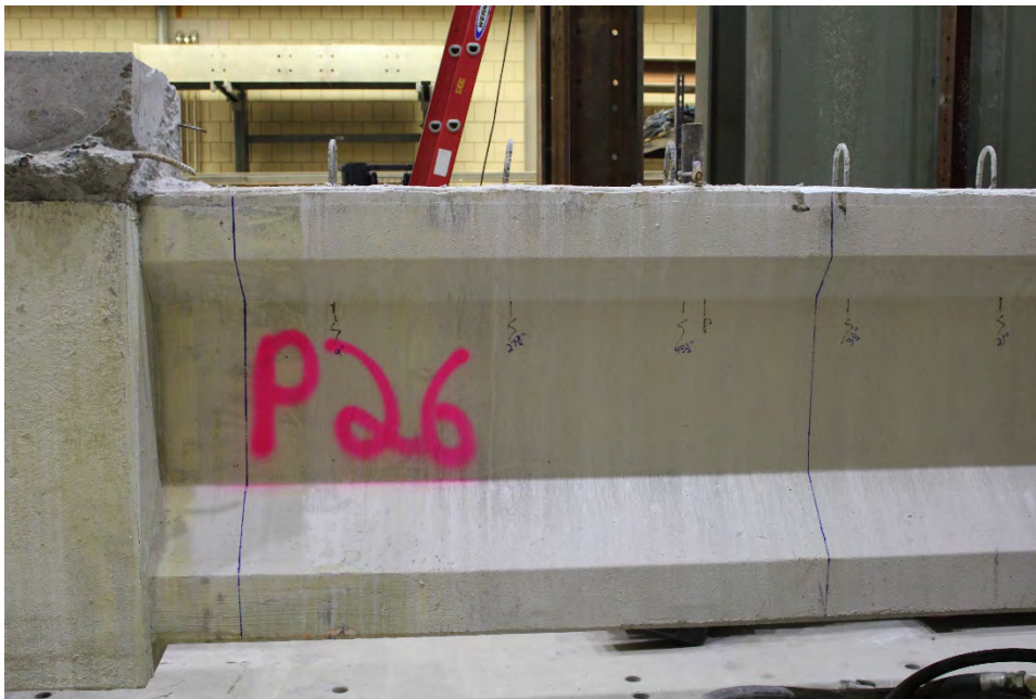
Figure B.85 Girder P26 Prior to Casting – Section 2
