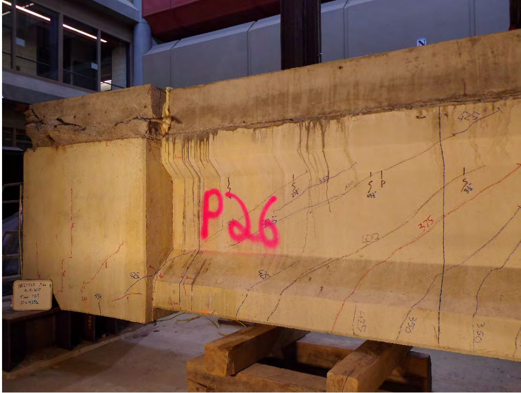
Figure B.114 Girder P26 Repair Section 1 – Section 2 P=425 kips
