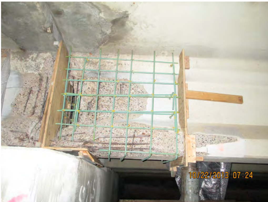
Figure 1.6 Supplemental reinforcement in place on external side of girder at Pier 26
