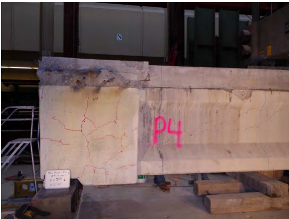
Figure 4.3 Girder P4 web shear cracking P= 325 k
