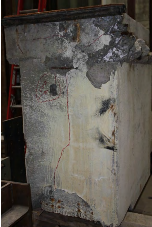
Figure 2.11 Girder P26 end condition
