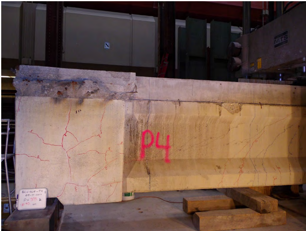
Figure B.38 Girder P4 Southside Section 1-Section 3 P=375 kips
