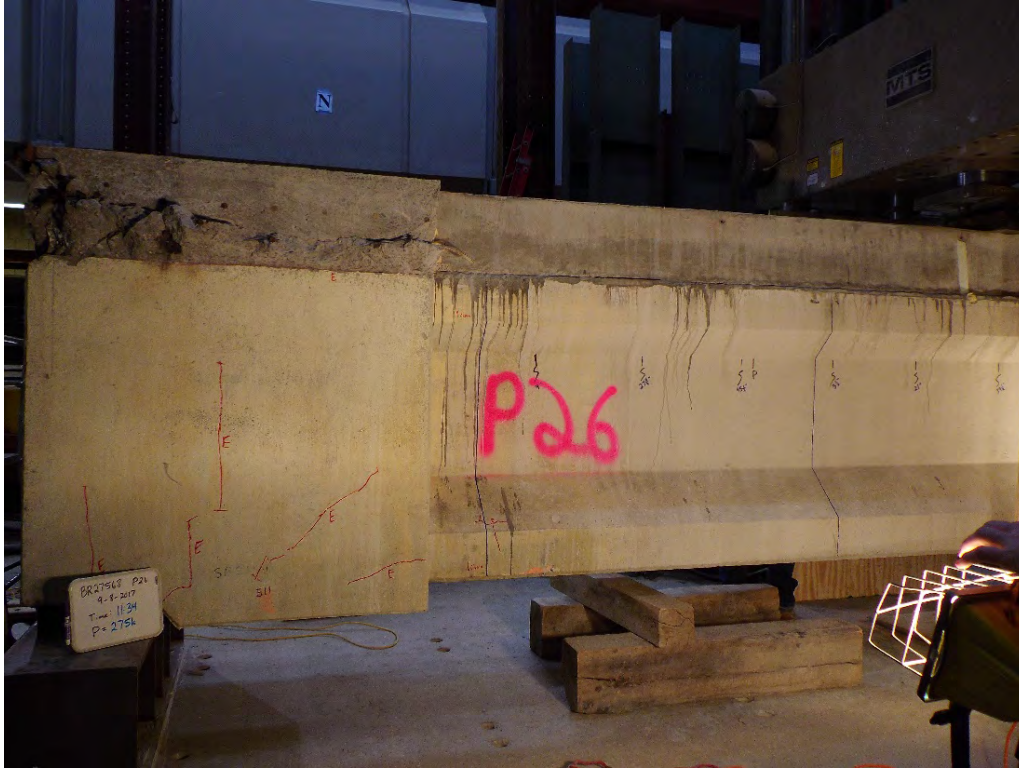
Figure B.92 Girder P26 Southside Section 1-Section 3 P=275 kips
