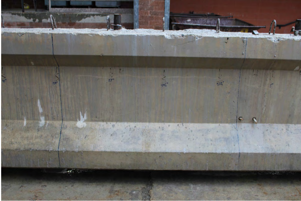
Figure B.4 Girder P2 Prior to Casting – Section 4
