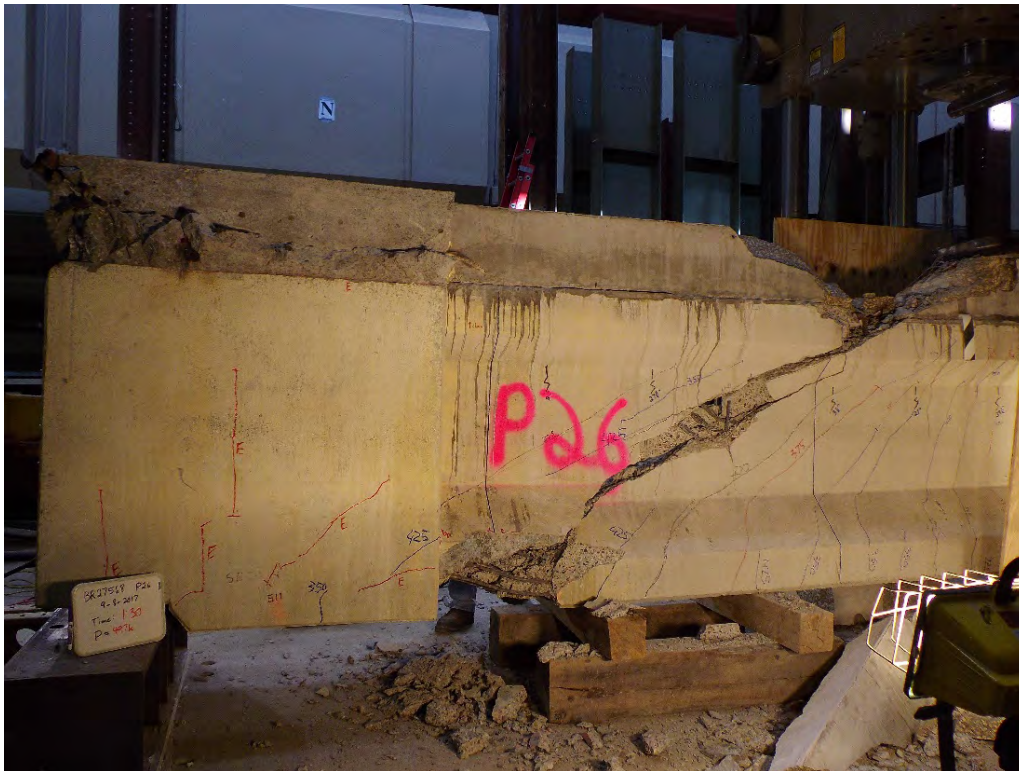
Figure B.99 Girder P26 Southside Section 1-Section 3 Failure
