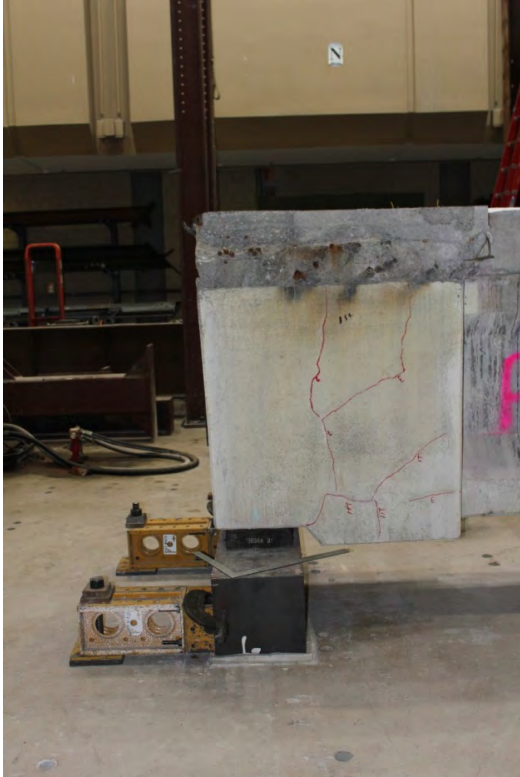
Figure 2.7 Girder P4 as-received cracking on the exterior side at the repaired end
