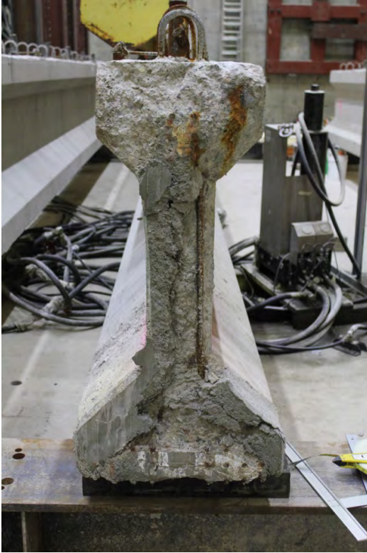
Figure 2.5 Corrosion of transverse reinforcement at the end of interest on Girder P24
