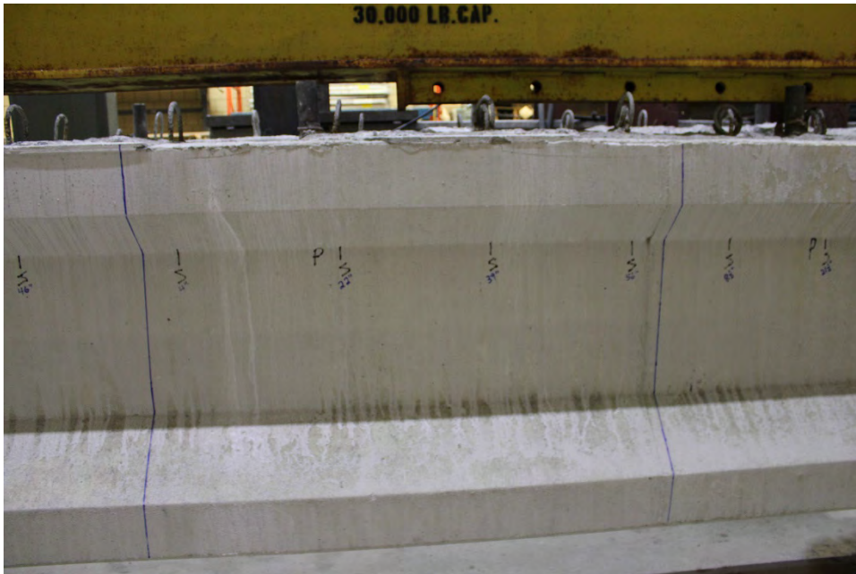
Figure B.62 Girder P24 Prior to Casting – Section 6
