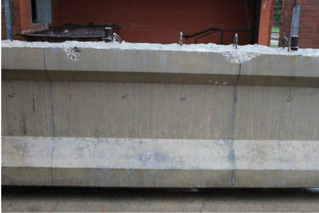
Figure B.6 Girder P2 Prior to Casting – Section 6
