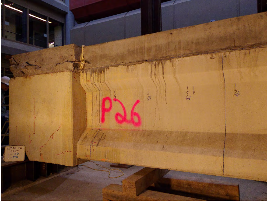
Figure B.108 Girder P26 Repair Section 1 – Section 2 P=275 kips
