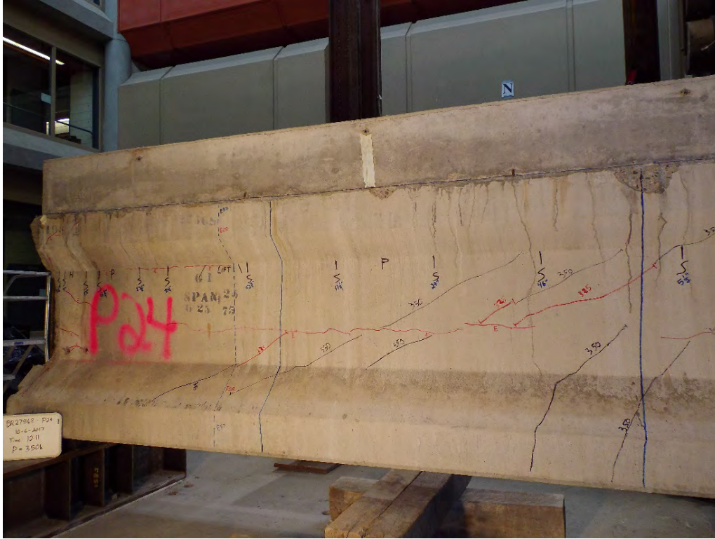
Figure B.69 Girder P24 Southside Section 1-Section 2 P=350 kips
