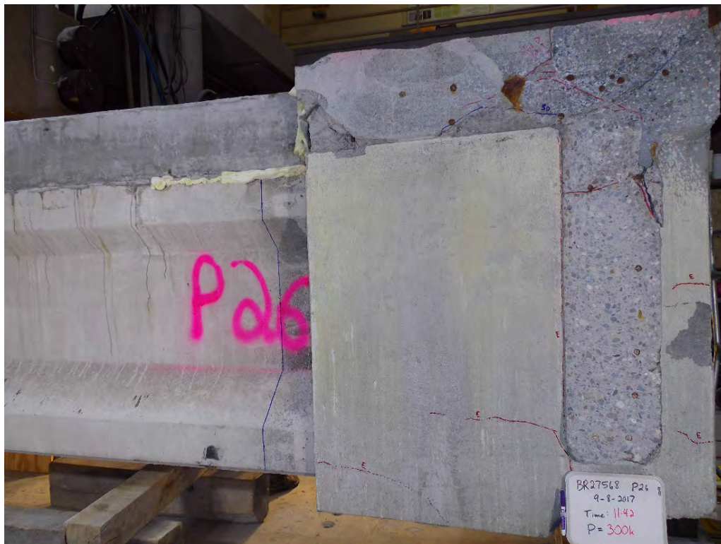
Figure B.101 Girder P26 Northside Section 1-Section 2 P=300 kips
