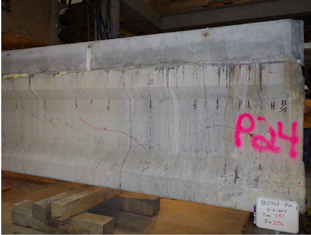
Figure B.77 Girder P24 Northside Section 1-Section 2 P=325 kips
