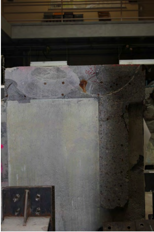
Figure 2.9 Girder P26 on diaphragm side
