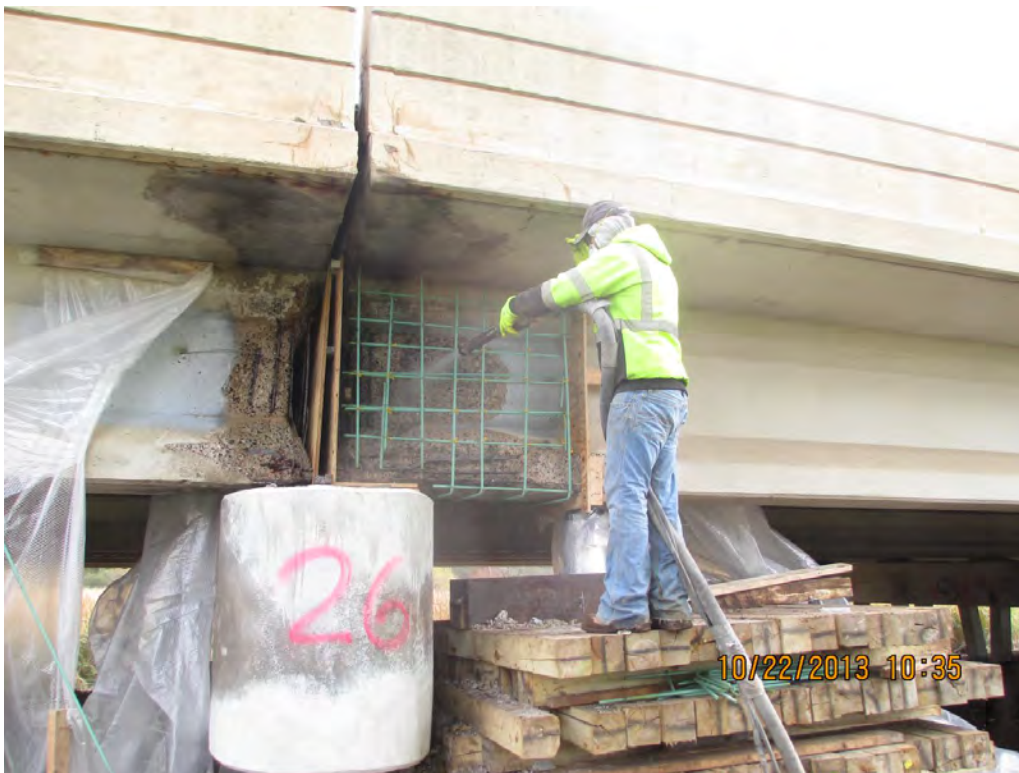
Figure 1.8 Shotcreting of repair on girder at Pier 26
