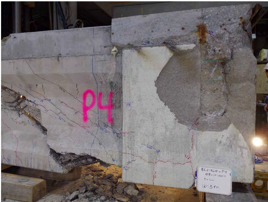
Figure B.52 Girder P4 Northside Section 1-Section 2 Failure
