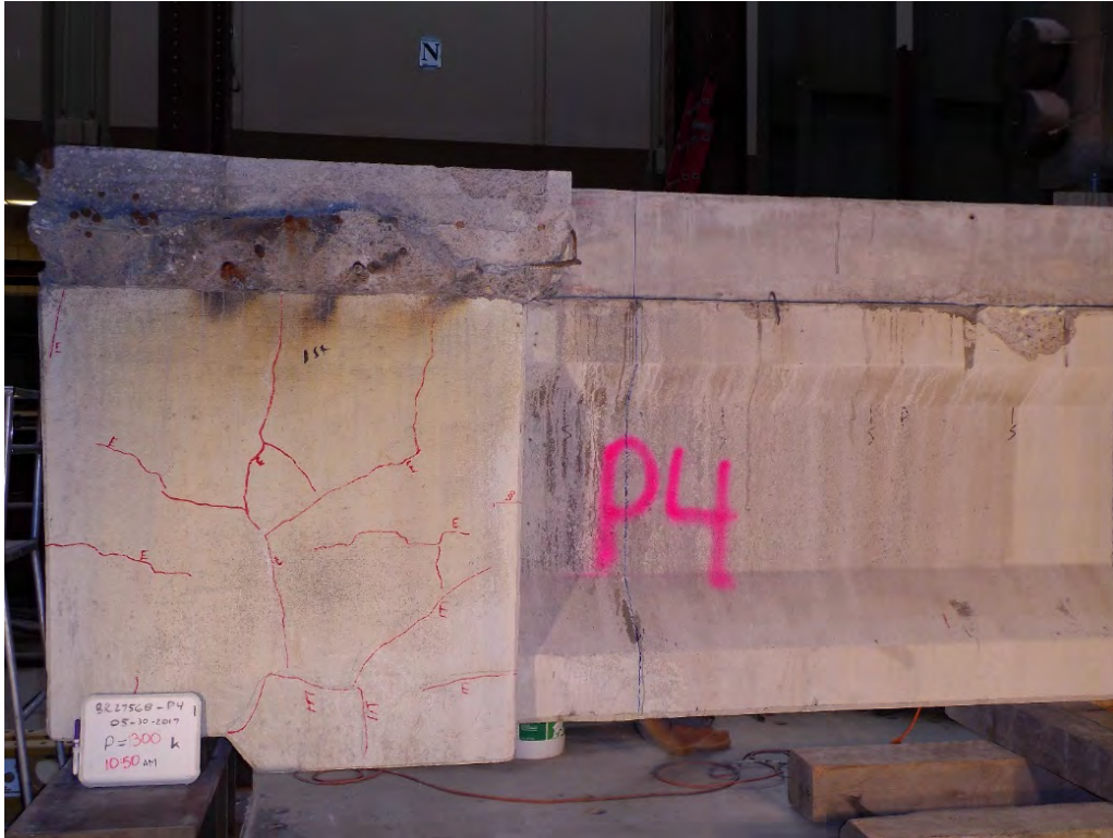
Figure B.35 Girder P4 Southside Section 1-Section 3 P=300 kips
