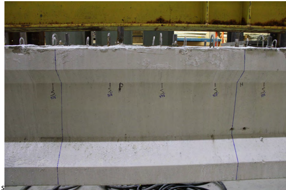
Figure B.60 Girder P24 Prior to Casting – Section 4
