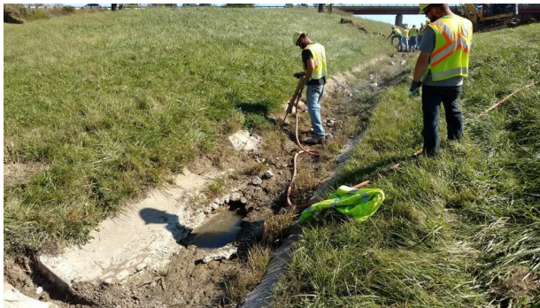
Figure 1. Observation of Current Ashland County Process. Left: Deteriorated concrete demolition. Right: New concrete placed in alternating segments.
