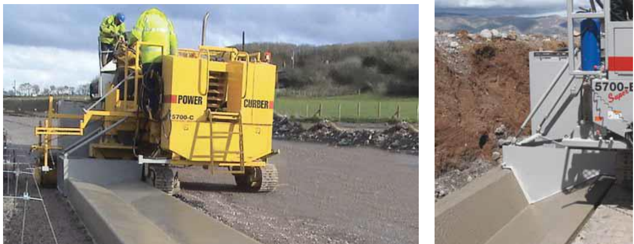
Figure 2. Curb Machine PWC5700-C V-Ditch Applications (Source: PowerCurbers Inc.)
