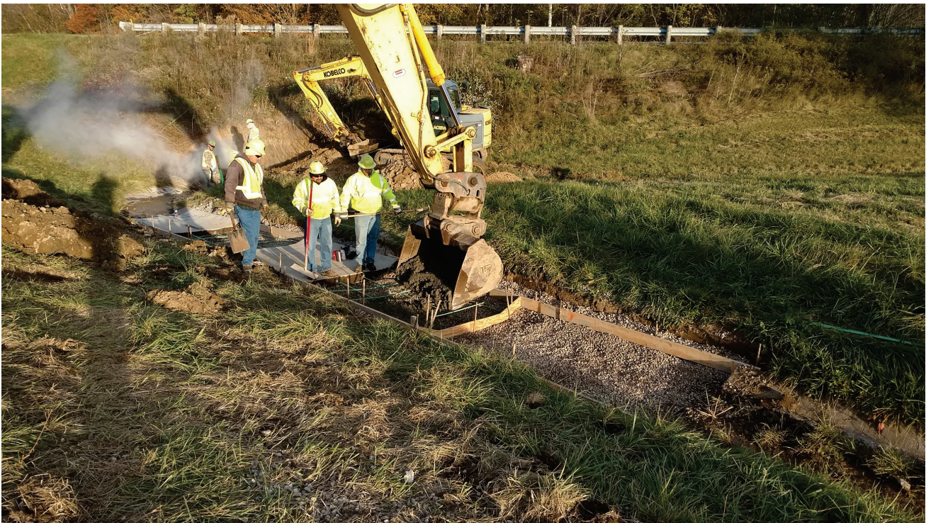
Placement of concrete was done by use of a backhoe which in this location worked fine. Workers in background did not have adequate safety PPE (Personnel Protective Equipment.)
