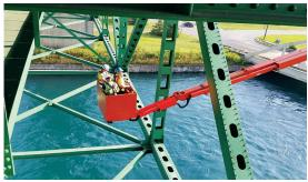
Large, complex bridges require inspection methods such as the use of underbridge inspection units (UBIUs) that reach from above deck to below.
